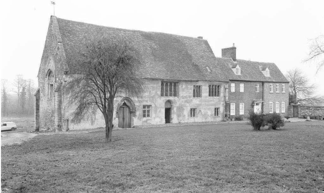
Fig 16: Bushmead Priory, Bedfordshire, c 1969, after the demolition of much of the house to reduce it to a more manageable size. © Crown Copyright
