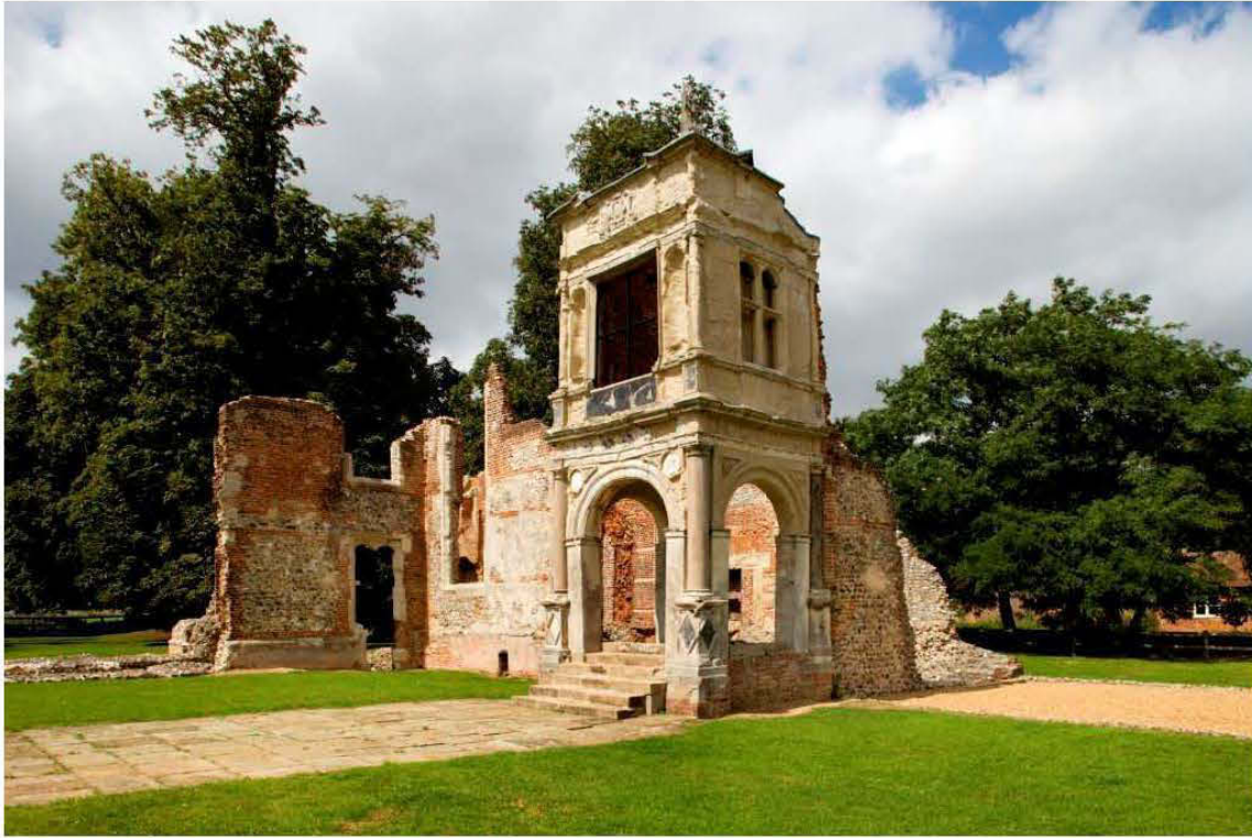
Fig 21: Old Gorhambury after treatment, photographed in 2009. © English Heritage
