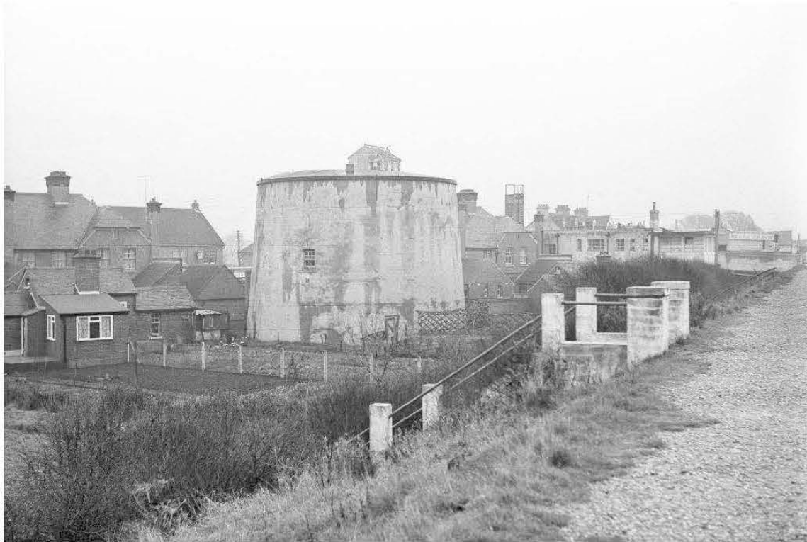
Fig 13: Dymchurch Martello Tower, Kent, in 1955. Reproduced by permission of English Heritage
