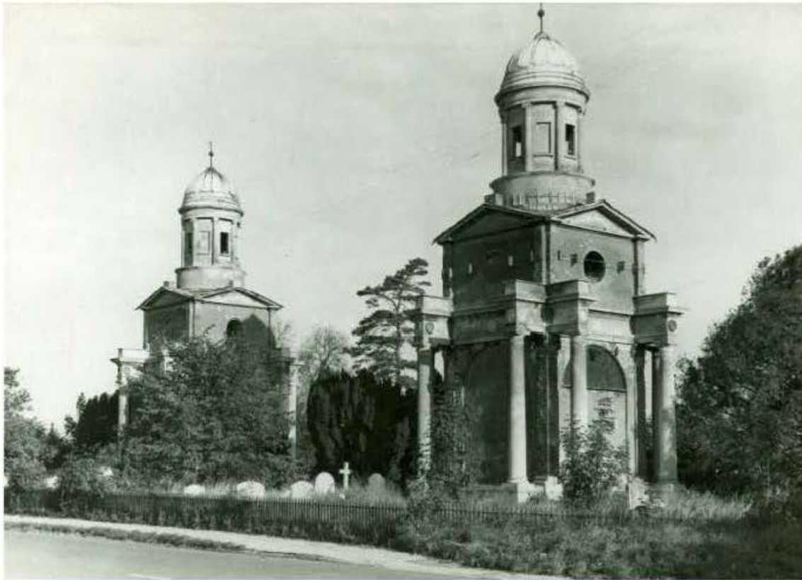
Fig 6: Mistley Towers, Essex, c. 1954, before repairs; note the bands tied round the nearer of the two towers in an attempt to stabilise it. Reproduced by permission of English Heritage
