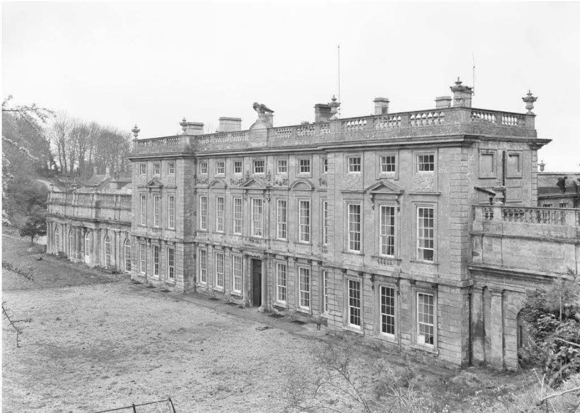
Fig 10: The east front of Dyrham Park, Gloucestershire in 1957, before repair by the Ministry. Reproduced by permission of English Heritage
