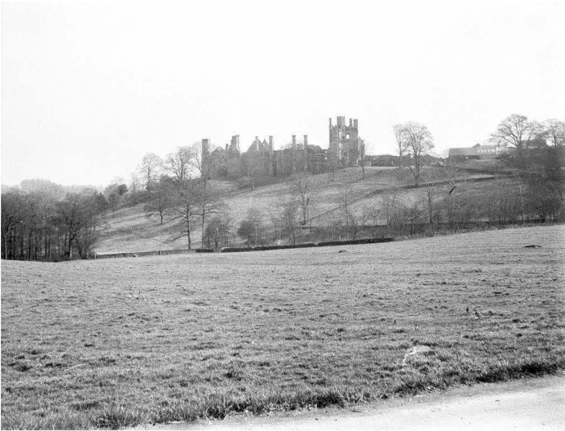
Fig 11: Wingfield Manor, Derbyshire in 1961. Reproduced by permission of English Heritage
