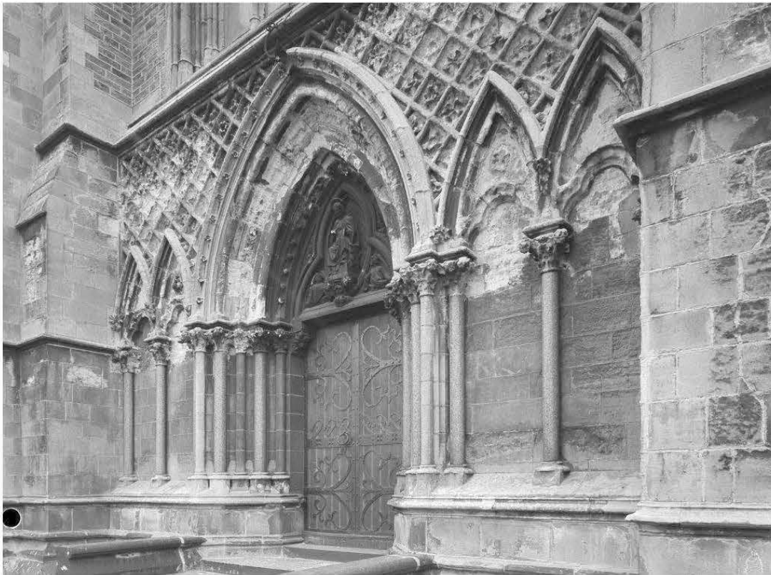
Fig 7: The west front of All Souls, Haley Hill showing the decay of the stonework. Reproduced by permission of English Heritage
