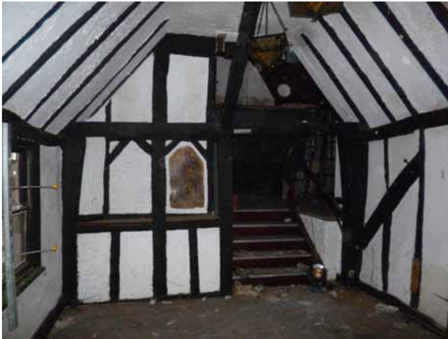
Figure 6: West wing, truss 1, photograph taken from the south (Robert Howard)
