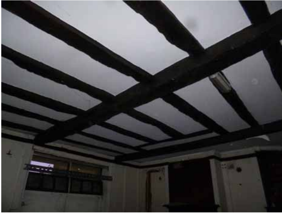
Figure 7: East wing, ground-floor ceiling, photograph taken from the north-east (Robert Howard)
