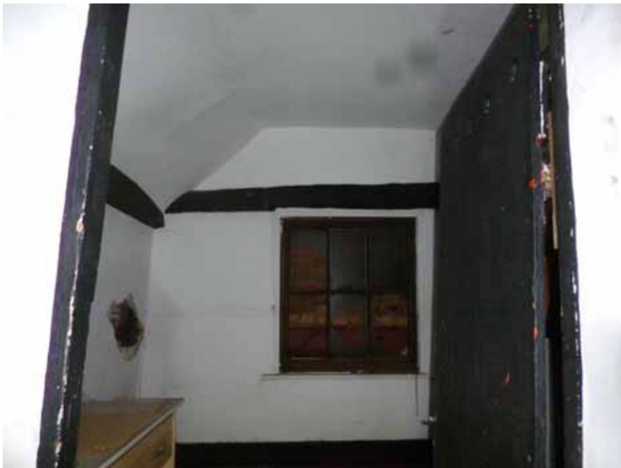
Figure 8: East wing, truss 1, photograph taken from the south (Robert Howard)
