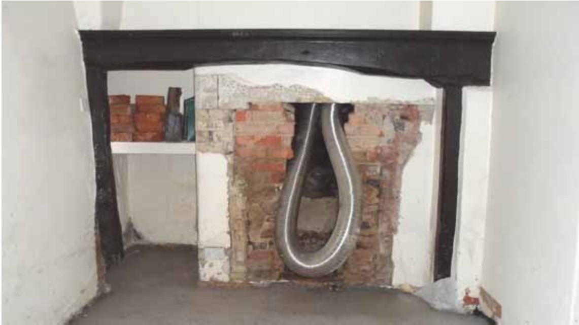
Figure 11: West wing, ground-floor bresummer and posts, photograph taken from the south (Alison Arnold)
