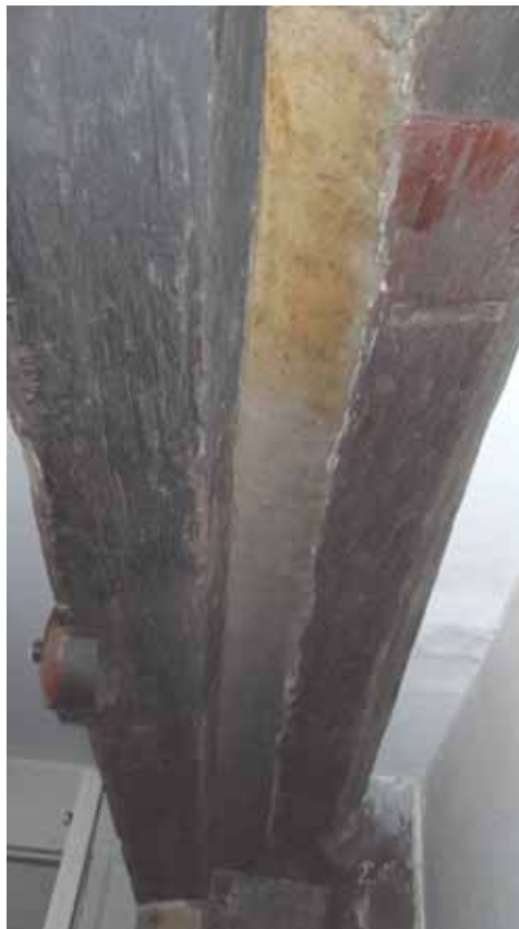
Figure 14: Chapel, double lintel over ground-floor fireplace, with inner lintel chamfered and stopped towards stack, photograph taken from the south (Alison Arnold)
