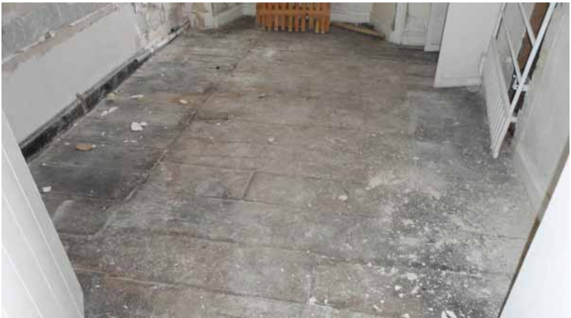
Figure 10: First-floor floorboards, photograph taken from the east (Alison Arnold)
