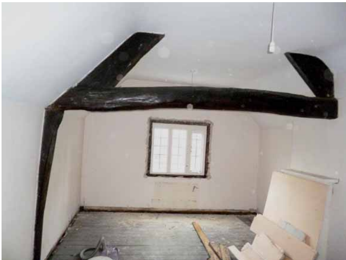
Figure 12: South-west wing, truss, photograph taken from the north (Alison Arnold)
