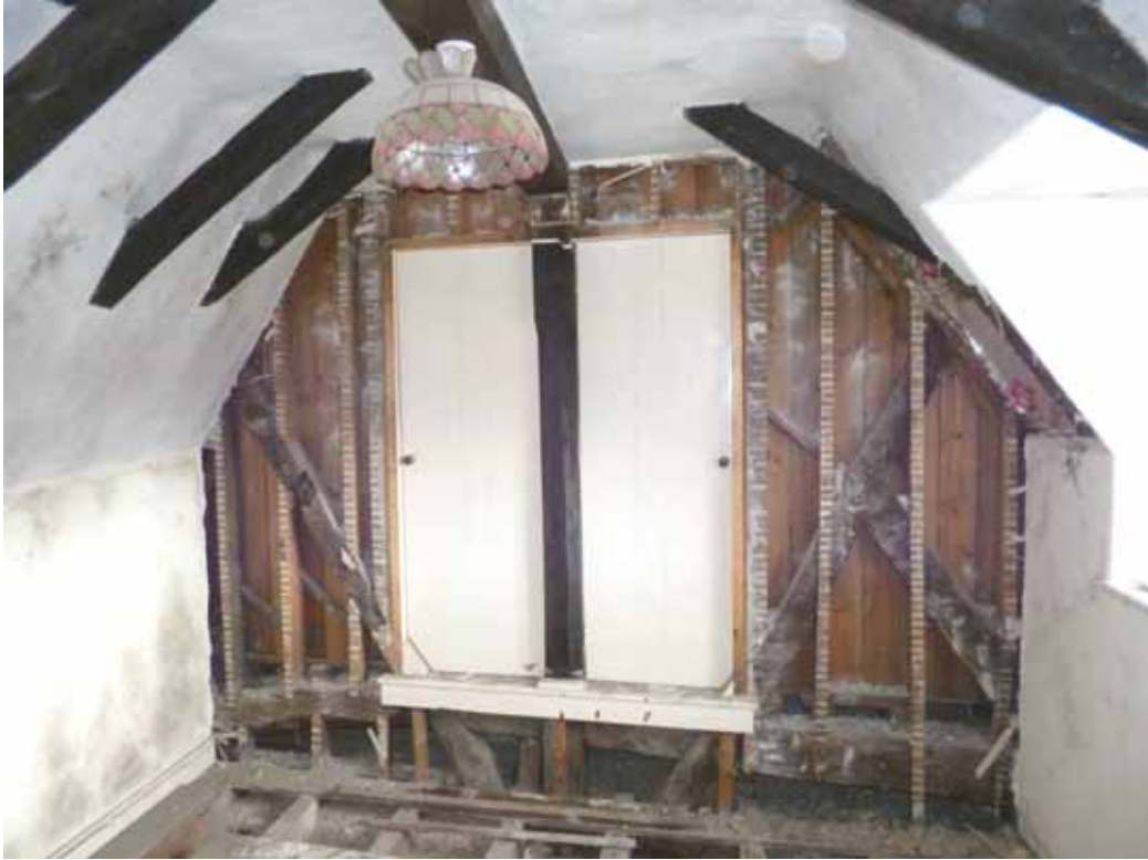
Figure 5: Hall house, roof, truss 1, photograph taken from the west (Alison Arnold)
