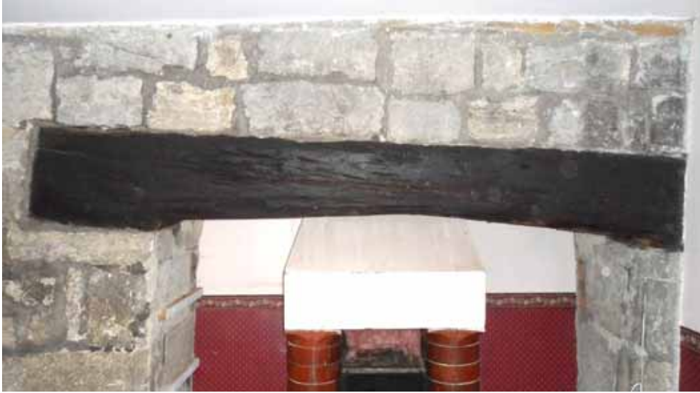
Figure 15: First-floor bedroom, fireplace lintel, photograph taken from the east (Alison Arnold)
