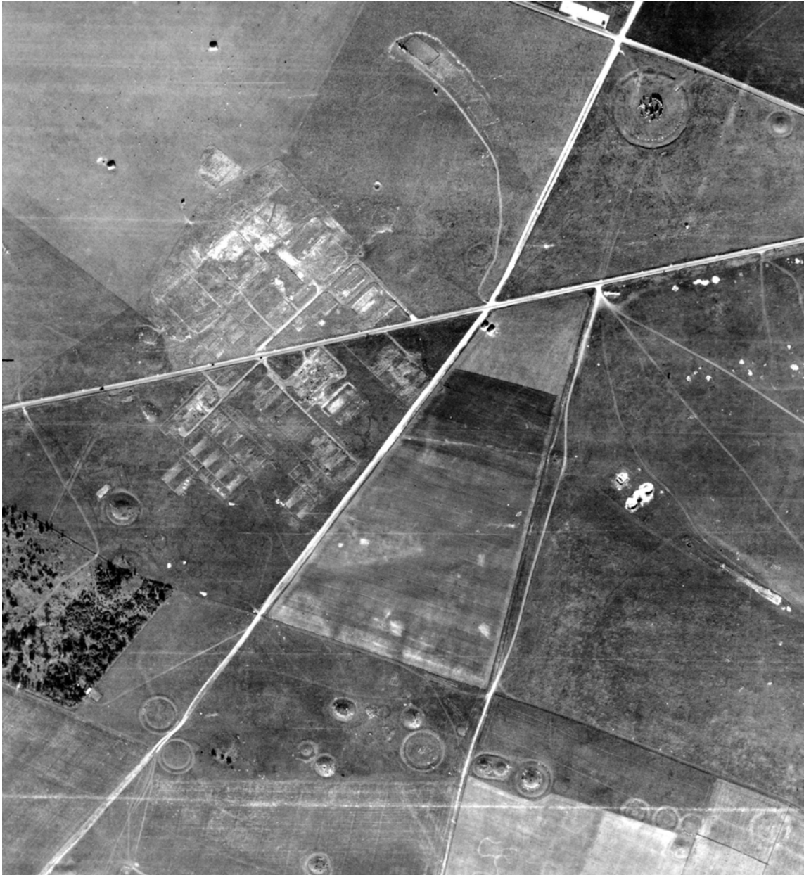
Figure 25: Extract from RAF vertical taken in October 1945, indicating that the floors of some of the buildings at least were still in situ beneath the turf. Presumably the same applied to the surfaces of the roads within the Camp. Other notable features include what looks like a succession of sheep pens between the Aerodrome site and Stonehenge, approached by a curving track heading north from the A303. Extreme top, right of centre, the surface of the Stonehenge Car Park is highly visible, and empty. At the bottom of the photograph, the Normanton Down barrow group stretches from left to right across the frame, in the process changing from earthworks to more ghost-like soil- and cropmarks. English Heritage Archive RAF Photography RAF 106G/UK/915/3203 11 October 1945.
