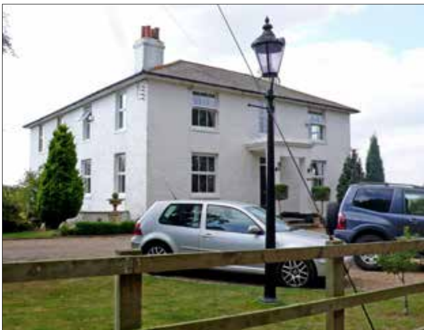
Figure 10 The former neo-classical villa-style farmhouse of Coombe Farm, now called Coombe House (P5733074)
