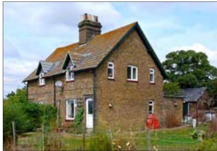
Figure 15 Nos 4-6, The Street: a surviving pair of late-19 th century farmworkers' houses in St Mary Hoo. (P5733079)
