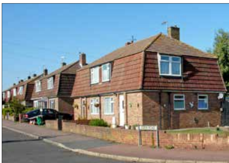
Figure 14 Non-traditional (Cornish Unit Type I) housing along Eden Road. (P5733063)
