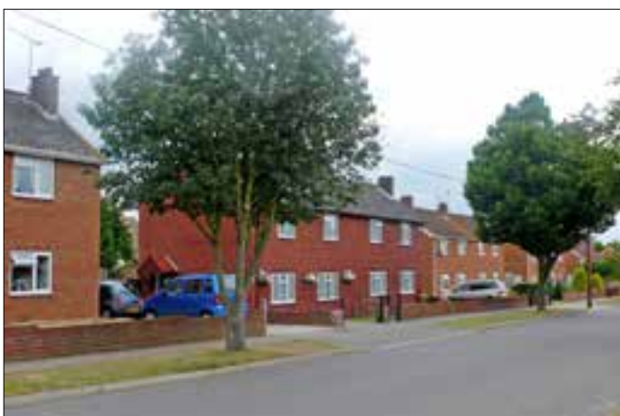
Figure 23 The Swingate Estate still preserves much of the character of a post-war local authority planned estate, despite the early-21st-century brick re-cladding of many of the non-traditional (Airey-type) houses. (P5733100)
