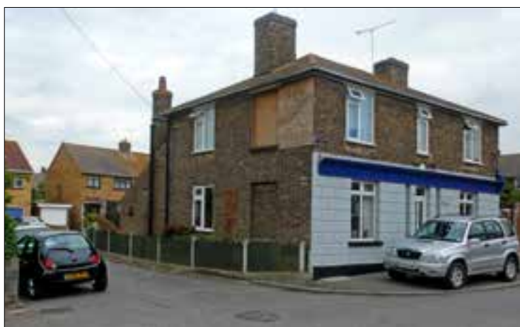
Figure 20 The former Compasses public house on Marsh Lane, dated 'SR 1849': an uncommon survivor from the Cliffe's pre-industrialised era. (P5733097)
