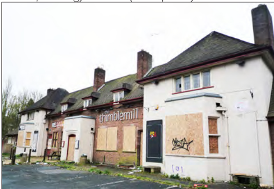
1.2 The Thimblemill pub, Smethwick, Birmingham, built in 1928 to designs by T. Spencer Wood of Wood, Kendrick and Edwin F. Reynolds. The pub was closed and demolished in 2014, to be replaced with a care home. (© Historic England, Emily Cole)
