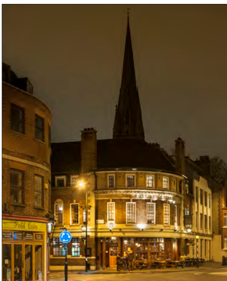
1.6 A night-time view of the Rose and Crown, Stoke Newington, London. This pub, built in 1930-32 for Truman’s brewery, is one of the 37 buildings considered in detail as part of this project. (© Historic England, Derek Kendall, DPI52310)
