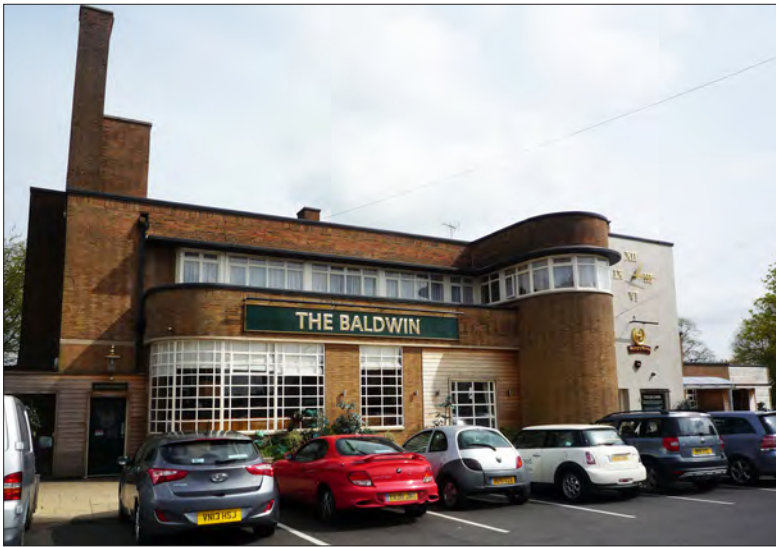
11.29 The Baldwin, Hall Green, Birmingham, is one of the many inter-war pubs that have now been converted into carveries or family-friendly pub/restaurants. The pub was built in 1937 by Mitchells & Butlers to designs by the local firm Bateman's. It is now part of the Hungry Horse chain, owned by Greene King brewery. (© Historic England, Emily Cole)
