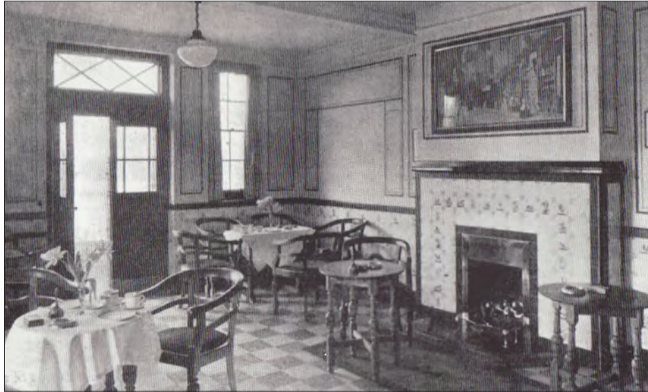
3.8 The elegant interior of the tea room at the Rose and Crown , Upperby, Carlisle, built in 1930 to designs by Harry Redfern. The pub was demolished in 2013; to date, it is the only one of Carlisle's 15 'model' inter-war pubs to have been lost. (Author's collection)
