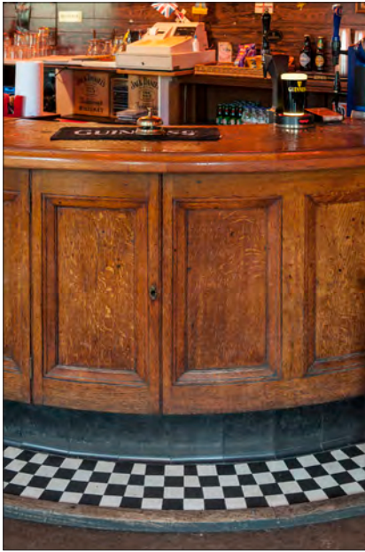
5.48 The counter in the saloon bar of the Palm Tree, Mile End, London (c. 1929), with its chequered tiled border. Such borders helped to protect floors and counters from damage by ash and discarded cigarette ends, and also from floor cleaning. (© Historic England, Derek Kendall, DPI52214)
