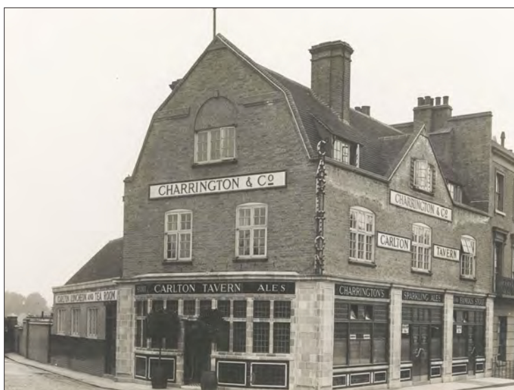
5.29 A photograph of 1924 showing the Carlton Tavern, Maida Vale, London, a Charrington's pub of 1920-21. The pub's rear block, on the left of the image, has tilework proclaiming its function as the 'Carlton Luncheon and Tea Room'. (Image courtesy of the National Brewery Centre, Burton on Trent)
