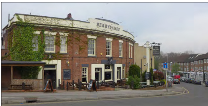
11.15 Inter-war pubs were very often plain in their external design, as here at the Berrylands Hotel, Surbiton, London, a pub of c. 1934, built for Hodgson's Kingston Brewery and designed by Joseph Hill. This plainness was a specific aim at the time, intended to differentiate pubs from their 'uncouth', often elaborate Victorian and Edwardian predecessors, but came to be viewed with criticism by those who felt pubs should 'stand out' in their settings. (© Historic England, Emily Cole)
