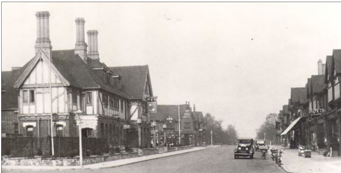
11.28 Many inter-war pubs were designed to be sensitive to the character and style of the surrounding buildings, as here with the Daylight Inn, Petts Wood, London (1935), seen in a photograph taken in 1936. The suburb of Petts Wood was built from the 1920s, mainly in the Neo-Tudor style. (Courtesy of Bromley Local Studies and Archives: C/OUDC/FIG213/3)
