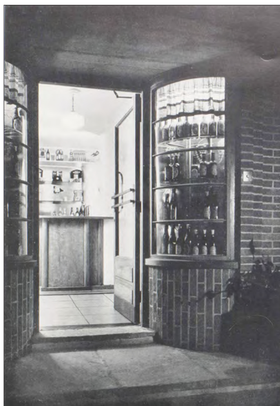
5.43 The display windows at the Nag's Head, Bishops Stortford, Hertfordshire (1936, by E. B. Musman; listed grade II), in a photograph published in the Architectural Review in 1936. The doorway led into the off sales compartment. It is now the main entrance to the pub, which has been altered in its planning.
