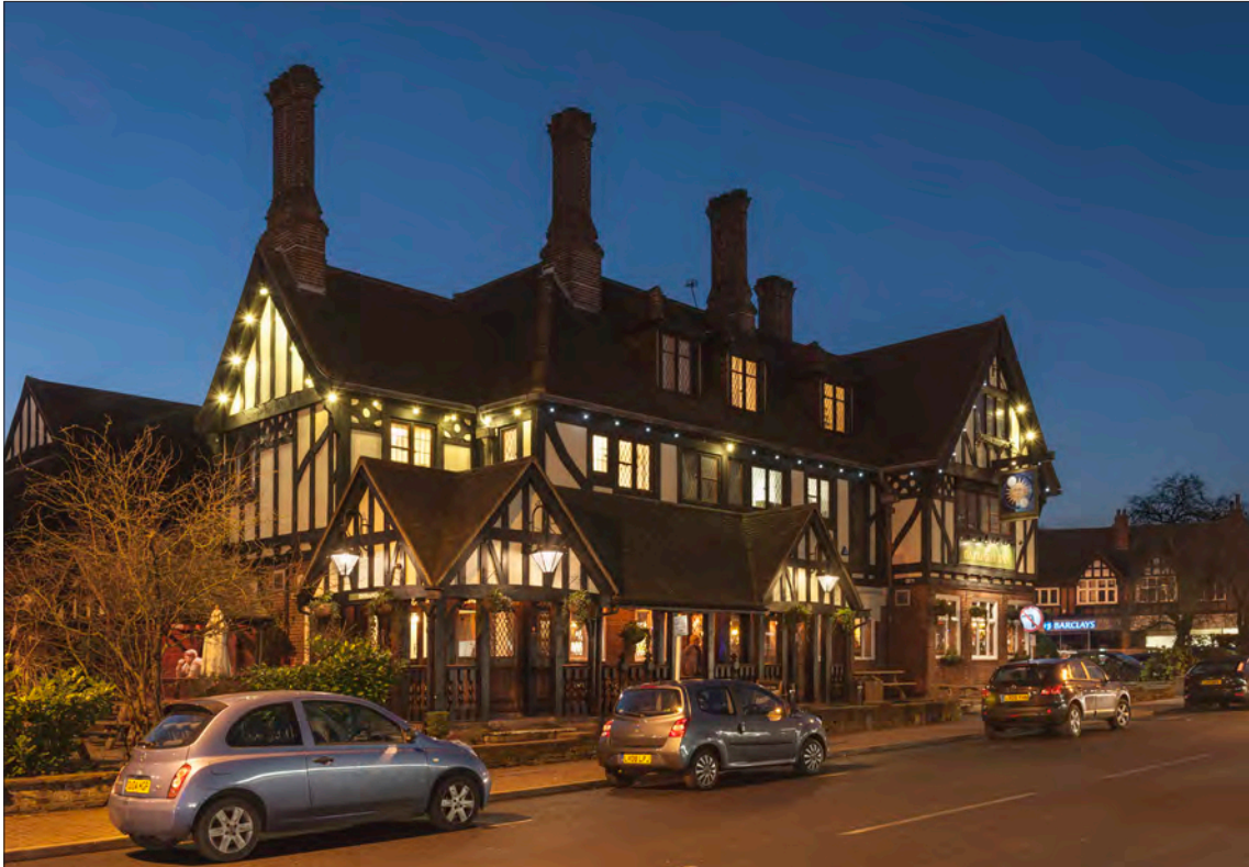
2.1 An example of an improved pub: the Daylight Inn, Petts Wood, London, built in 1935 and designed by Sidney C. Clark of Charrington's. (© Historic England, Derek Kendall, DPI70048)
