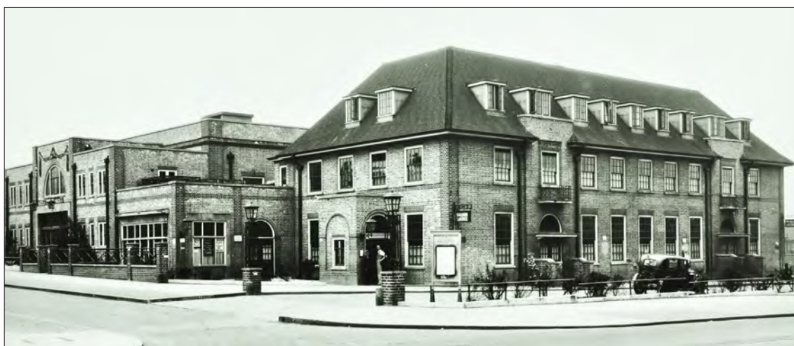
3.15 The Downham Tavern, Bromley, London, one of the largest and most significant pubs of the inter-war period. It was built by Barclay Perkins on a new LCC estate in 1929-30, to designs by F. G. Newnham and W. H. Fleeming, and was innovative and daring in certain aspects of its design – most controversially, as built, the pub contained no bar counters, customers being served by waiting staff. The Downham Tavern was demolished in c. 1995. (© London Metropolitan Archives, City of London: SC/PHL/02/0793/82/3464)
