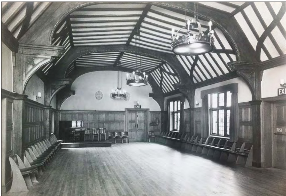
5.33 The striking interior of the first-floor social hall at the Stoneleigh Hotel, Ewell, Surrey (1934-35, by A. E. Sewell), which survives as built. (London Metropolitan Archives, City of London, B/THB/D/398, from the Truman Hanbury Buxton and Co. Ltd collection; copyright Heineken UK)
