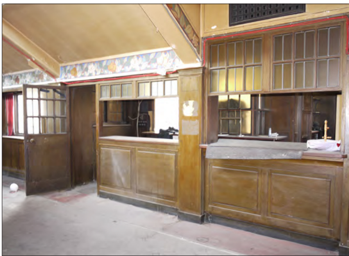
5.25 Counters in pubs built under the state management scheme in the Carlisle district were often of limited size and divided from the bar area by glazed screening. This was the case, for instance, with the first-floor rooms of the Apple Tree in central Carlisle (1927, by Harry Redfern; listed grade II). Shown here is the counter of the first-floor room reserved for 'men 1st class'. (© Historic England, Clare Howard)
