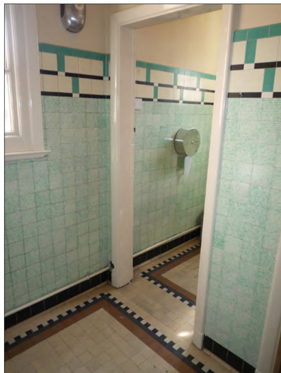
5.39 The tiled interior of the women's lavatories on the first floor of the Test Match Hotel, West Bridgford, Nottingham (1938; listed grade II*), adjacent to the cocktail lounge. The provision of adequate and convenient toilets was a development of pub planning in the inter-war years. (© Historic England, Emily Cole)
