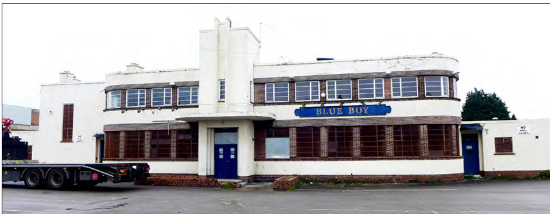
1.3 The Blue Boy pub, Chaddesden, Derby, designed by Browning & Hayes for Offilers brewery and built in 1935-36, in a Moderne style. The pub was closed in c. 2013 and was converted in a mixed scheme of retail and residential units in late 2014. (© Historic England, Luke Jacob)
