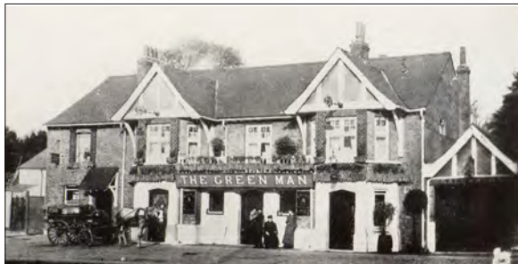
4.2 The Green Man, Southend village, Catford, London, shown before it was 'improved' in an image published in Building in 1927.
