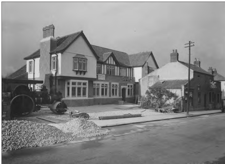
5.3 Some new pubs were built on a site immediately to the rear of their predecessors, and the earlier buildings then demolished, as with the Eastfield Inn, Henleaze, Bristol. The old and new pubs are seen together here in an image of c. 1934, taken shortly after the completion of the new inn. (© Courage Archive, Bristol [Heineken UK])
