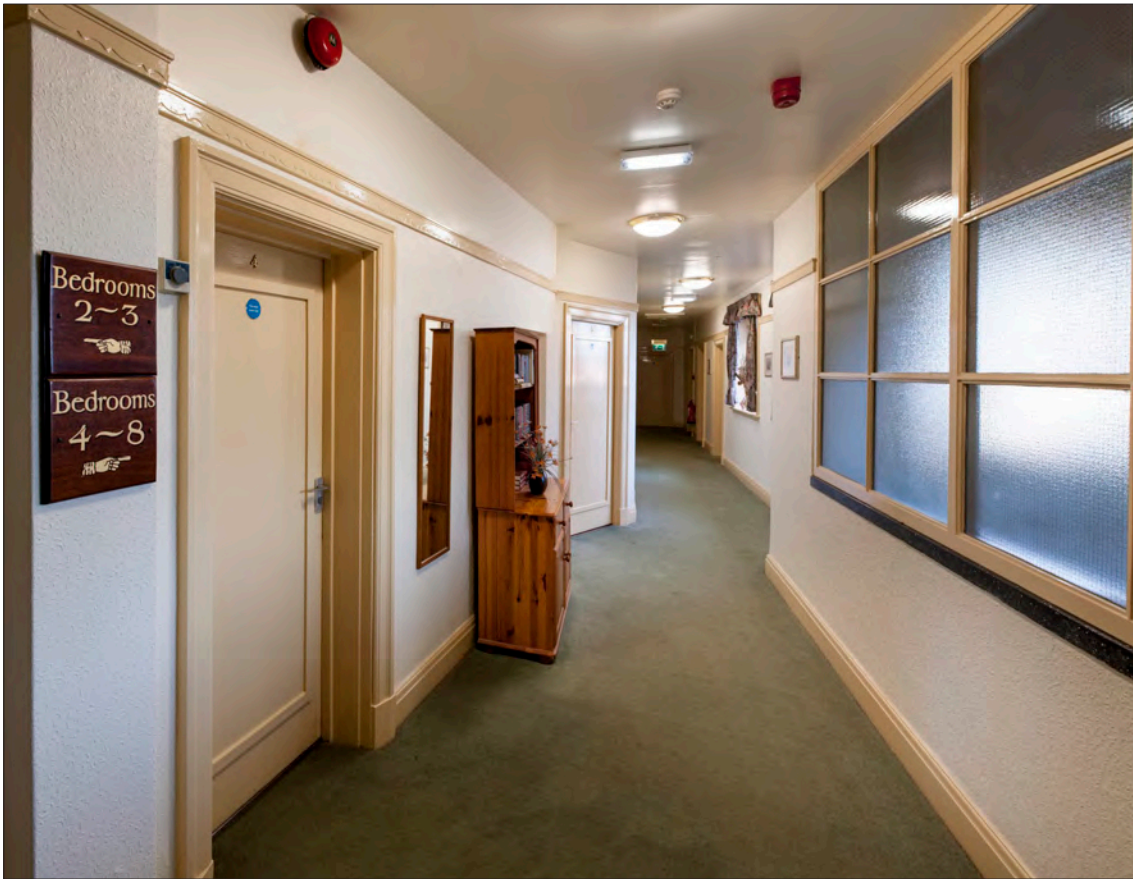
5.28 One of the corridors of guest rooms on the first floor of the Berkeley Hotel, Scunthorpe, Lincolnshire (1938-40, by Scott and Clark). This building is highly unusual in retaining original work in this area. The glazed partition on the right is the most prominent addition; it was probably put in between the corridor and the staircase during the 1970s for fire safety reasons. (© Historic England, Derek Kendall, DPI52483)
