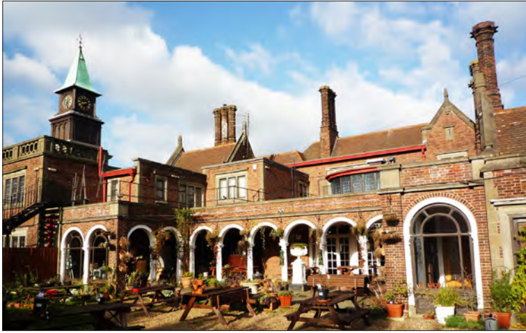
10.5 Some listed pubs are notable in terms of their quality of architecture and design, an example being the Suffolk Punch, Ipswich, Suffolk (1936-37, by Cautley & Barefoot for the Tollemache Brewery; listed grade II). This photograph shows the pub's rear elevation and garden. (© Historic England, Emily Cole)
