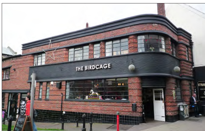
7.10 One of the towns and cities that was a particular focus for pub building in the inter-war period was Norwich. Pubs built included the Morning Star (now the Birdcage ) in Pottergate, which dates from c. 1937 and was a work of Bullards brewery, designed in the Moderne style. It was criticised at the time for its 'incongruous' design within its historic setting; the pub is adjacent to the medieval Church of St Gregory. (© Historic England, Luke Jacob)
