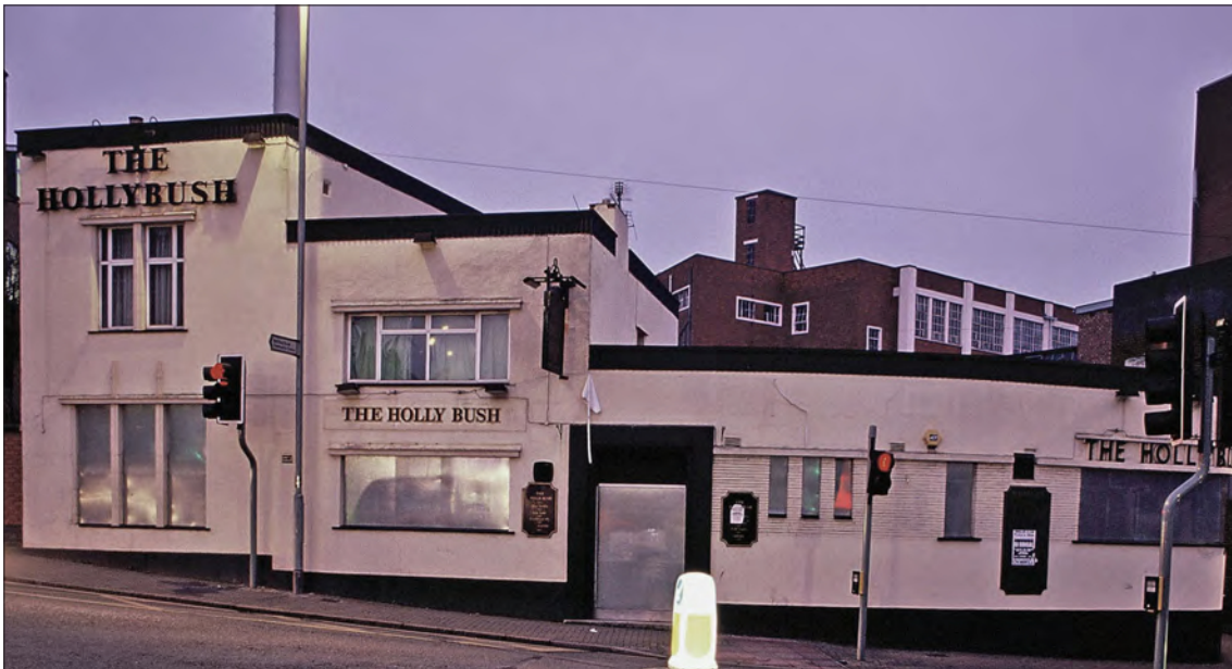
2.10 The Holly Bush pub, Hinckley, Leicestershire, built in the late 1930s. The pub was listed grade II in 2005, but subsequently closed and has now been converted to restaurant use. (© Michael Slaughter LRPS)
