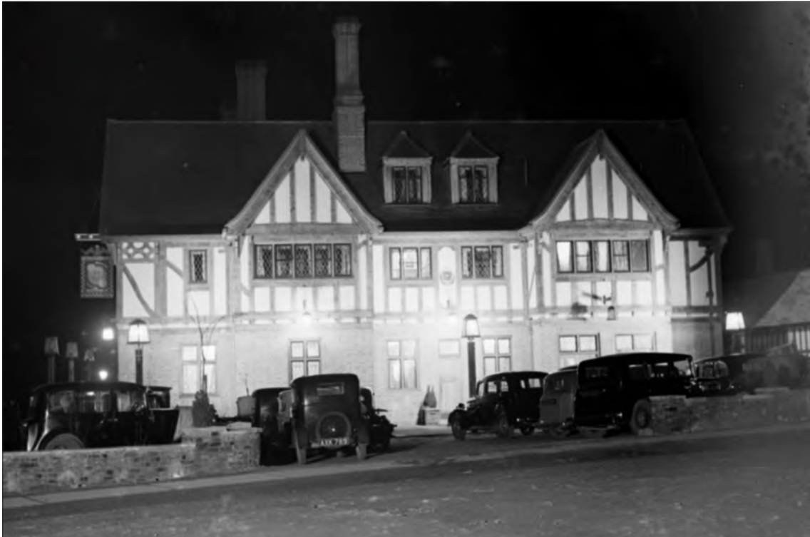
6.2 The north elevation of the Daylight Inn, Petts Wood, London (1935, by Sidney C. Clark), in a photograph of 1936. The car park – placed by the entrance to the pub’s ballroom and enclosed by low boundary walls – is here shown filled with cars. (© TopFoto)
