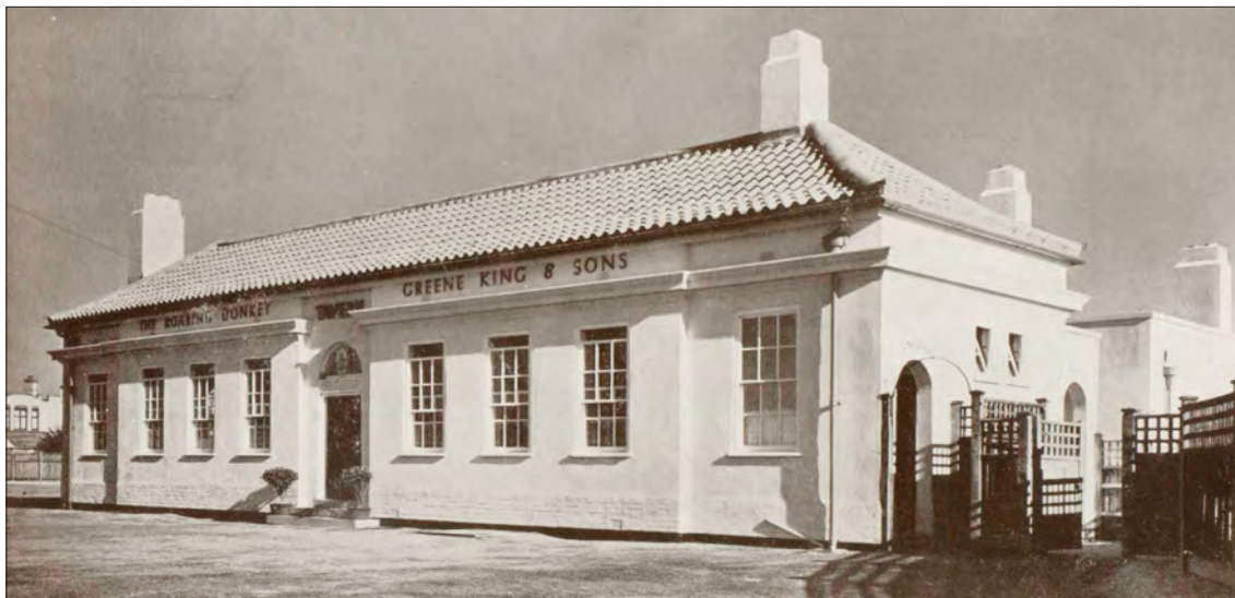
2.4 The Roaring Donkey, Holland-on-Sea, Essex, designed by the noted pub architect Basil Oliver and featured in Architecture Illustrated in 1935. The building has since been much altered but remains a pub.
