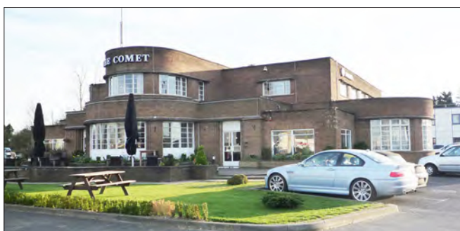
5.14 The Comet, Hatfield, Hertfordshire, built in 1933 to designs by E. B. Musman and commissioned by Benskin’s Watford Brewery. The building, now a Ramada hotel, is listed grade II, and is notable for its Moderne style. Its design was widely acclaimed at the time. (© Historic England, Luke Jacob)
