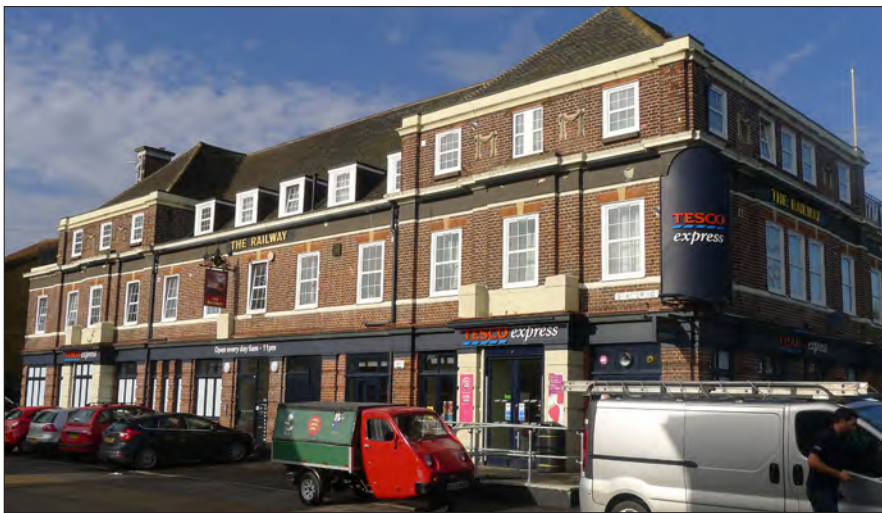
2.5 An example of a much altered inter-war pub is the former Railway Hotel, Dagenham, London, converted to a Tesco in c. 2012. All original windows have been replaced and the interior greatly reworked. (© Historic England, Luke Jacob)
