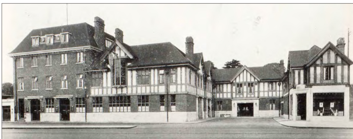
4.3 The Green Man, Southend village, Catford, London, following rebuilding, as illustrated in Building. The new pub, completed in 1927 for Watney's, was of a substantial size; it was designed by Grace & Grace & Farmer, with M. T. Saunders. The four-storey block on the left contained public and private bars on the ground floor, kitchen on the first floor, and staff accommodation on the two upper floors. The saloon bar, saloon lounge, assembly hall and other higher-class rooms were in the pub's timbered section, while a block on the right contained an off licence.
