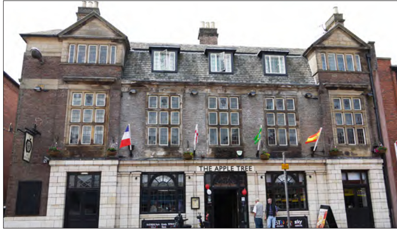
3.5 The pubs rebuilt and newly constructed in the Carlisle district under the state management scheme were of huge significance to the development of the public house in England. The first newly built 'model' pub, designed by the scheme's architect Harry Redfern, was the Apple Tree, central Carlisle, completed in 1927 (listed grade II). (© Historic England, Luke Jacob)
