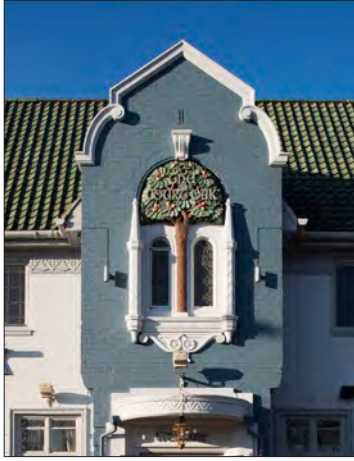
5.18 A detail of the main façade of the Court Oak, Quinton, Birmingham (1932), showing the carved pub sign and the original green pantiles. The sign is probably the work of William Bloye or one of the sculptors in his circle. (© Historic England, James O. Davies, DPI66395)
