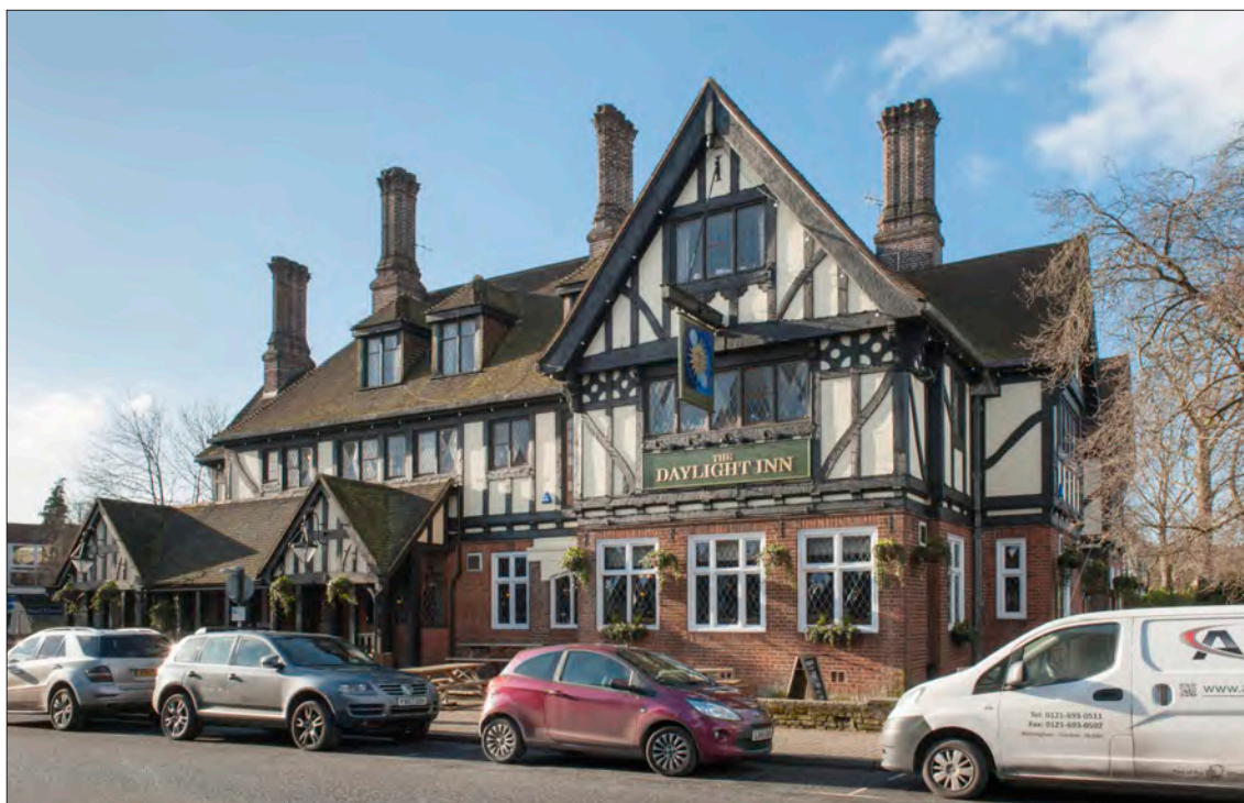
12.14.1 The Daylight Inn seen from the north-east. The single-storey gabled extension on the left of the picture was added in 1996, in sympathetic style. (© Historic England, Derek Kendall, DPI70023)
