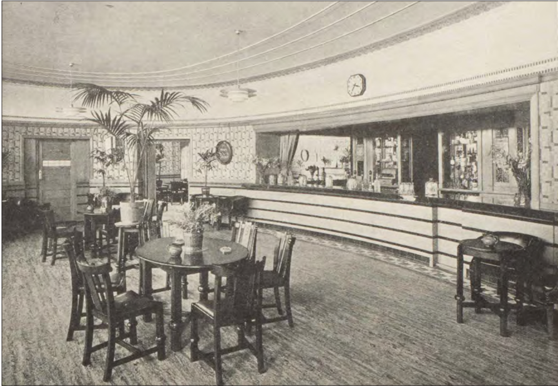
12.31.4 The interior of the oval lounge/luncheon room at the rear of the Round House, as featured in The Builder in 1936.
