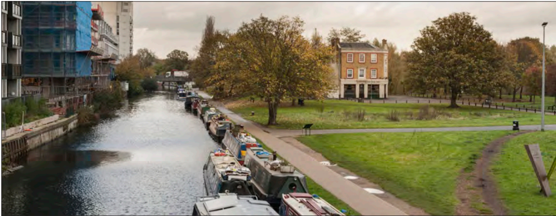
12.25.1 The Palm Tree seen from a bridge over the Grand Union (Regent's) Canal. The pub is now in an isolated location, but was once part of a network of streets. (© Historic England, Derek Kendall, DPI52169)
