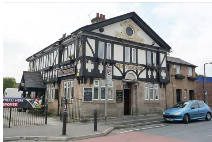
12.27.3 The pub's side elevation to Withens Lane, with its bullseye window and decorative surround at attic level. The side doorway led to the off sales area, and also to the parlour, with access to the other main rooms of the pub. (© Historic England, Emily Cole)
