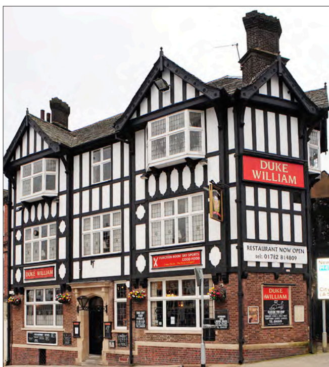
12.17.1 The exterior of the Duke William, facing onto St John's Square. There has been a pub on the site since at least 1818. (© Michael Slaughter LRPS)
