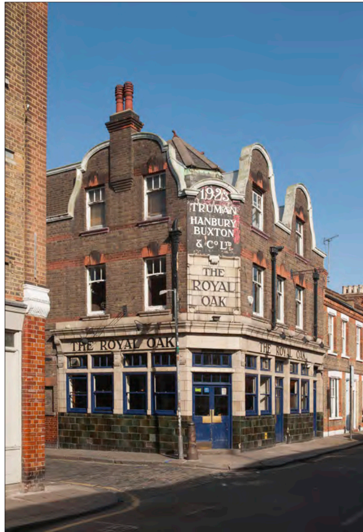
12.32.2 The pub seen from Columbia Road. The exterior has been very little altered since the building's completion in 1923. (© Historic England, Derek Kendall, DPI70190)
