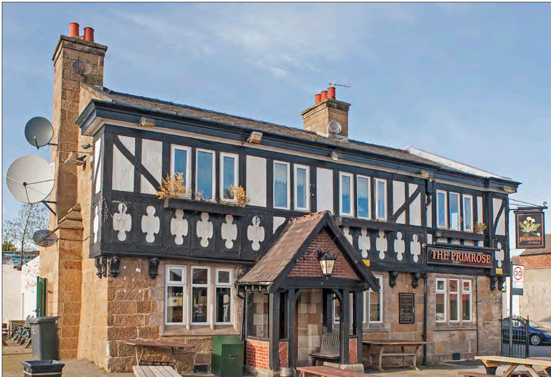
12.27.1 The main (south-east) elevation of the Primrose. Aside from the replacement windows, the pub appears to survive largely as rebuilt in 1922-23. (© Michael Slaughter LRPS)
