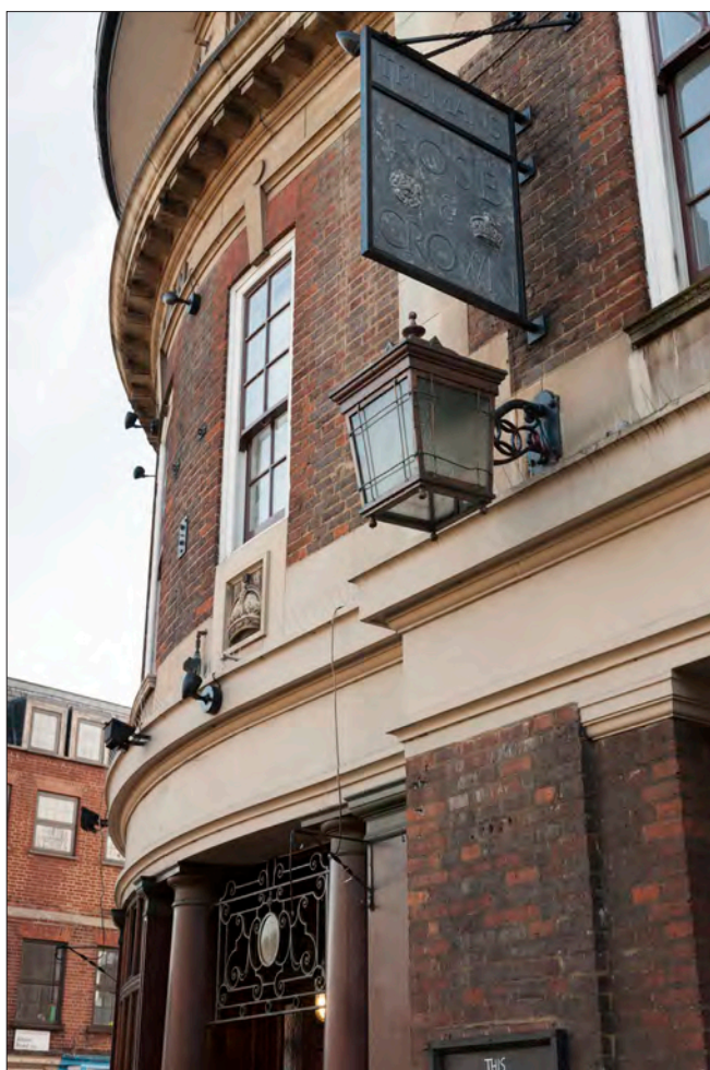
12.30.3 A detail of the north elevation of the Rose and Crown. The metal hanging sign is original work of 1932, as are the glazed lamp and the decorative ironwork at ground-floor level, above the entrance to the private bar. The sign – one of a pair – and the pub's ironwork are the work of the notable art foundry Morris Singer Co. (© Historic England, Derek Kendall, DPI52305)
