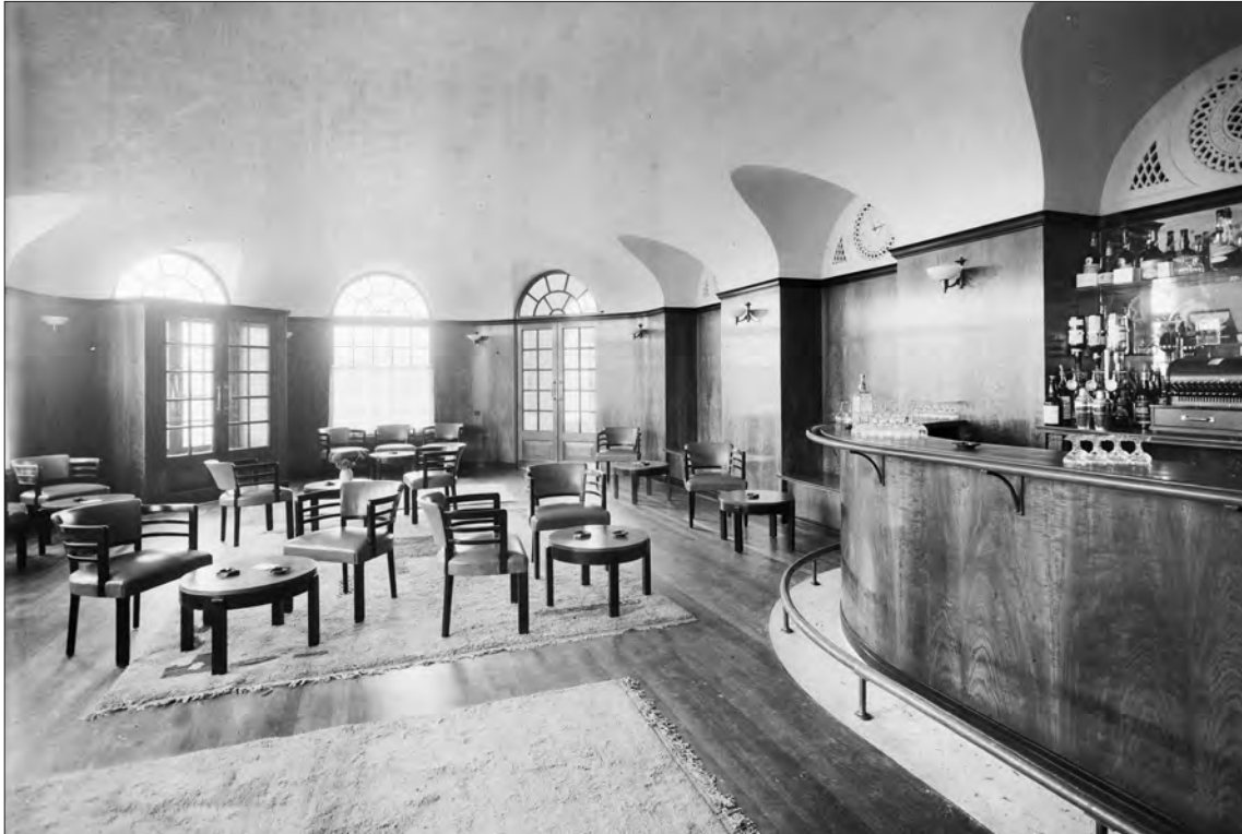
12.24.4 The elegant interior of the pub's saloon lounge, in a photograph taken shortly after its completion. The room had a vaulted ceiling and was panelled in teak. Drinks served here included tea and cocktails. (Reproduced by permission of Historic England)
