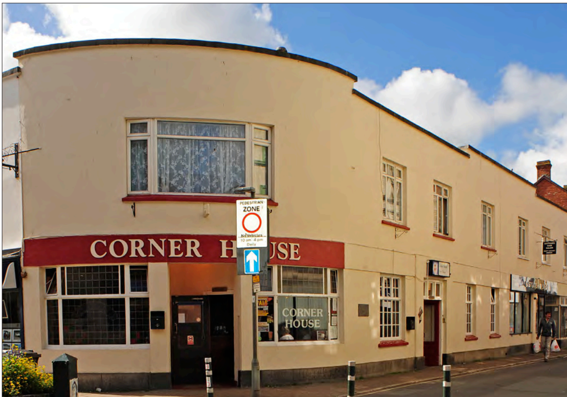
12.12.1 The exterior of the Corner House. Some of the ground-floor windows are original, but those on the first floor have been replaced with uPVC, including the window in the pub's curved corner. (© Michael Slaughter LRPS)
