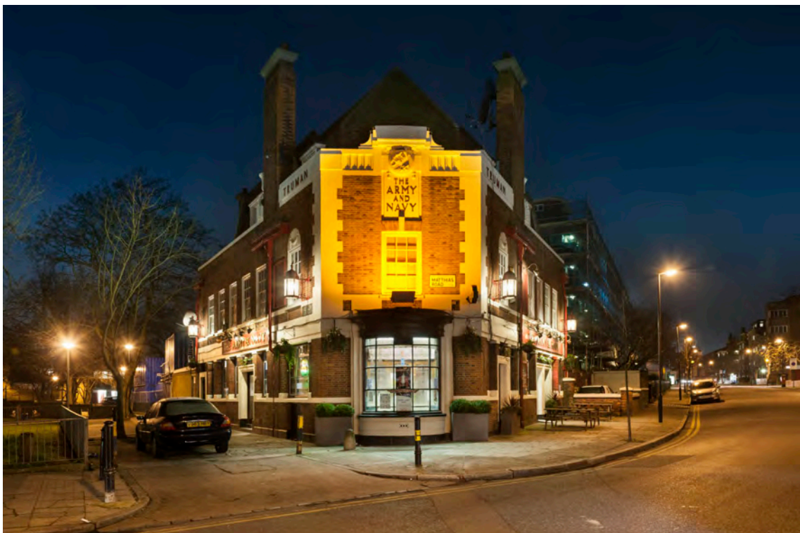
12.2.2 The Army and Navy today, with its original display window and pub sign illuminated. (© Historic England, Derek Kendall, DPI70131)
