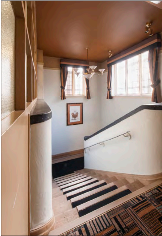
12.5.8 The guest staircase at the centre of the pub's plan, seen from the first-floor landing. The glazed screening on the left is an insertion of the 1970s, added for fire safety reasons. (© Historic England, Derek Kendall, DPI52482)
