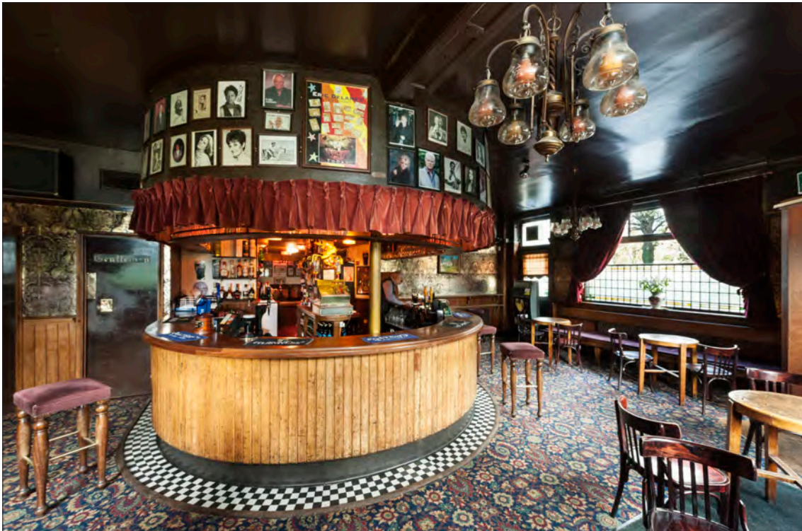
12.25.6 The interior of the Palm Tree's main bar. As is shown by the ceiling breaks, this was originally divided into three spaces: private bar, public bar and off sales compartment, the latter accessed by the door which can be seen on the right of the picture. Original work includes the counter and chequer-tiled border, though the canopy and gantry/glass shelf were added in about 1980. (© Historic England, Derek Kendall, DPI52193)
