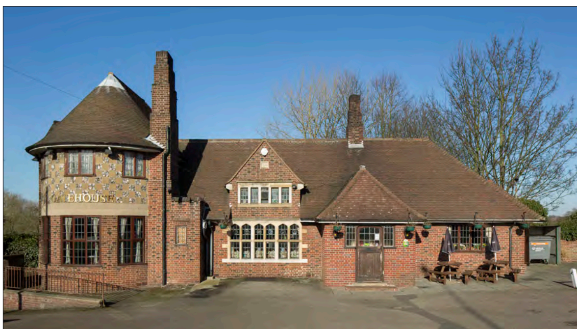
12.20.1 The main elevation of the Gate House survives largely as built. The entrance porch is an addition, but is sympathetic in style and reuses original work. The pub is notable for its distinctive design, influenced by the Arts and Crafts and local vernacular traditions. (© Historic England, Patricia Payne, DPI72331)
