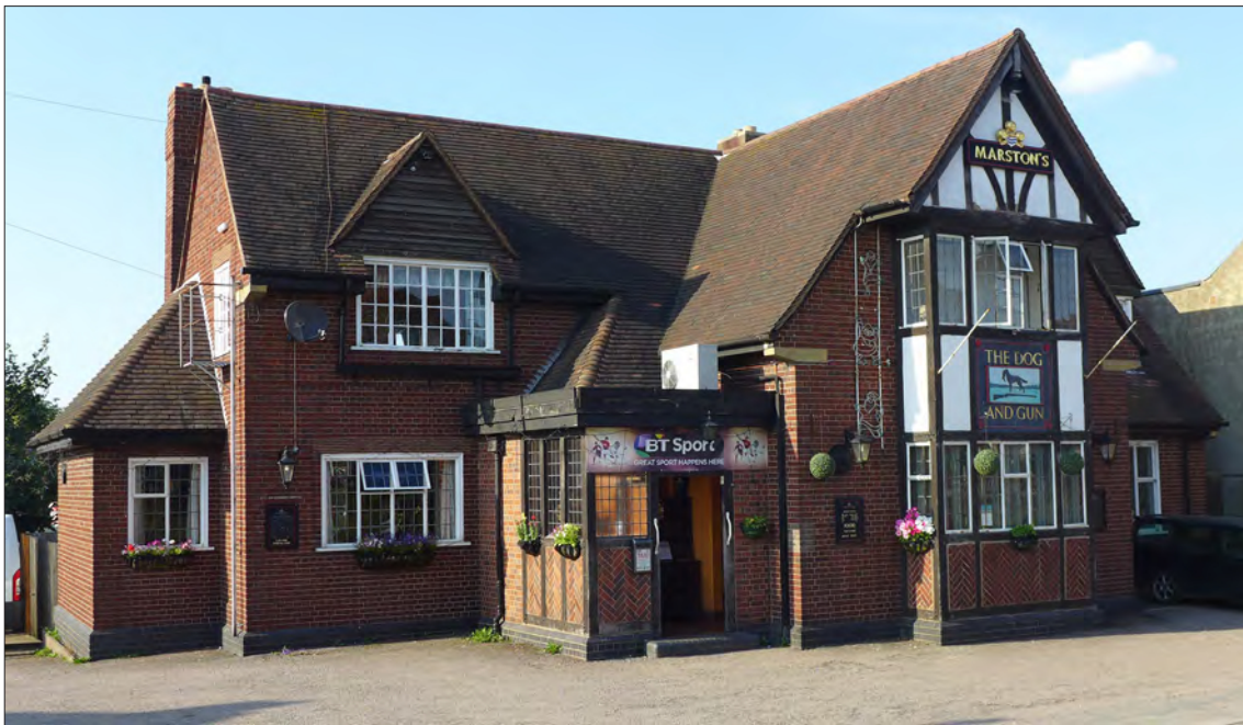
12.15.1 The exterior of the Dog and Gun, which remains largely as completed in 1932. (© Historic England, Luke Jacob)
