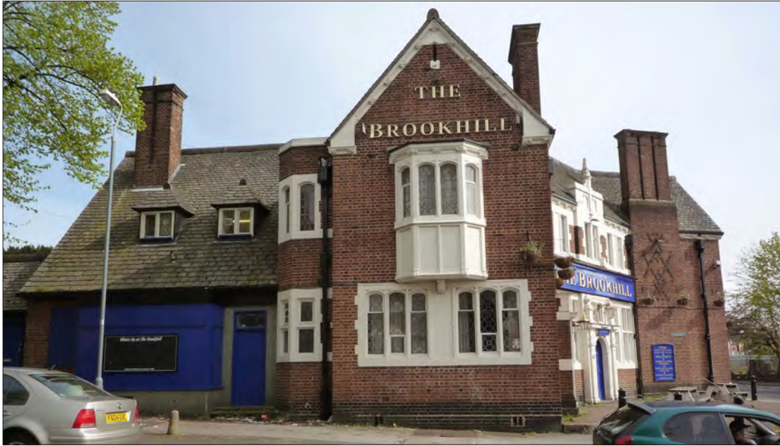
12.9.2 The Brookhill Tavern in April 2014, seen from Brook Hill Road. The shopfront on the left of the image seems to have been inserted around the late 1950s, and probably served as an off licence. It occupies the site of the pub's original off sales compartment. (© Historic England, Emily Cole)
