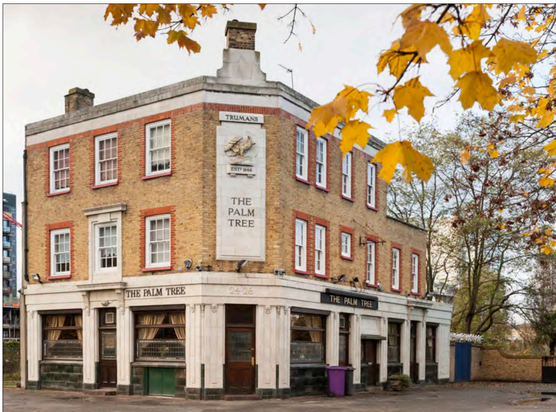
12.25.3 The exterior of the Palm Tree, which was a comparatively early inter-war building project for Truman's brewery. (© Historic England, Derek Kendall, DPI52175)
