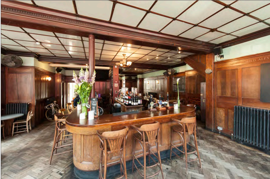
12.32.4 The interior of the Royal Oak, now unified, looking north-west. Original features include the Vitrolite ceiling, the island servery and the panelling. The saloon bar was originally on the left and the public bar on the right, the two areas divided by an off sales compartment. (© Historic England, Derek Kendall, DPI70451)
