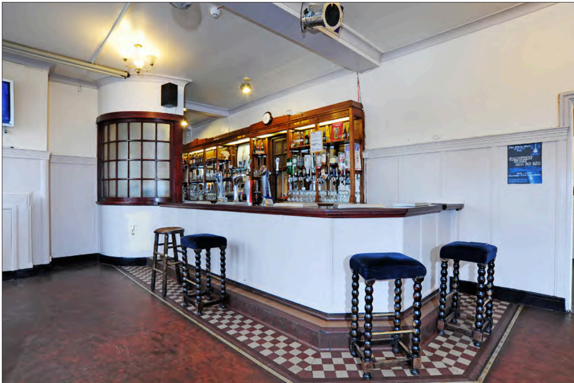
12.36.3 The interior of the saloon bar. The counter, panelling and fireplace are all original, but have now been painted white. The glazed screen would have served to give privacy and borrowed light to the adjacent off sales compartment. (© Historic England, Luke Jacob)
