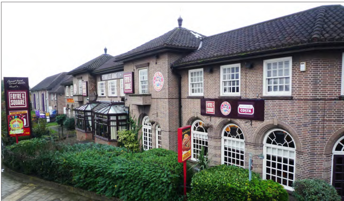
12.24.1 The Myllet Arms seen from the north-west. The glazed conservatory is a modern addition, as is the signage, but the exterior of the pub otherwise survives largely unaltered. (© Historic England, Emily Cole)
