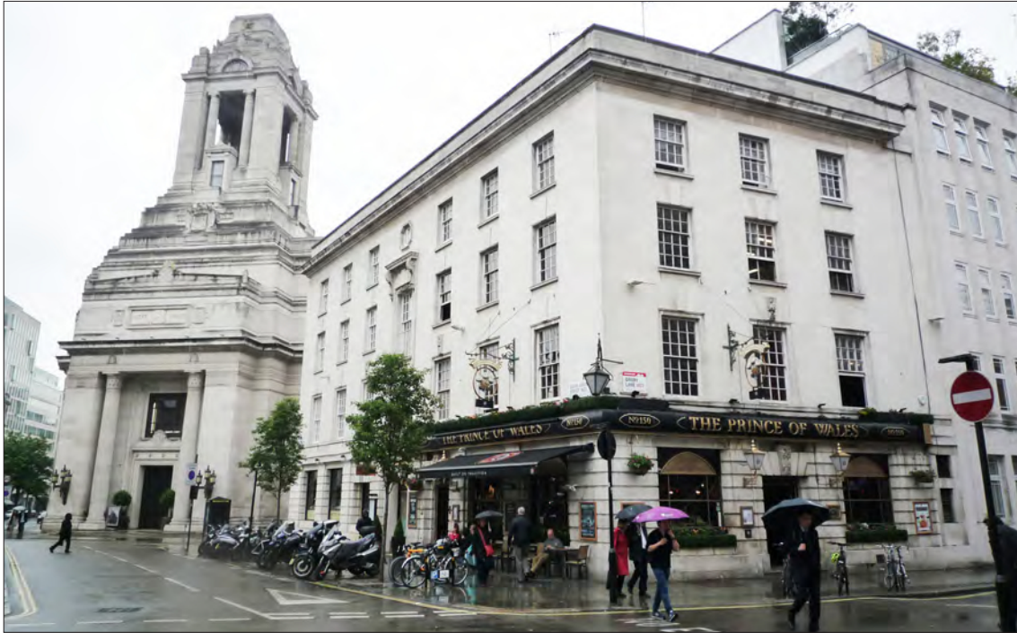
12.28.1 A modern view of the Prince of Wales, taken from Drury Lane, with the Freemasons' Hall of 1927-33 (listed grade II*) on the left of the photograph. (© Historic England, Emily Cole)
