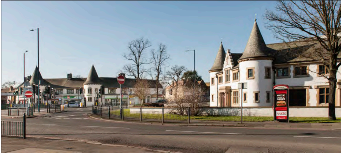
12.4.1 A view showing the former Berkeley Arms Hotel on the right and, on the opposite side of the crossroads on the left of the image, one of the shopping parades which were built in 1934 in a design which imitates that of the pub. E. B. Musman successfully sued the architects of the shopping parades for copying his pub design. (© Historic England, Derek Kendall, DPI70182)
