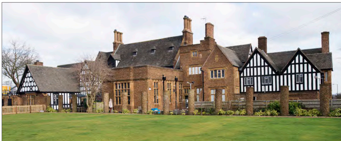
12.7.2 The rear elevation of the Black Horse, with the bowling green in the foreground. The pillared screen is original, but it has lost its horizontal lintel stones. (© Historic England, James O. Davies, DPI66446)
