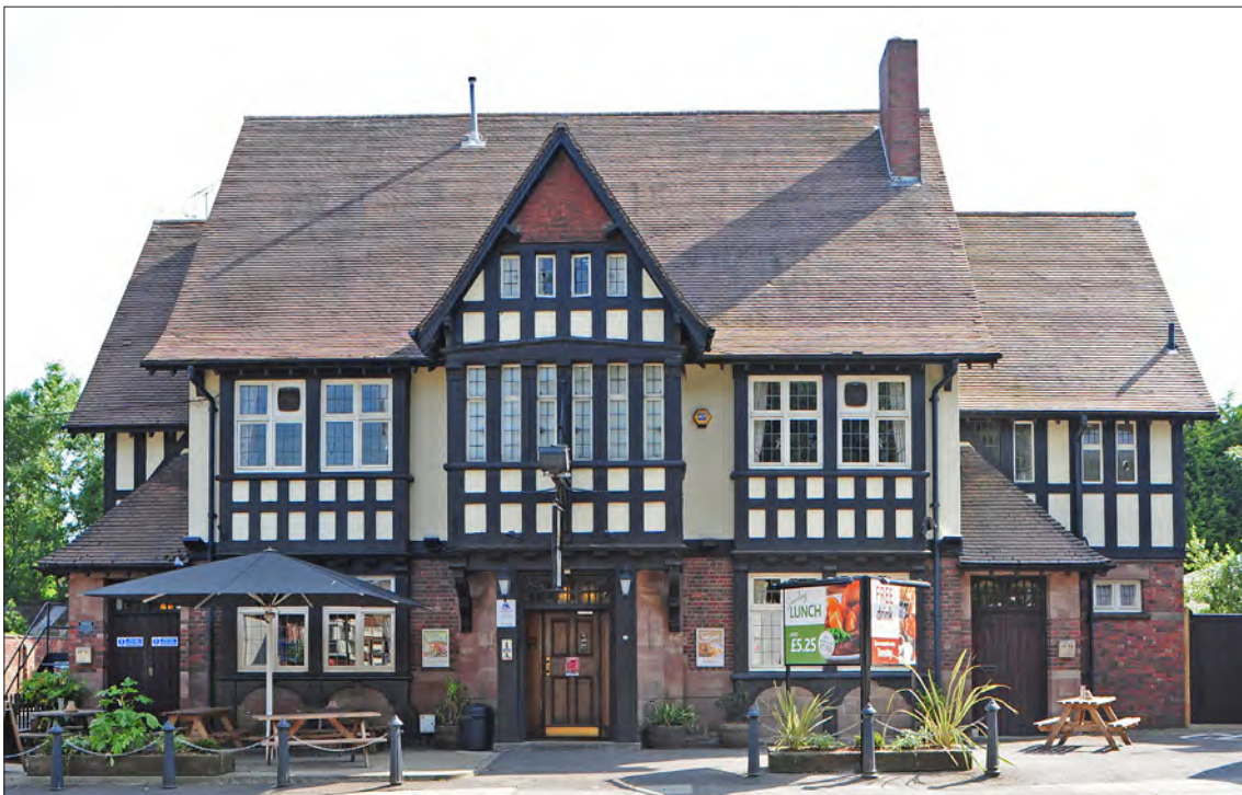
12.6.1 The main (north) elevation of the Biggin Hall Hotel. (© Michael Slaughter LRPS)
