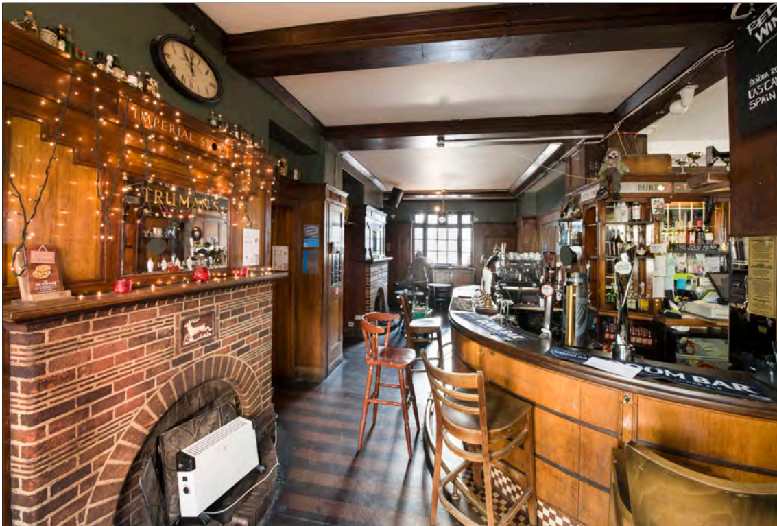
12.33.4 The east (left-hand) side of the Stag's Head, which contained the saloon bar and, to the rear, what was probably a saloon dining room, both served by brick fireplaces and a Moderne-style counter. Doorways have been inserted in the left wall to provide access to the function room block added in c. 1970. (© Historic England, Derek Kendall, DPI52388)
