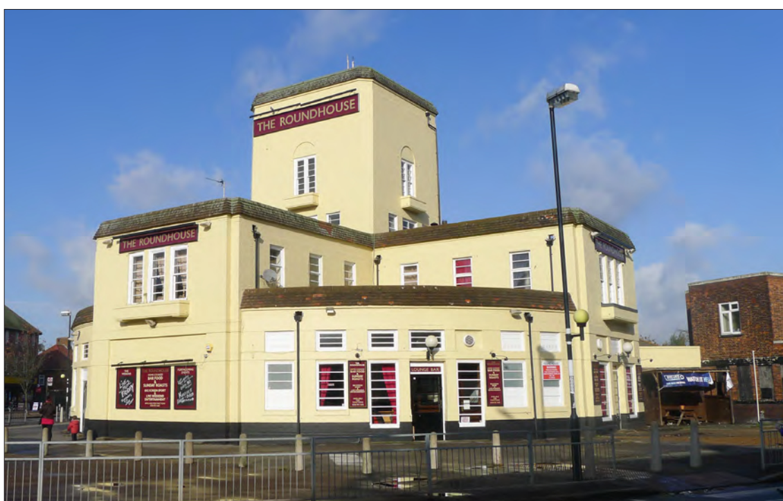
12.31.1 The striking exterior of the Round House, seen from Porters Avenue. The ground floor of the two-storey block on the left of the image originally contained an off licence with showcase windows (see Fig. 5.16), but this area has since been infilled. (© Historic England, Luke Jacob)
