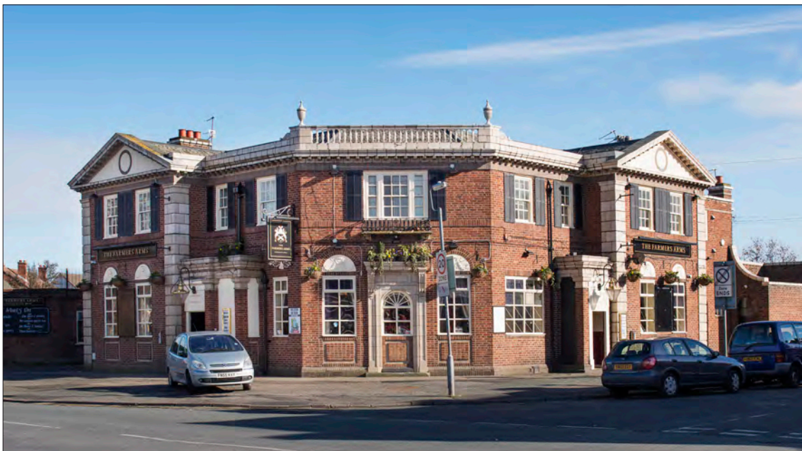
12.19.1 The main elevations of the Farmers' Arms, seen here from the north-west, survive almost entirely as completed in the inter-war period. The pub's striking Neo-Georgian design is typical of the work of Harold E. Davies & Son. (© Historic England, James O. Davies, DPI66553)
