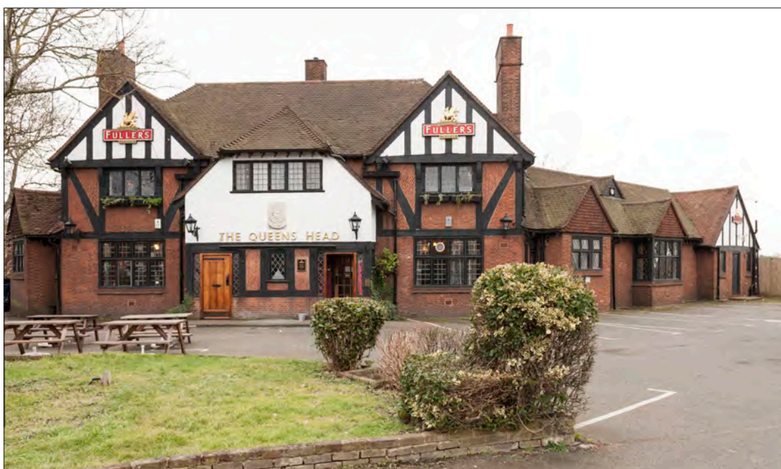
12.29.1 The Queen's Head seen from the north-west. The single-storey wing on the right contains the former saloon lounge, while the pub's 'draw in' and car park can be seen in the foreground. (© Historic England, Derek Kendall, DPI70056)
