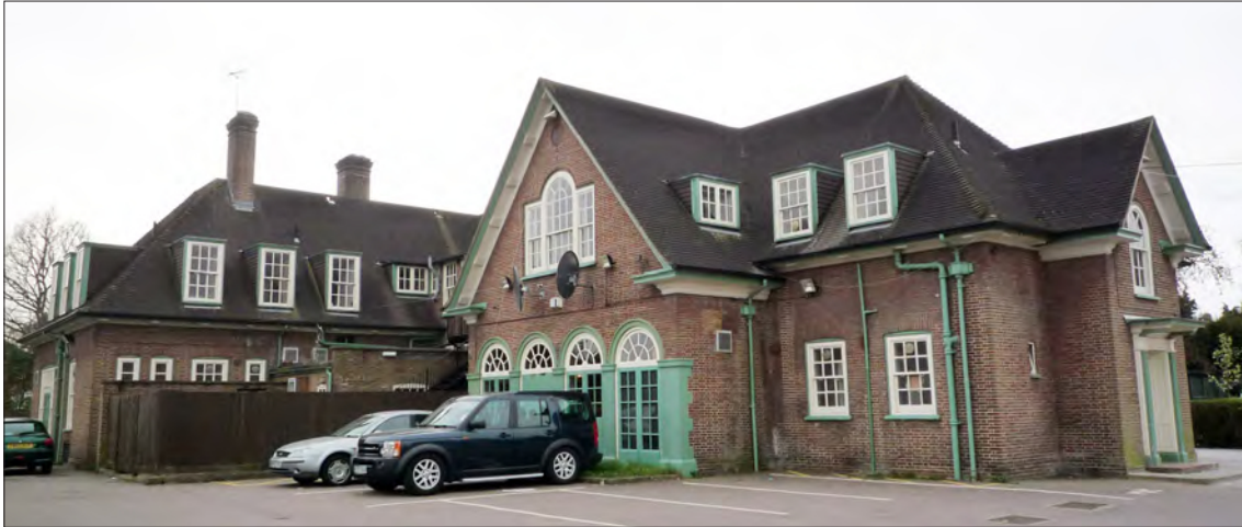
12.26.2 The Pear Tree seen from the north-east. The car park was always to the north of the pub. The doorway on the right of the image leads to the stairhall which provides access to the first-floor club room, lit by Venetian windows at each end. (© Historic England, Luke Jacob)
