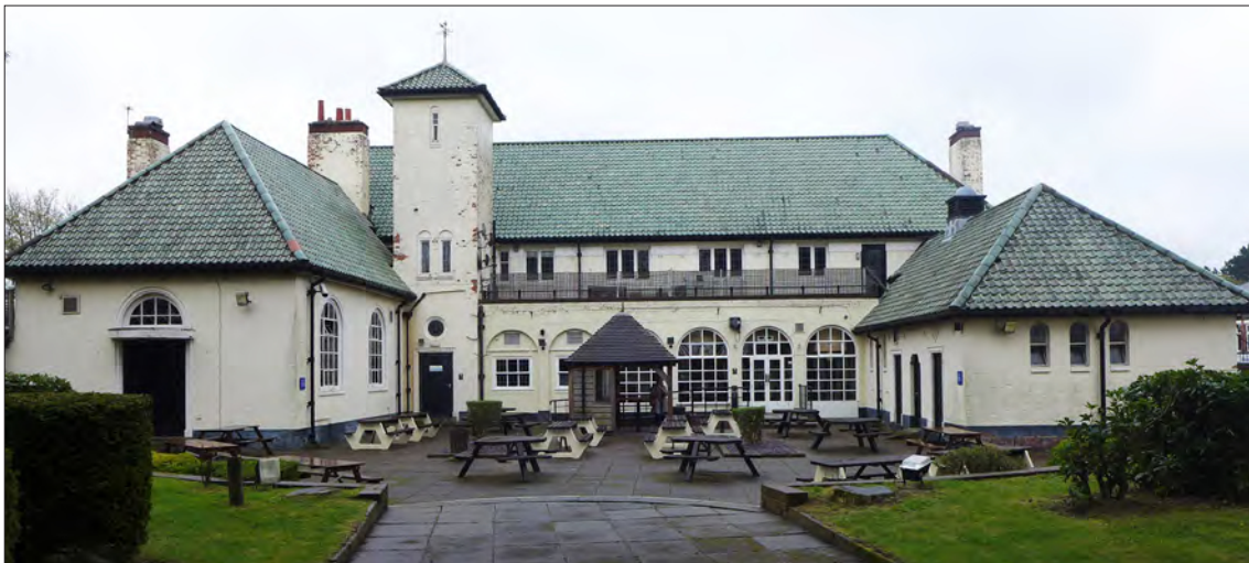
12.13.3 The pub's rear elevation, with its tower and two projecting wings. The arcaded section at the centre was probably originally an open loggia. (© Historic England, Luke Jacob)
