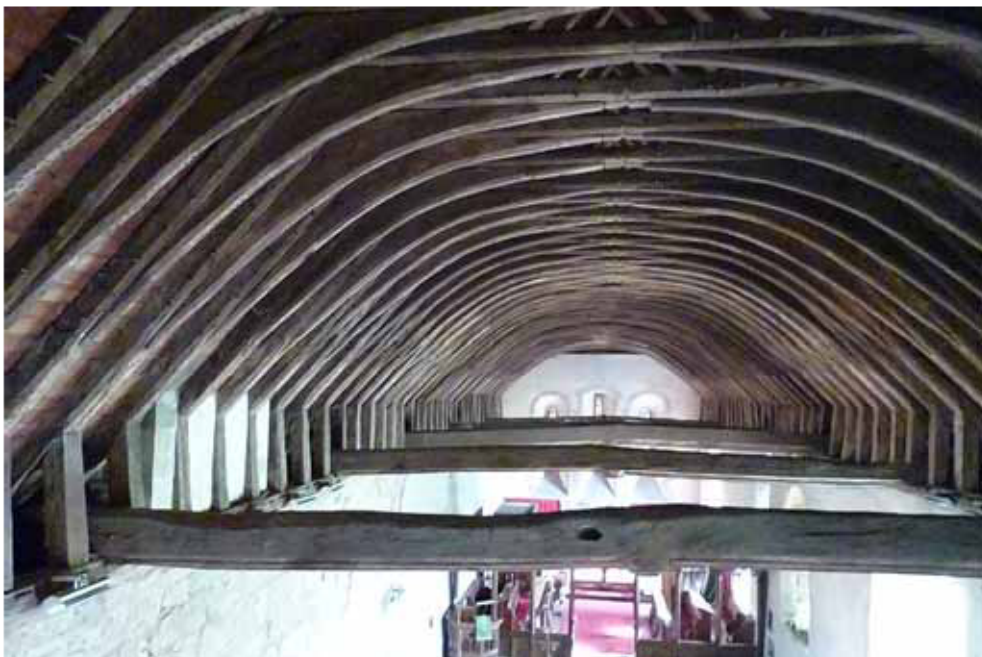
Figure 3: View of the nave roof looking west to east (photograph Robert Howard)
