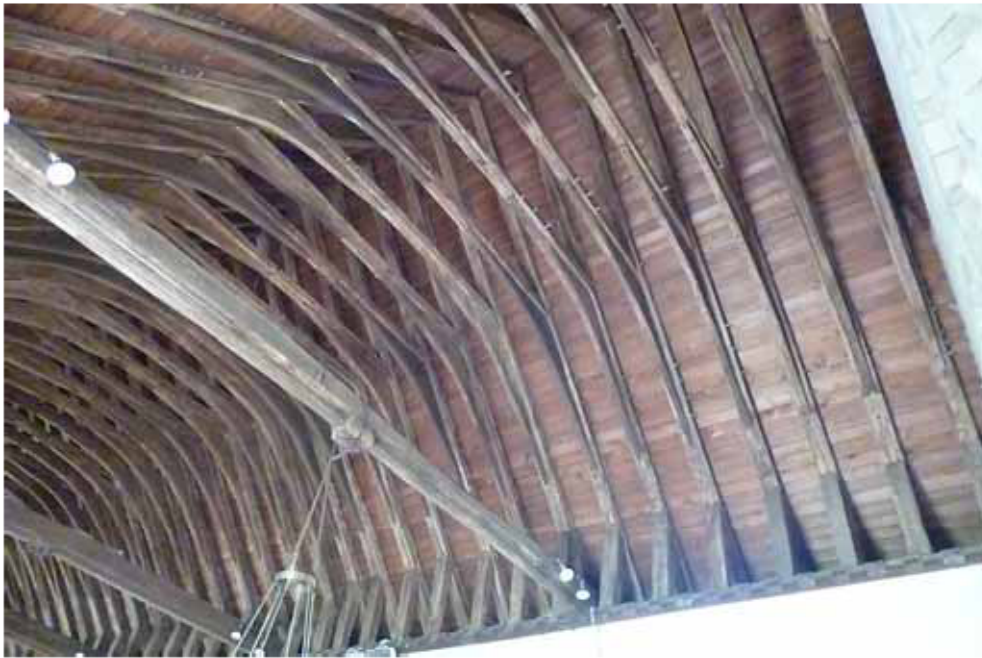
Figure 2: View of the chancel roof of St Mary's Church (photograph Robert Howard)
