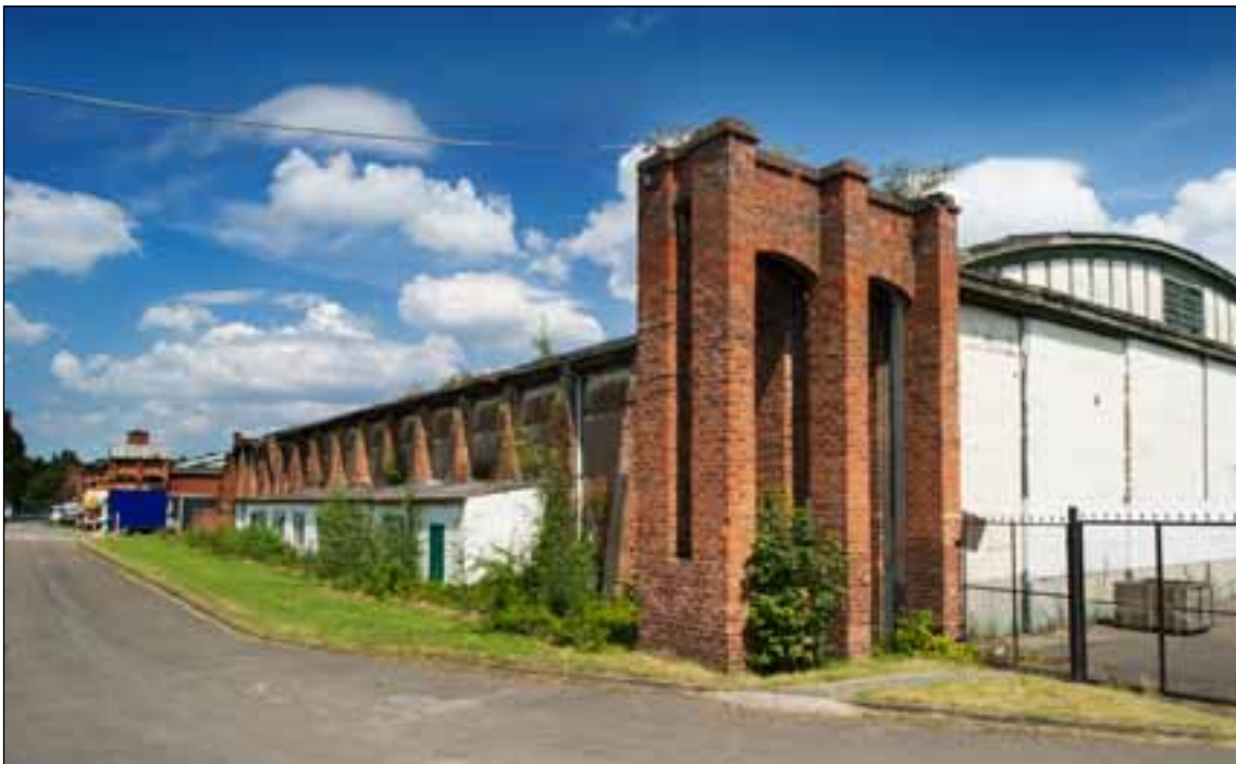
Figure 14: Building 18 from the south (DPI68379 © English Heritage, photograph: Alun Bull).
