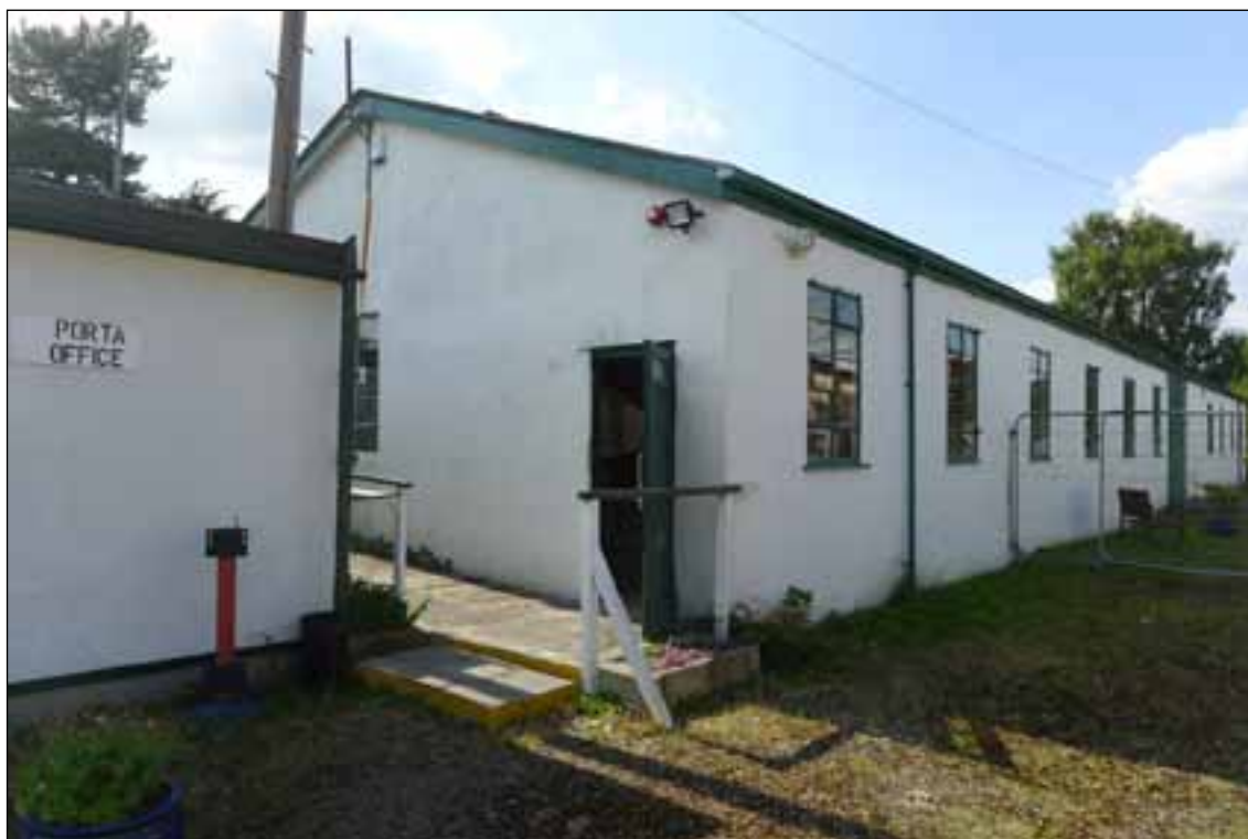
Figure 28: Building 27 from the south-east (© English Heritage, photograph: Clare Howard).
