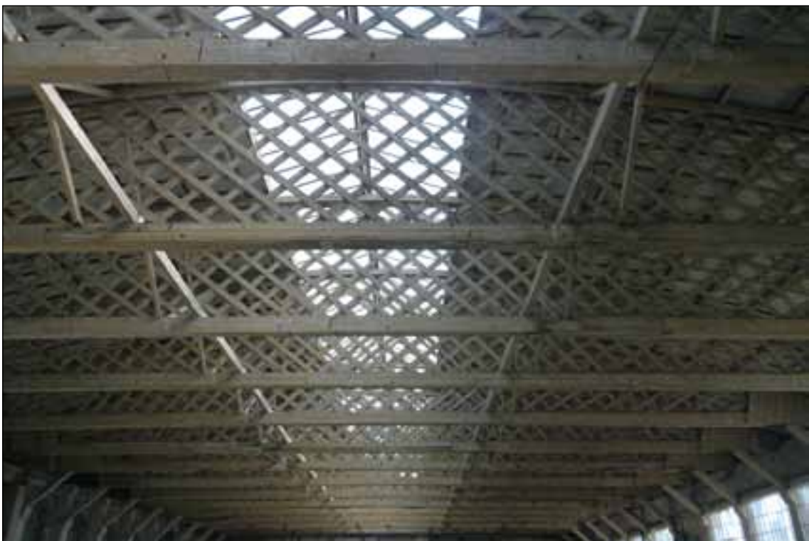
Figure 16: Belfast trusses in Building 17 (© English Heritage, photograph: Simon Taylor).
