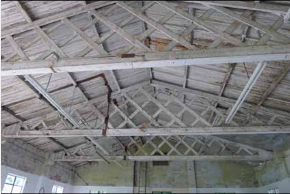
Figure 30: Wooden lattice roof trusses in Building 42 (© English Heritage, photograph: Clare Howard).
