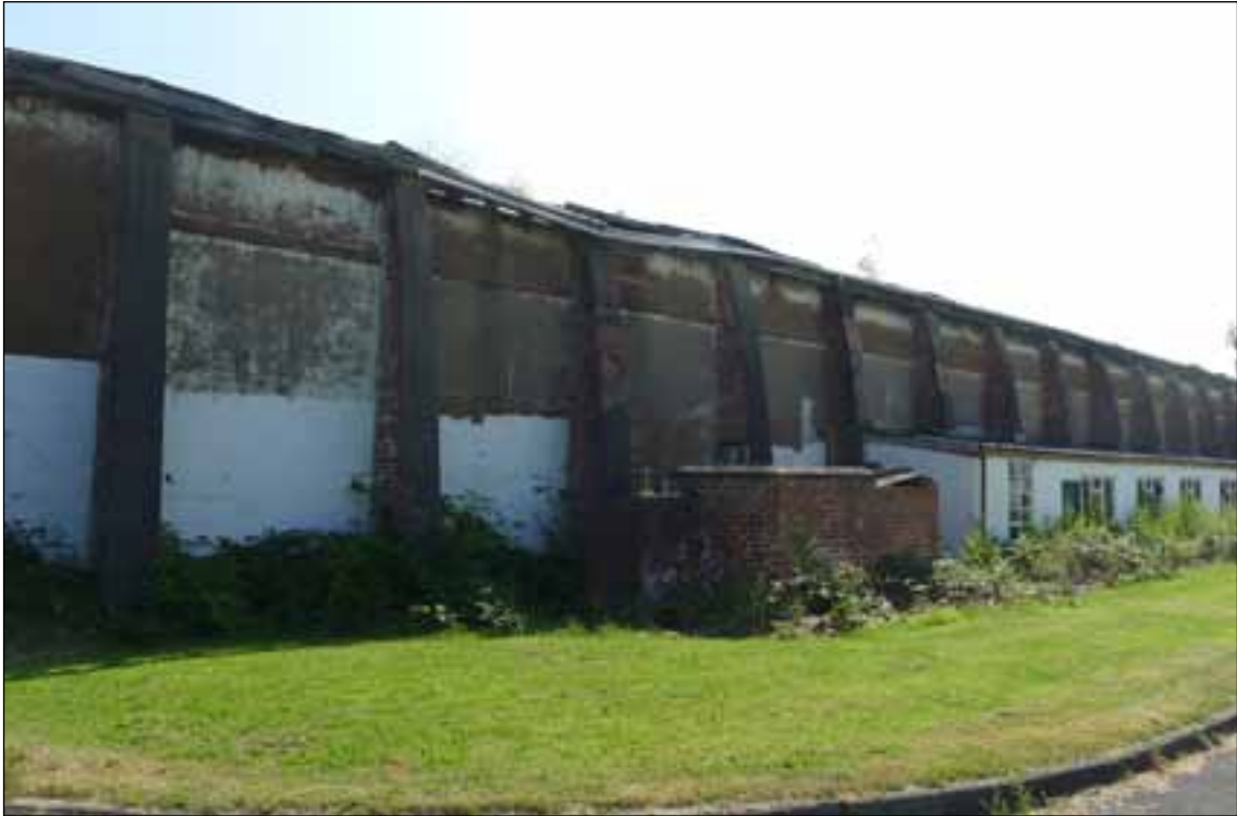
Figure 25: Annexe and sanitary addition, Building 18 (© English Heritage, photograph: Clare Howard).
