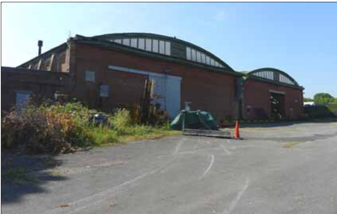
Figure 27: Building 18 from the north (© English Heritage, photograph: Clare Howard).
