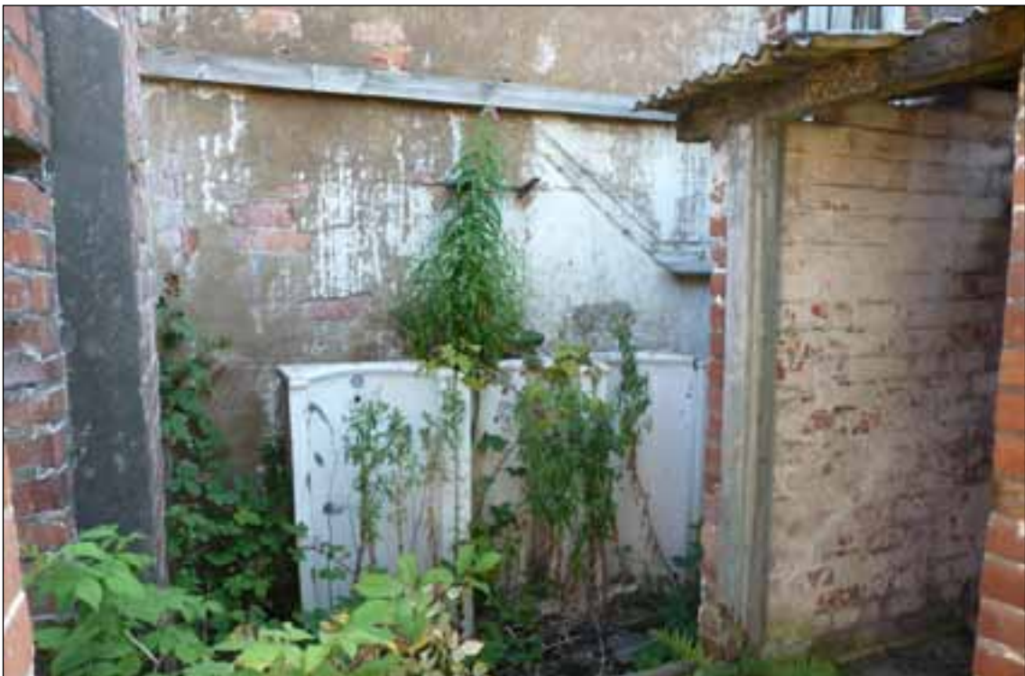
Figure 26: Urinals within the sanitary addition, Building 18 (© English Heritage, photograph: Allan Adams).
