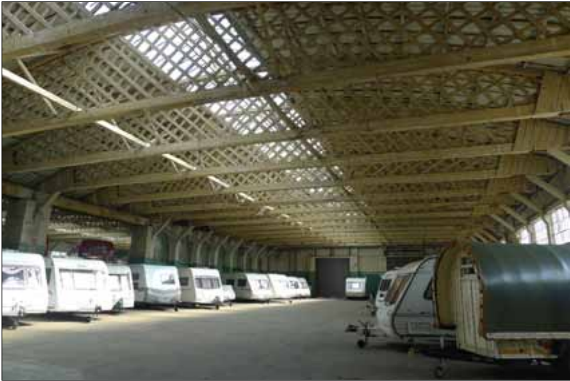
Figure 15: Interior of Building 17 (© English Heritage, photograph: Clare Howard).
