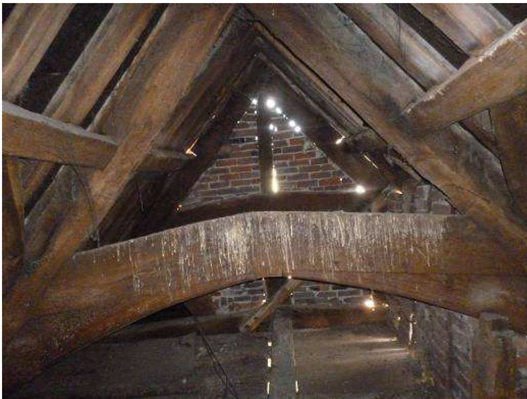
Figure 2a/b: Views of the impressive timber framing to the first floor (top) and the inaccessible trusses (bottom) (photographs Robert Howard)
