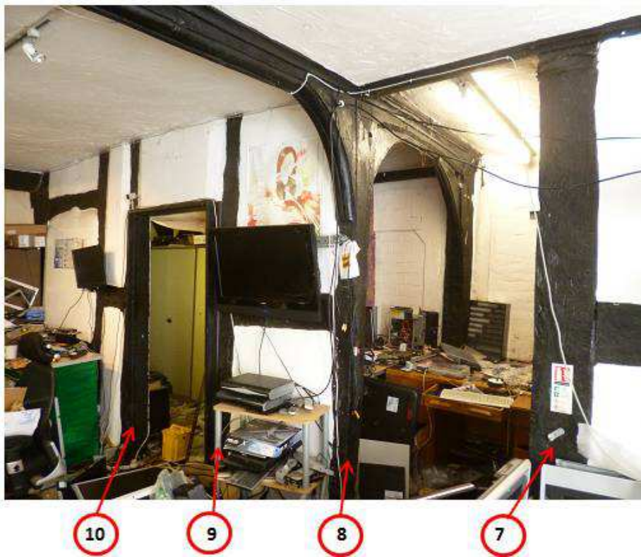
Figure 4a/b: Views to help locate sampled roof (top) and ground-floor timbers (bottom) (photographs Robert Howard)
