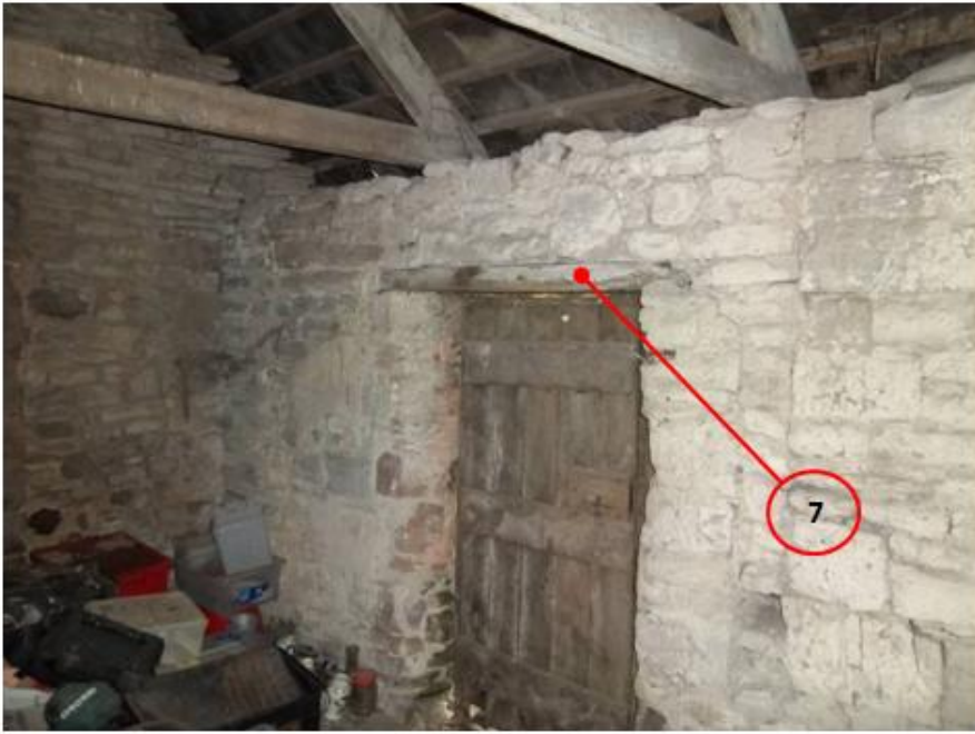
Figure 8g: KLV-A07: first floor, west wall, south window lintel (photograph Robert Howard)
