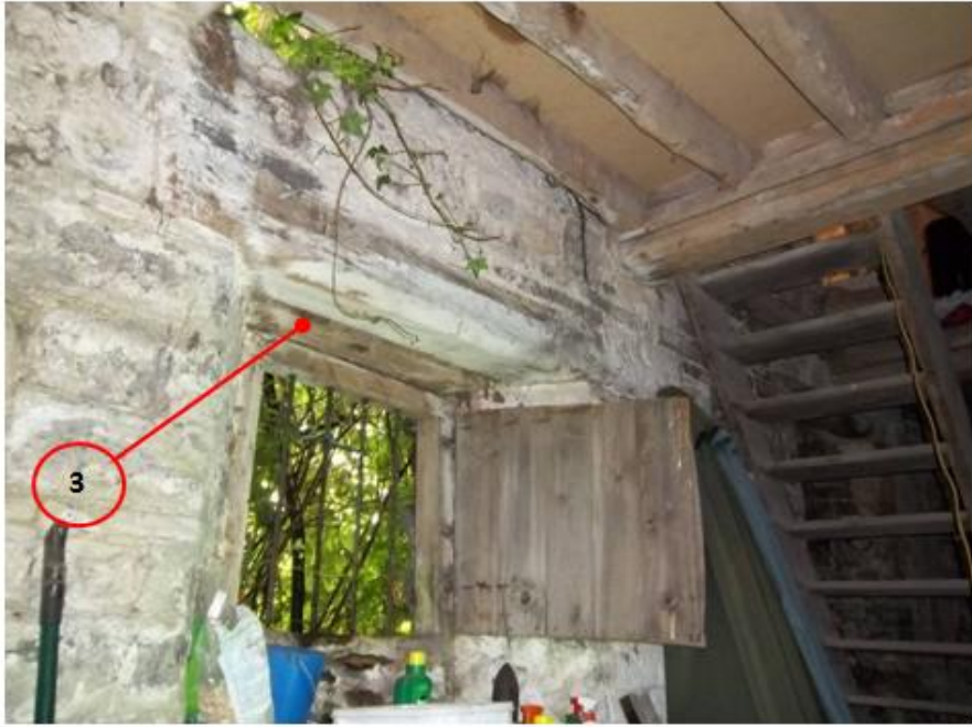
Figure 8c: KLV-A03: ground floor, west wall, south window, outer lintel (photograph Robert Howard)
