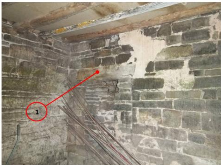
Figure 8a: KLV-A01: ground floor, east wall, north window, inner lintel (photograph Robert Howard)
