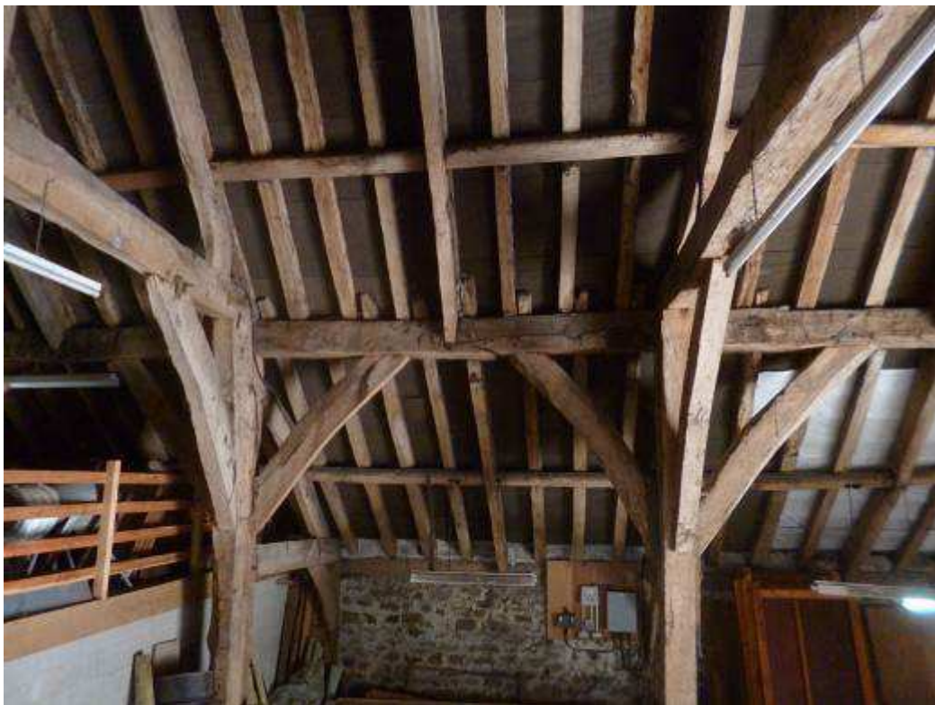
Figure 4a/b: Views of the trusses (photographs Robert Howard)
