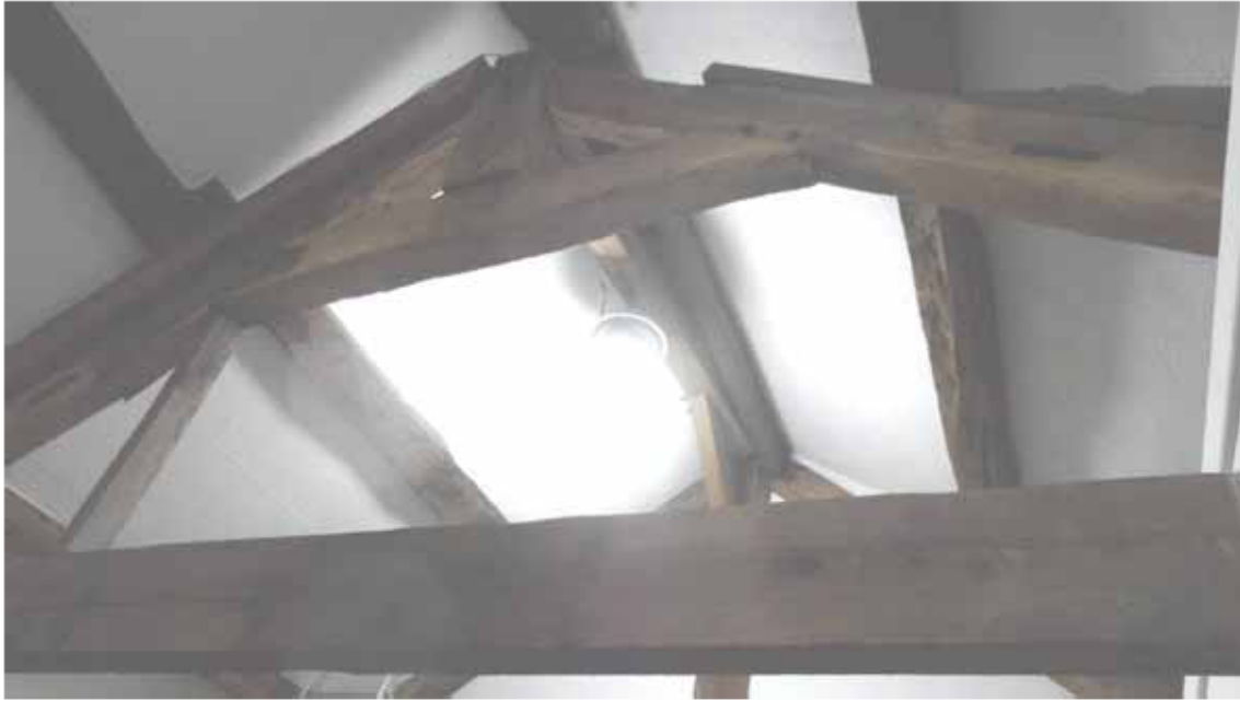
Figure 7: Stables, truss 2 with high collar and modern tiebeam, photograph taken from the east (Alison Arnold)
