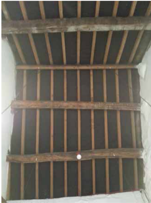
Figure 13: Lobby roof, photograph taken from the north (William Howard)
