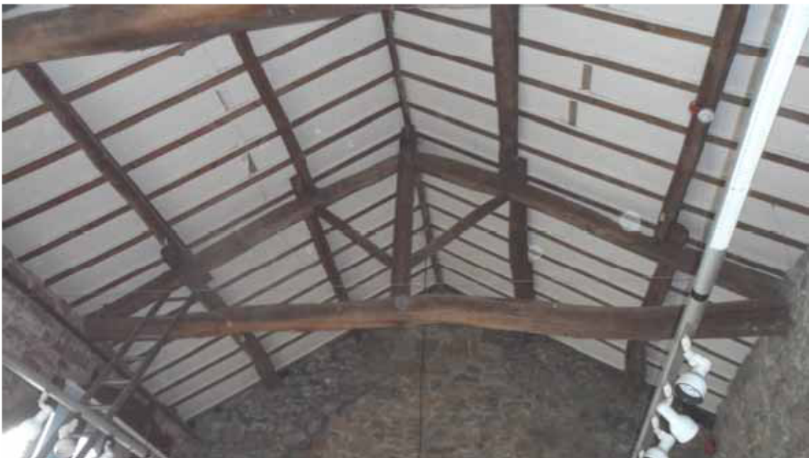
Figure 12: Carriage house, truss 2, photograph taken from the east (Alison Arnold)
