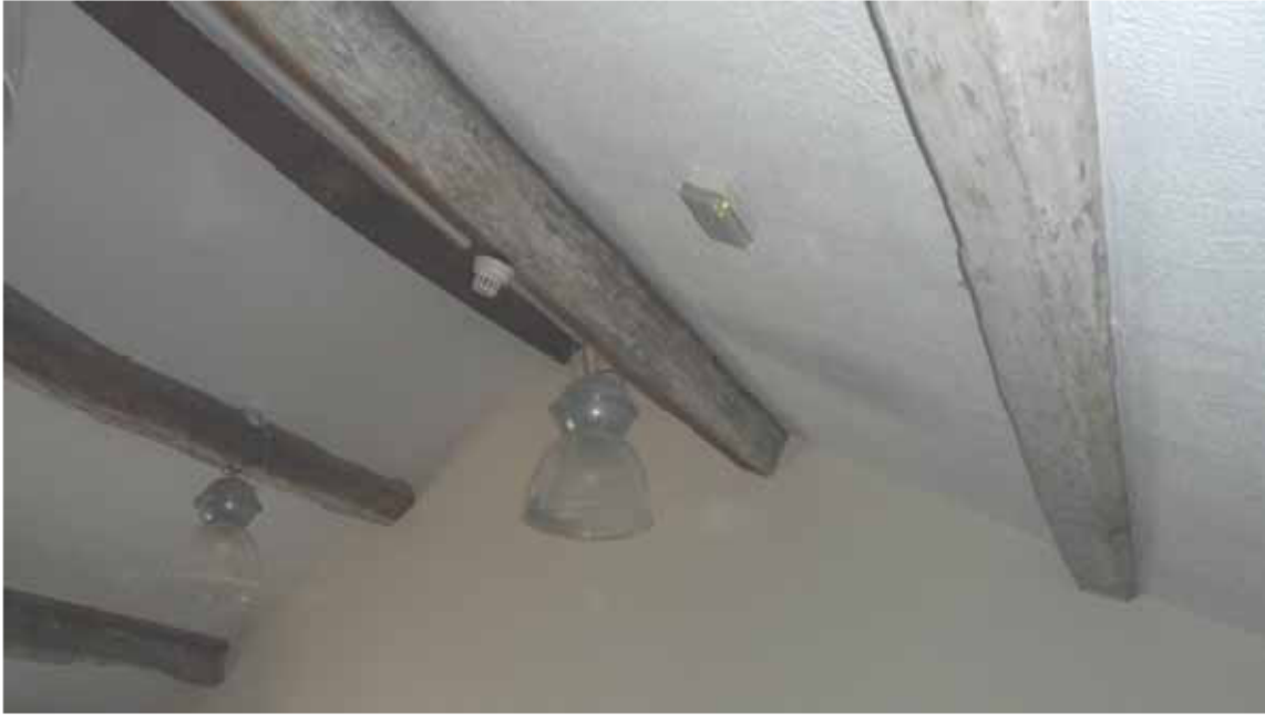
Figure 11: Former bothy roof, photograph taken from the north-east (Alison Arnold)
