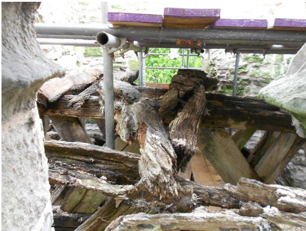
Figure 2: Photograph of the old roof timbers lying on top of the bellframe (Tim Allen)
