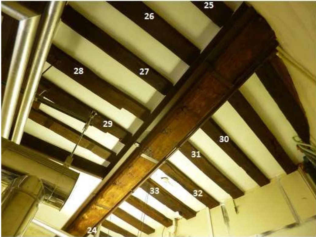
Figure 4e: Annotated photograph of the Porter's Lodge ground-floor ceiling to locate sampled timbers (photograph Robert Howard)
