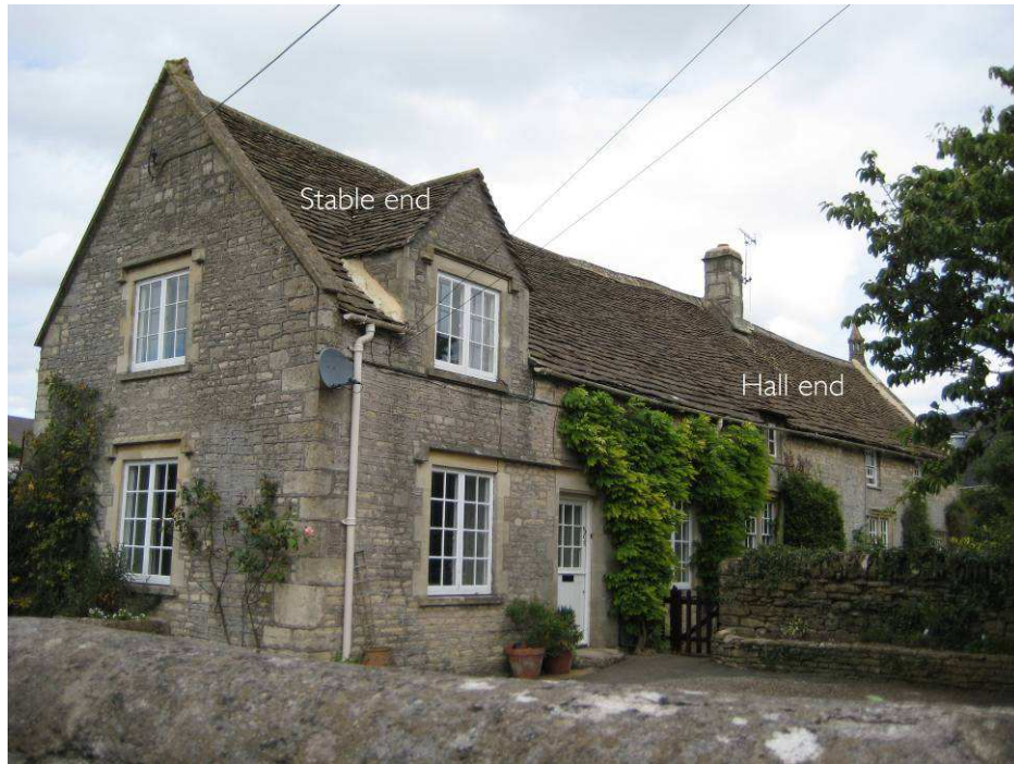
Figure 3: West gable end and south front of Daubeney's (Matt Hurford)
