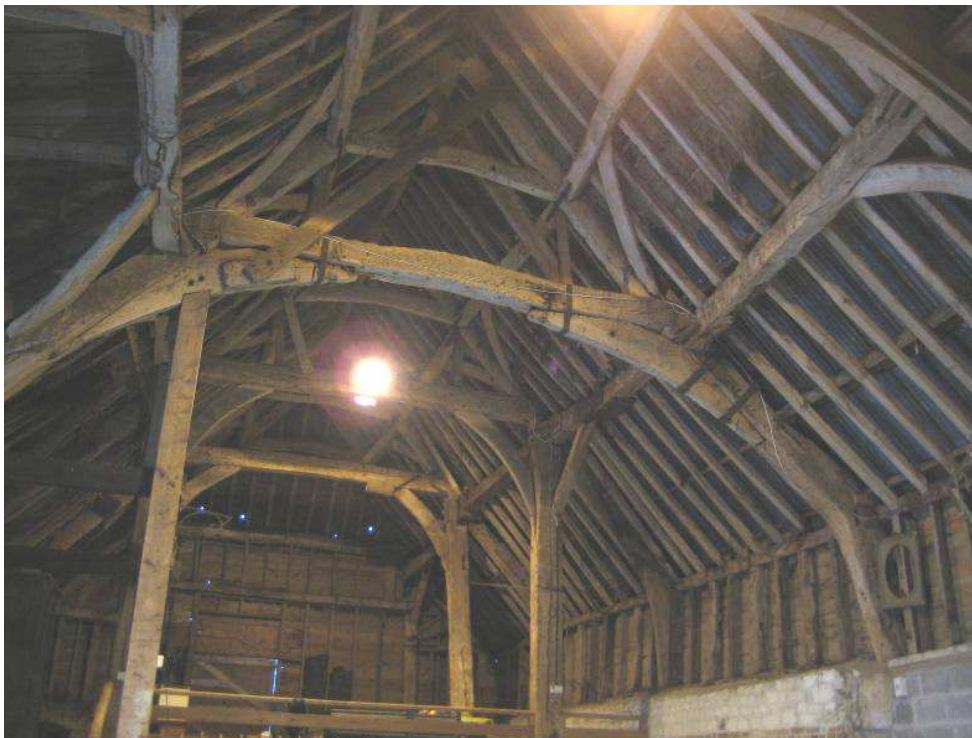
Figure 4: Truss 5 viewed looking south-west (photo Matt Hurford)
