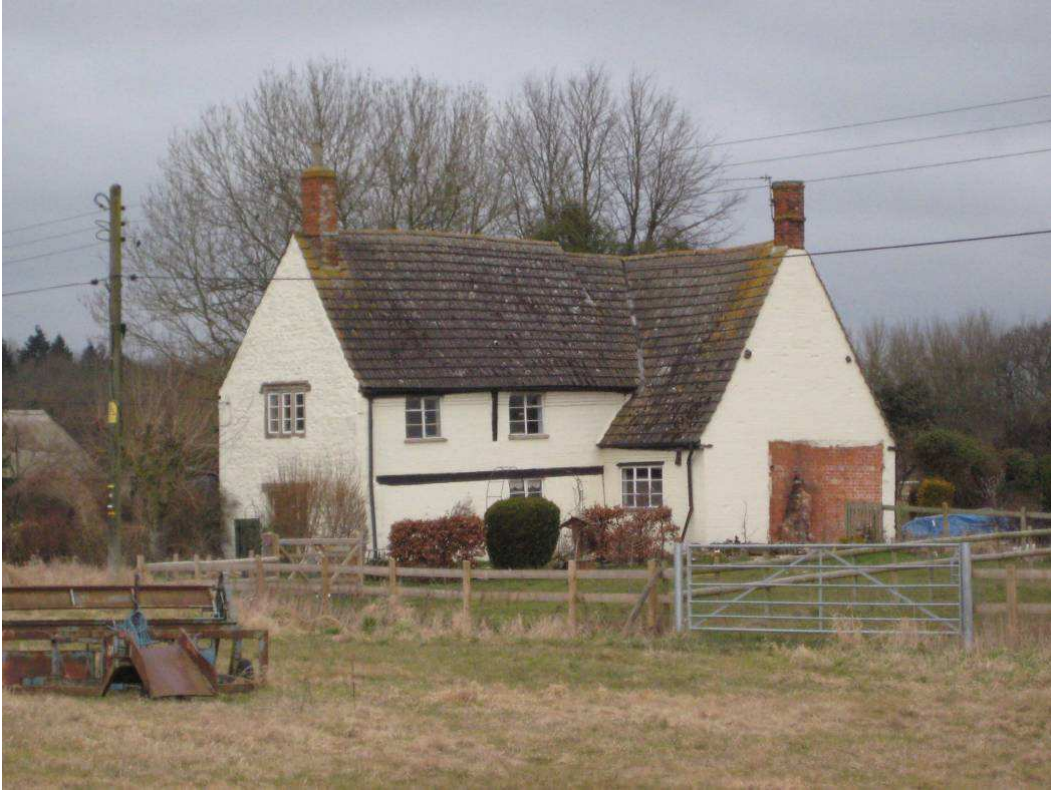
Figure 3: General view of Wick Farm Cottage viewed looking north-west (photo Matt Hurford)
