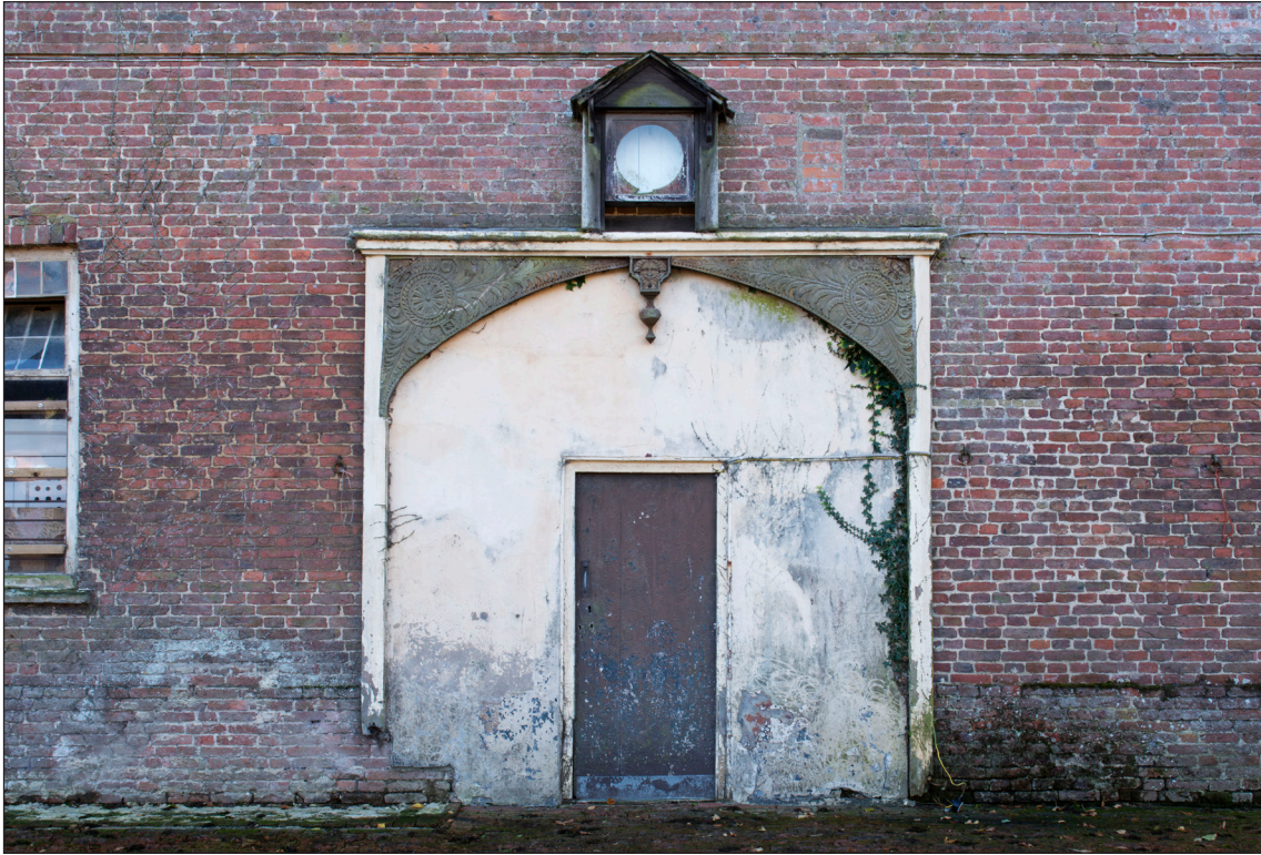
Figure 28: Detail of extant central doorway on the north elevation, showing blocked earlier doorway to the right of the plastered section (DP166147 © Historic England, photograph: James O. Davies).
