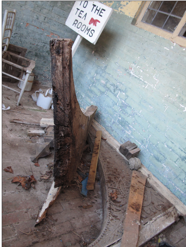
Figure 39: Side of spandrel, showing indications of a sawn off tenon (© Historic England, photograph: Rebecca Lane).
