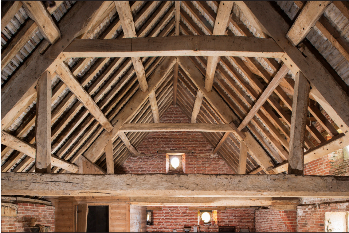
Figure 23: Roof structure looking east (DP166167 © Historic England, photograph: James O. Davies).
