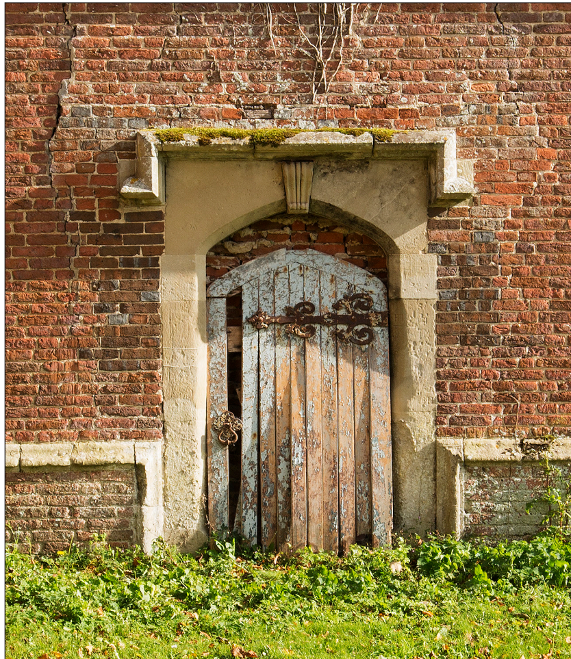
Figure 9: detail of the west doorway, showing poor alignment of the stones of the doorhead with the jambs (DP166171 crop © Historic England, photograph James O. Davies).
