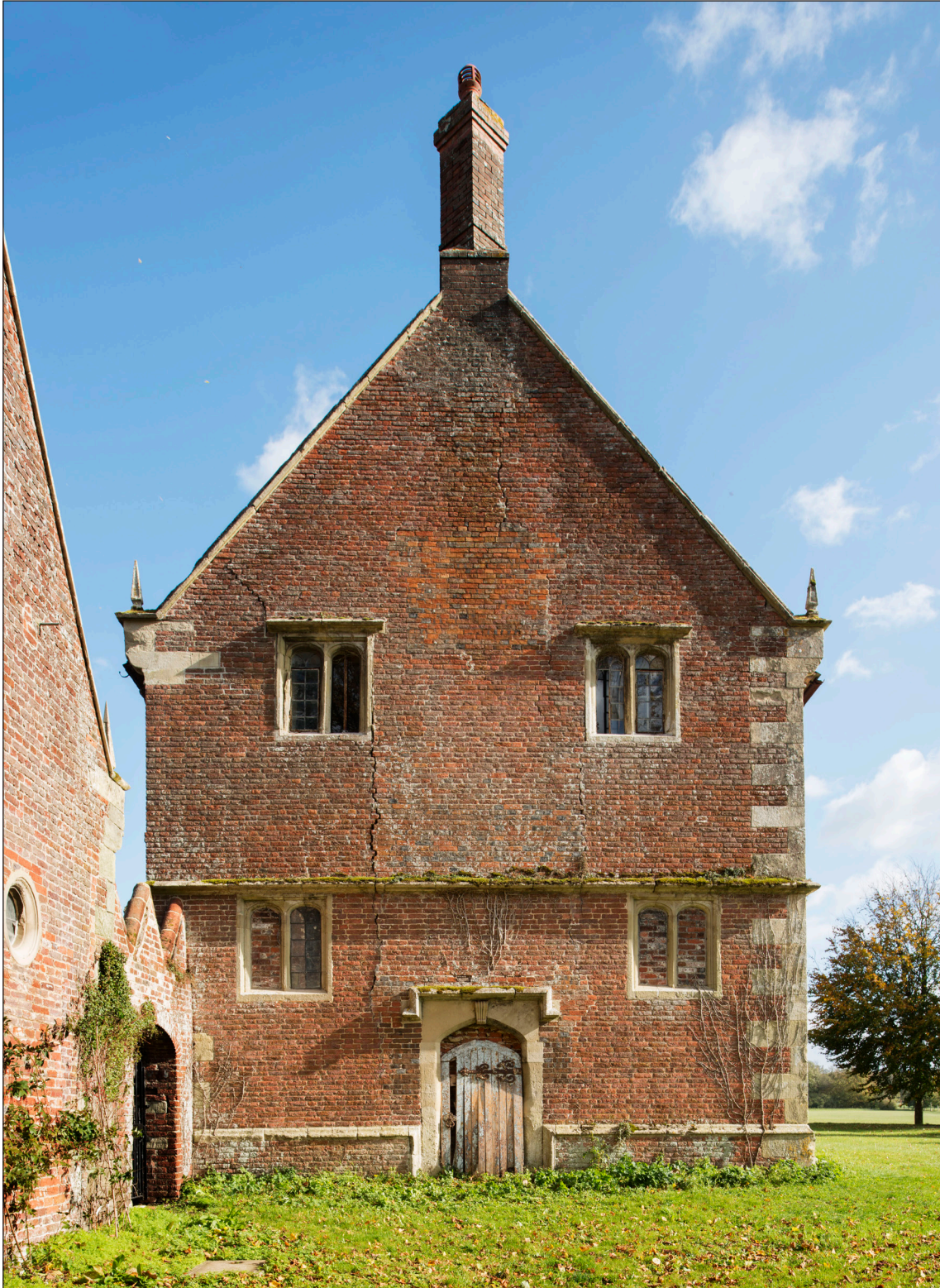
Figure 8: West elevation (DP166171 © Historic England, photograph: James O. Davies).
