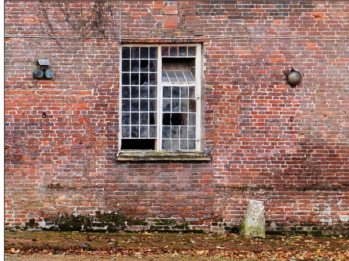
Figure 12: Position of original door opening, indicated by rows of queen closers and infill brickwork (DP166142 crop (c) Historic England, photograph: James O. Davies).
