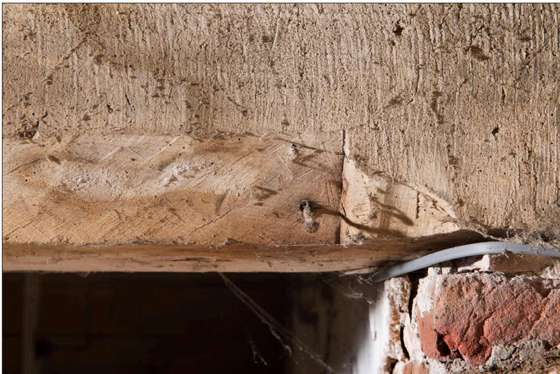
Figure 21: Detail of chamfer stop (DP166178 © Historic England, photograph: James O. Davies).
