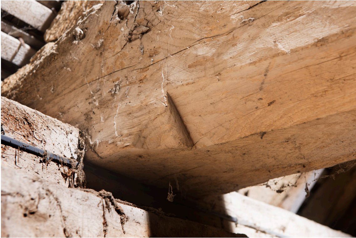
Figure 24: Detail of chamfer stop on tie beam (DP166177 © Historic England, photograph: James O. Davies).
