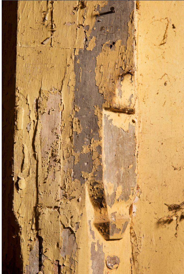
Figure 14: Detail of the chamfer stop on the post (DP166158 © Historic England, photograph: James O. Davies).
