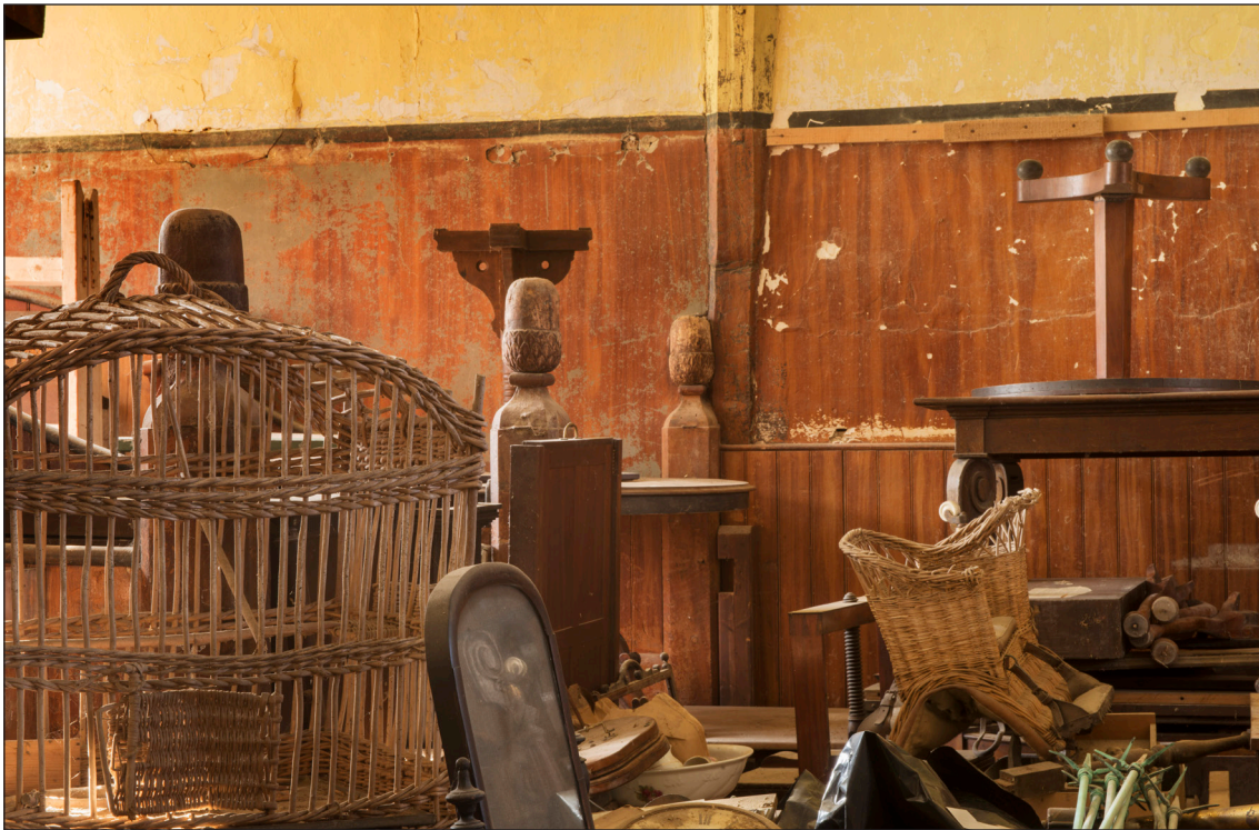
Figure 29: Surviving stalling visible in the east stable, acorn finails marking the end of each bay (DP166187 © Historic England, photograph: James O. Davies).
