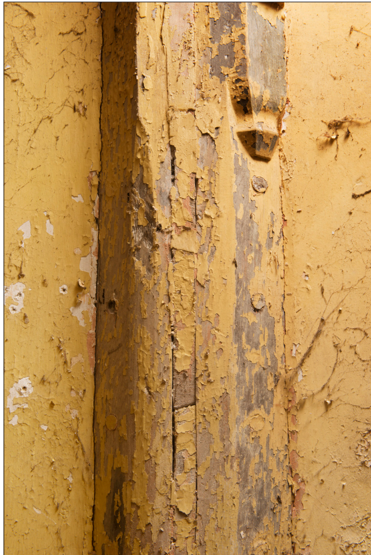
Figure 16: Detail of the upper section of the mortice showing some of the pegs to either side formerly holding it in place (DP166159 © Historic England, photograph James O. Davies).
