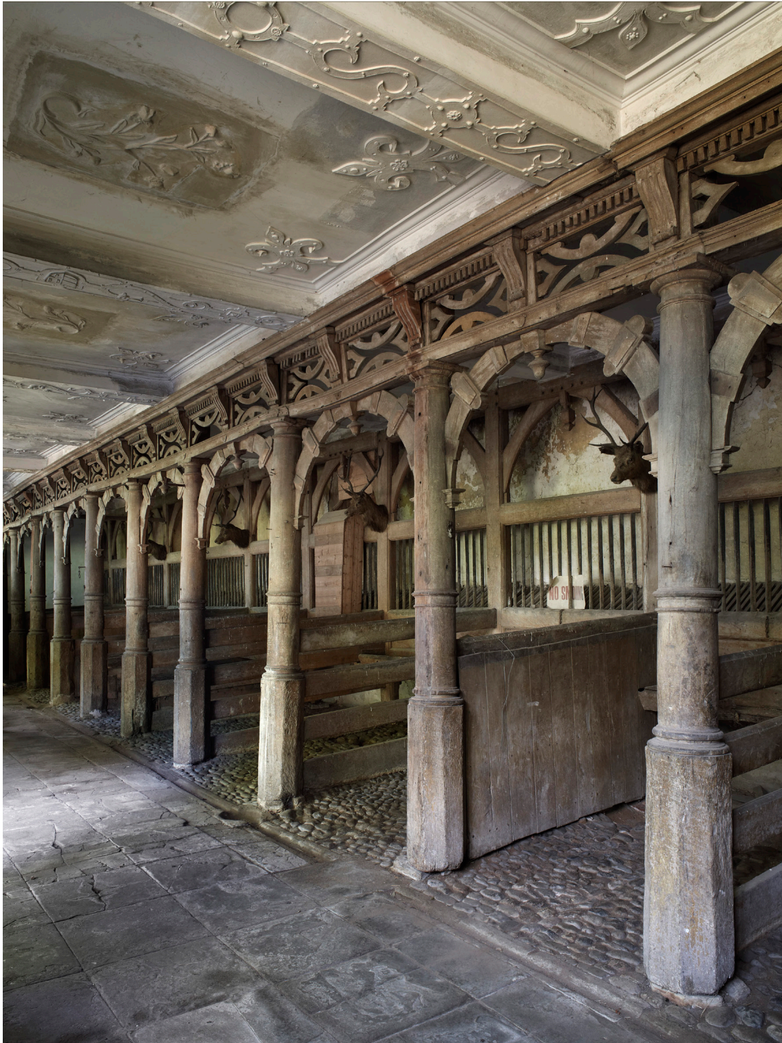
Figure 40: Stable arcade surviving at Peover Hall, Cheshire (Photograph reproduced courtesy of Angelo Hornack).
