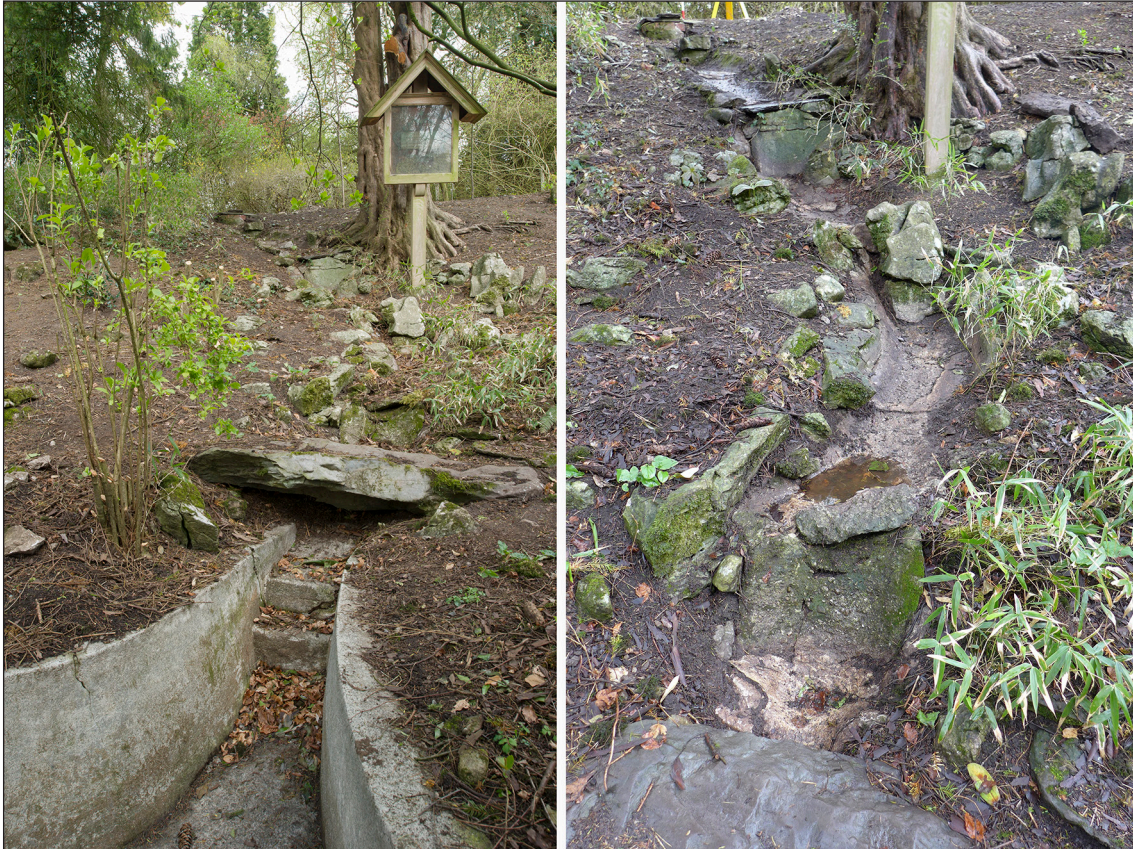
Figure 19: Farrer's 'stream', showing (left) the full cascade from the brick manhole down to the 'block-bridge' at the pond's inlet, and (right) a detail of the central section showing limestone pieces set into the crude concrete channel, looking north-east. © Historic England: (left) DP168959/Alun Bull, 28th April 2015, and (right) Rebecca Pullen, 29th April 2015.
