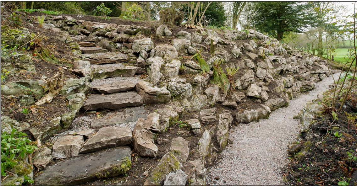
Figure 12: The east steps and the rock face, looking south-east (note the horizontal arrangement of the lowest tier of limestone blocks). DP169007 © Historic England/Alun Bull, 28th April 2015.
