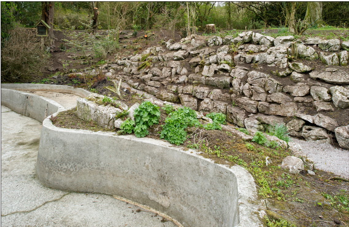
Figure 26: The concrete shelf of the bog garden, with communicating drainage holes (far left), and the rock face beyond, looking north-east. DP168994 © Historic England/Alun Bull, 28th April 2015.
