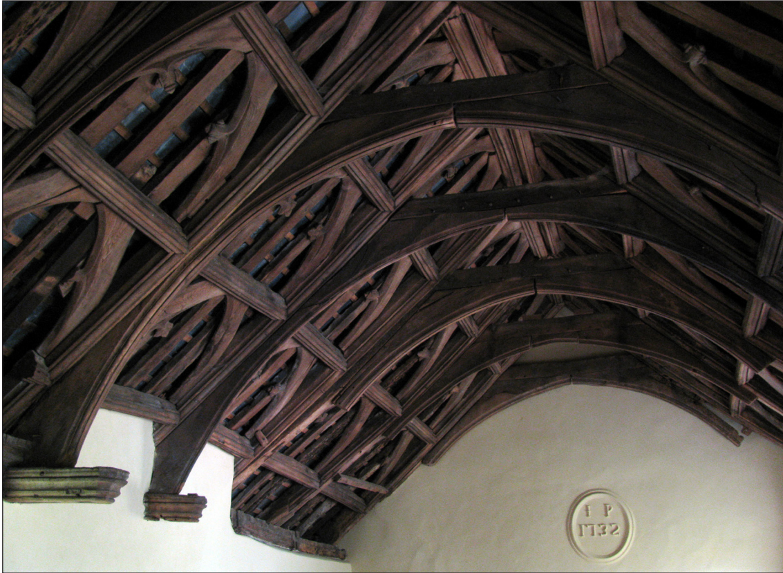
Figure 7: The 15th-century false hammer beam roof at West Challacombe Manor farm house © Historic England, Rebecca Pullen
