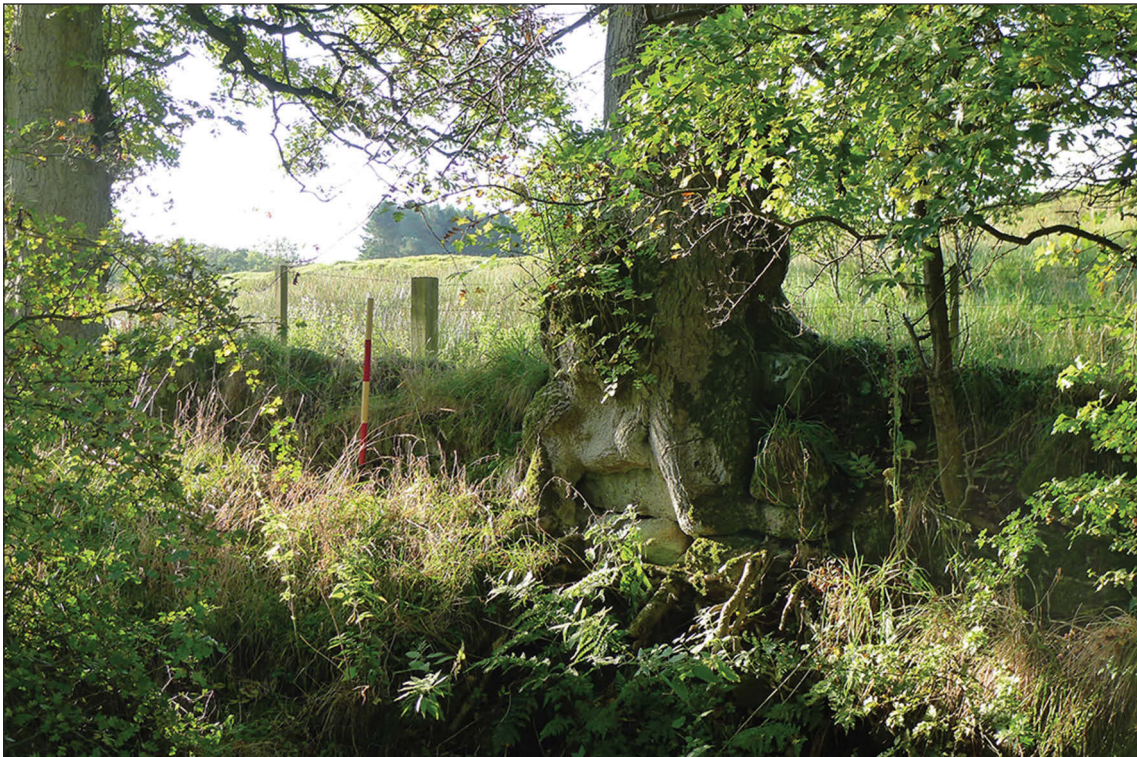
Figure 15. The north-east wall of the bastle viewed across the Linn Kern, showing the top of the boulder plinth and the effects of tree growth, 15 October 2015. © Historic England / David Went.
