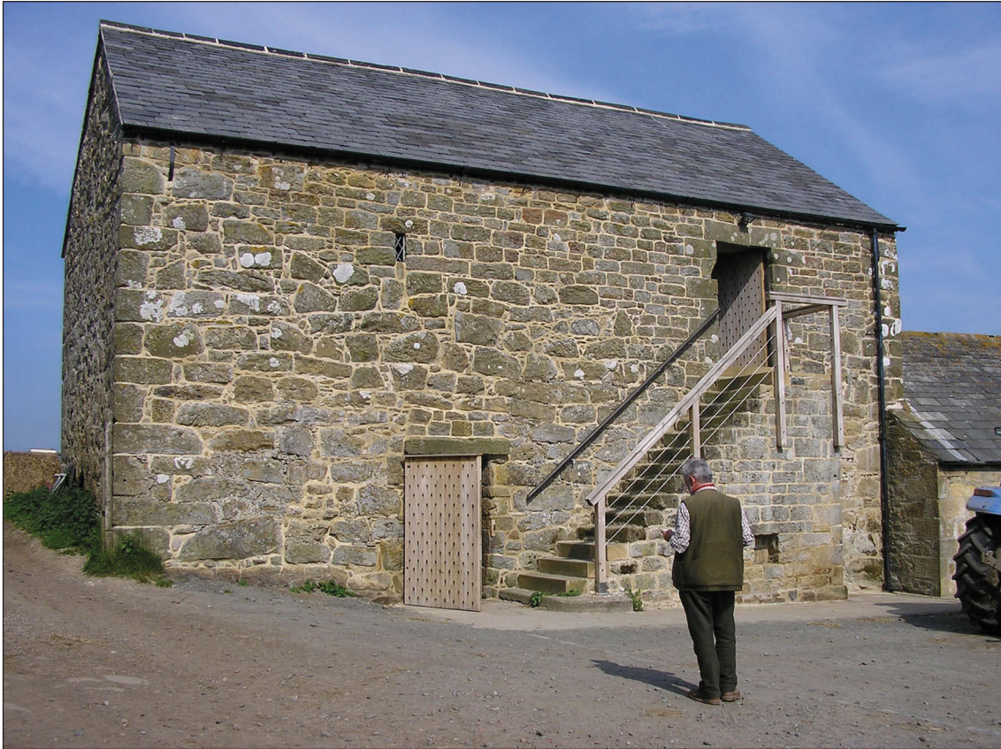
Figure 2. The Raw, Hepple, Northumberland: a fine example of a standing bastle. The lower entrance is modern, replacing the original byre door in the gable wall to the right. An external stairway leads to the upper doorway which would have originally required a ladder. © Historic England.
