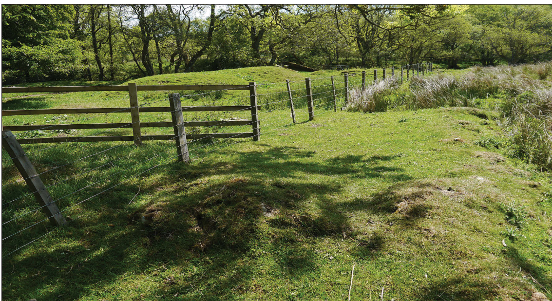
Figure 17. The south east wall of the bastle viewed from within the building's footprint, and the level area extending further south-east which may be a second building or a yard. The large spoil mound [H] is visible beyond. 12 June 2015. © Historic England / Simon Taylor.
