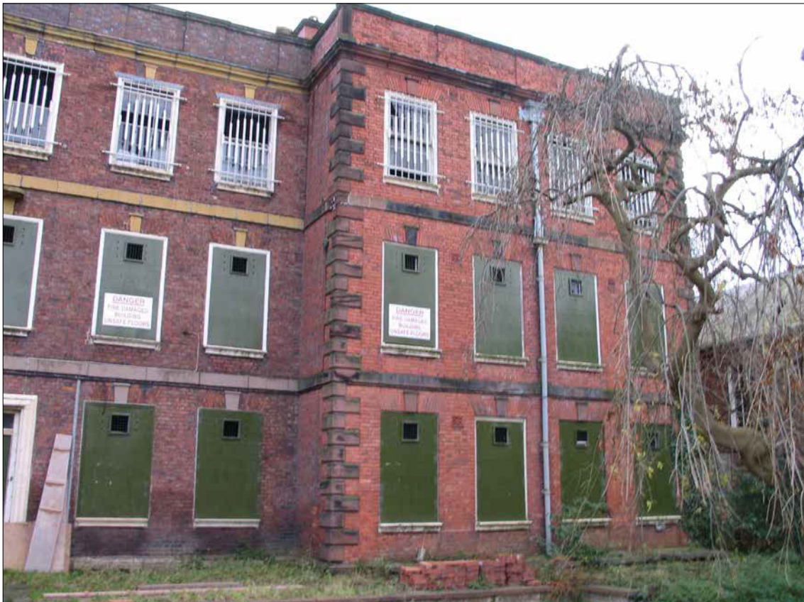
Figure 42: Late-19th-century extension to the west of the original house (© Historic England, photograph: Adam Menuge).
