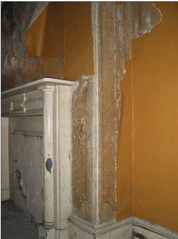
Figure 33: Early-19th-century applied decoration in the drawing room (© Historic England, photograph: Adam Menuge).
