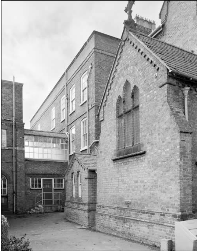
Figure 15: Part of the rear range at Dee House in 1991 (BB91/26351 © Historic England, photograph: Bob Skingle).
