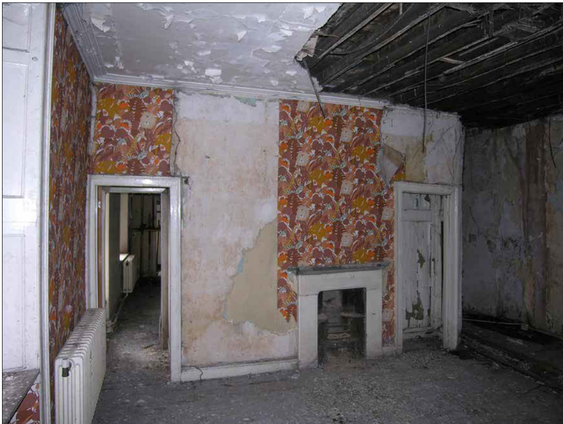
Figure 30: Bedroom 4 on the first floor (© Historic England, photograph: Adam Menuge).
