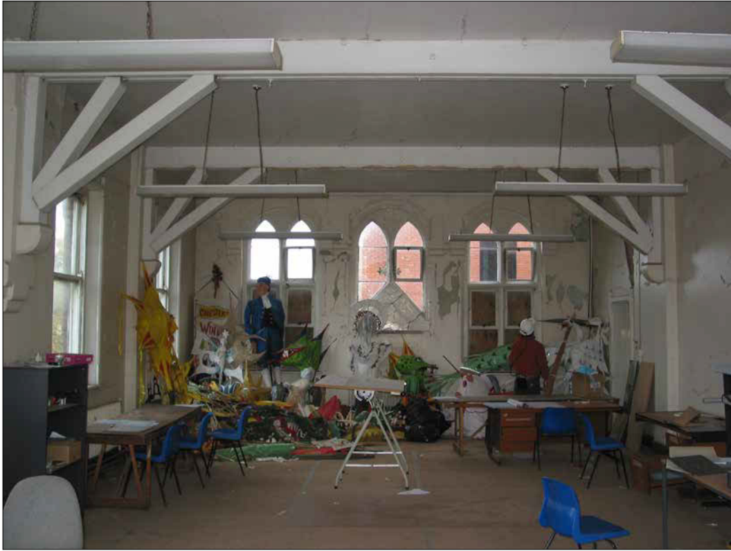
Figure 40: First-floor classroom in chapel-wing extension (© Historic England, photograph: Adam Menuge).
