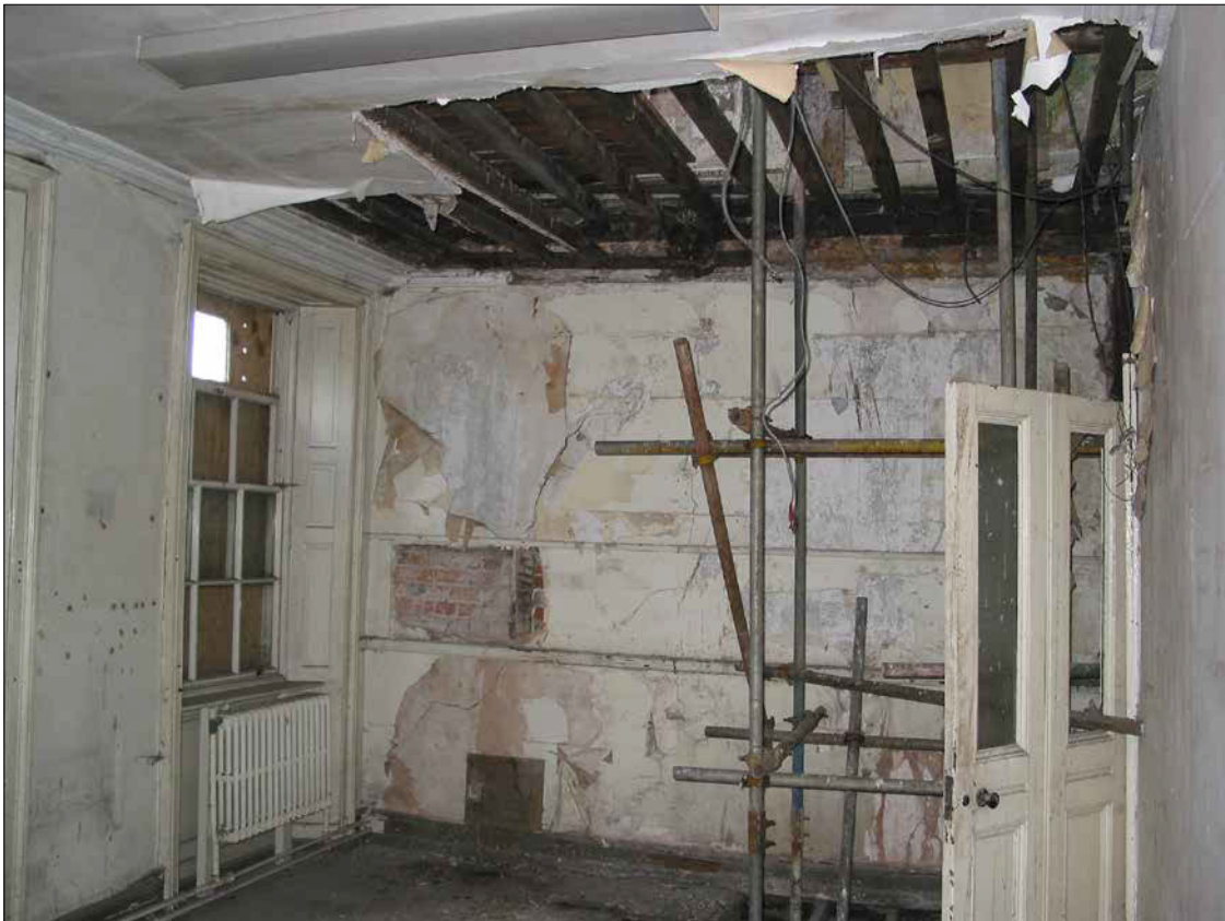
Figure 26: Bedroom 1 on the first floor (© Historic England, photograph: Adam Menuge).
