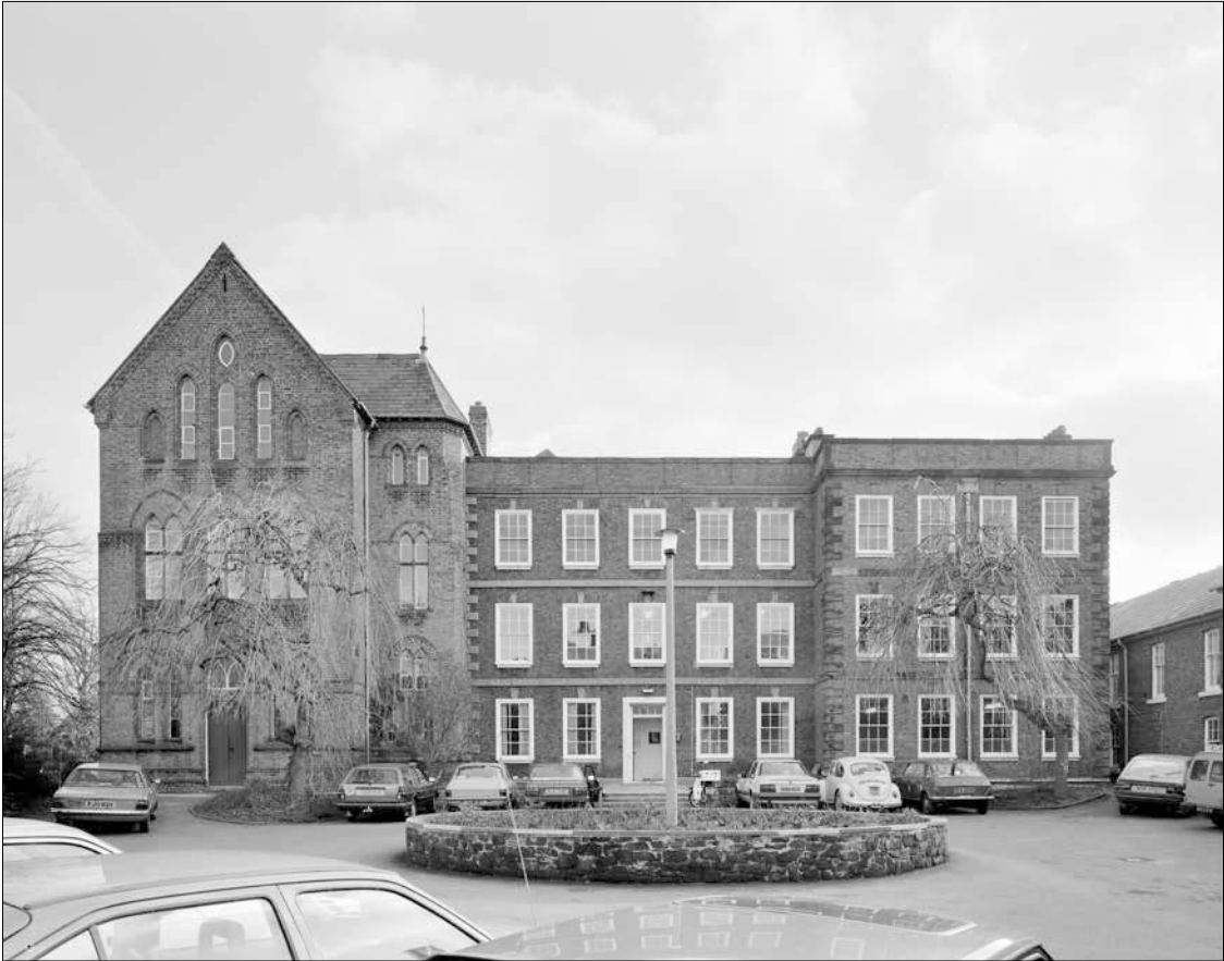
Figure 45: Dee House photographed from the north in 1991 before falling into decay (BB91/26343 © Historic England, photograph: Bob Skingle).
