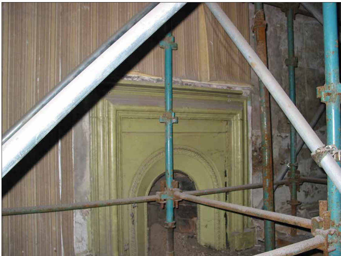
Figure 23: Fireplace in the dining room (© Historic England, photograph: Adam Menuge).
