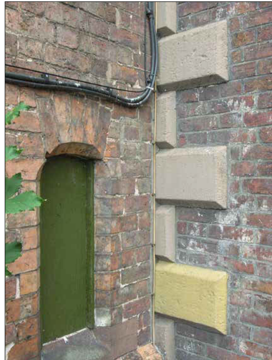
Figure 18: Partially concealed quoins at the north-east corner of the original house (© Historic England, photograph: Adam Menuge).
