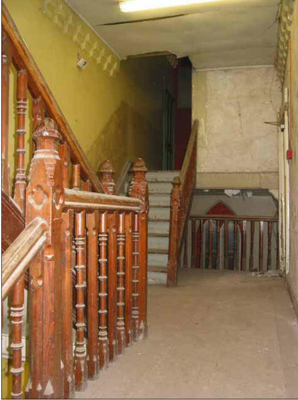
Figure 39: Staircase in chapel-wing extension (© Historic England, photograph: Adam Menuge).
