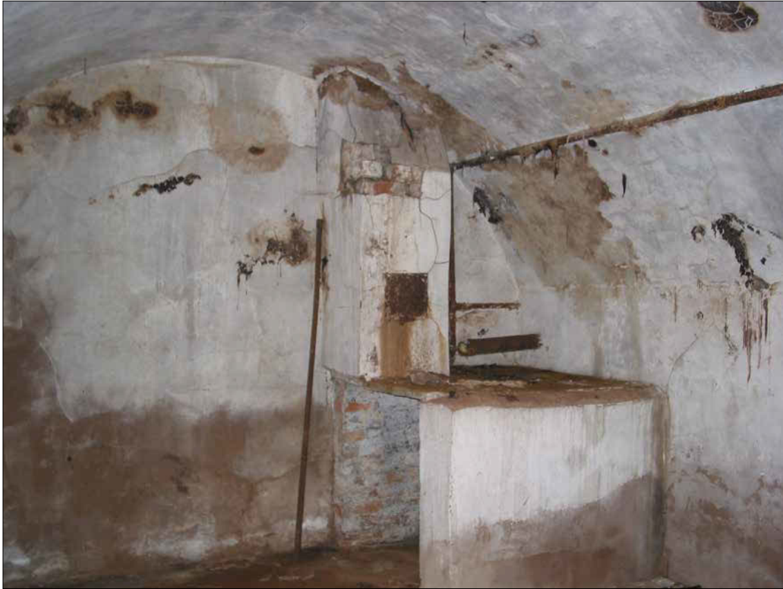
Figure 25: Cellar beneath the original house (© Historic England, photograph: Adam Menuge).
