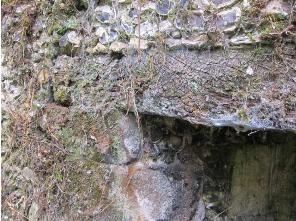
Figure 5: Photograph showing the one of the window lintels (photograph Meriel O'Dowd,)
