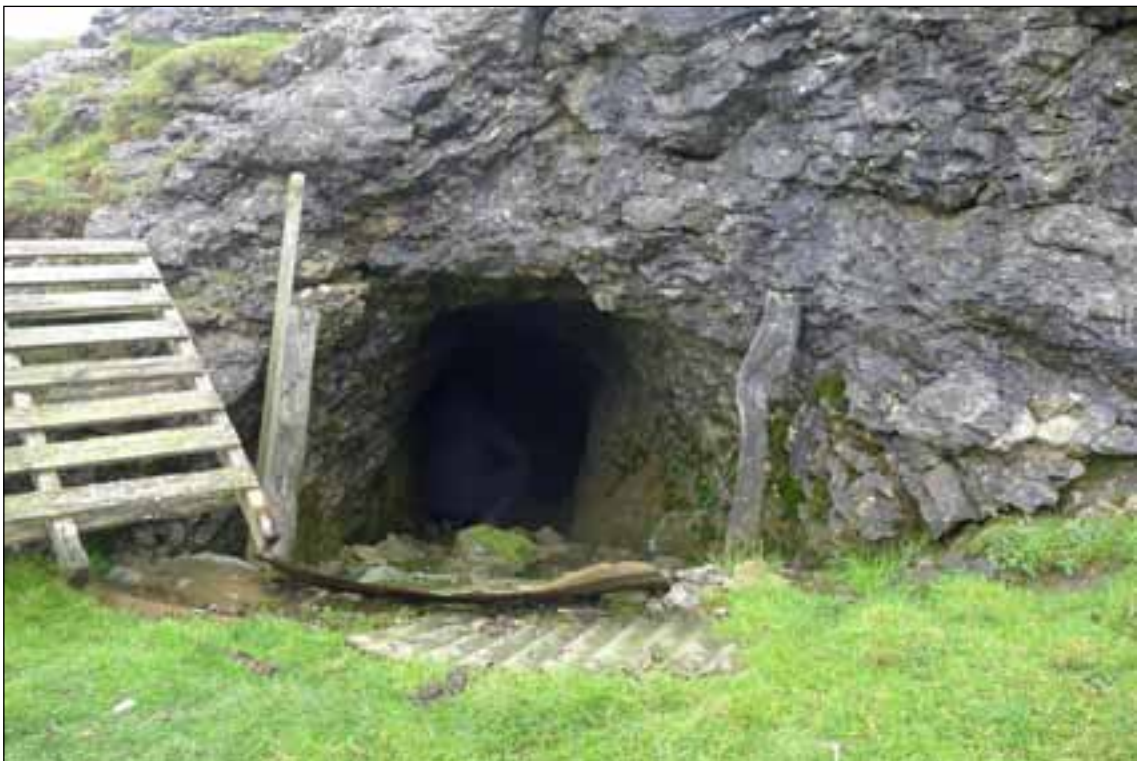
Figure 12: The southern mine entrance (27), and sole surviving point of access to the main levels beneath the knoll. Photo: Rebecca Pullen, © English Heritage.
