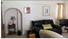
Fig. 54 The north wall of the living/dining room. The arched opening gave access to a closet/larder, and there was formerly a staircase in front of this (see Fig. 40). (© Historic England, K. Morrison)
