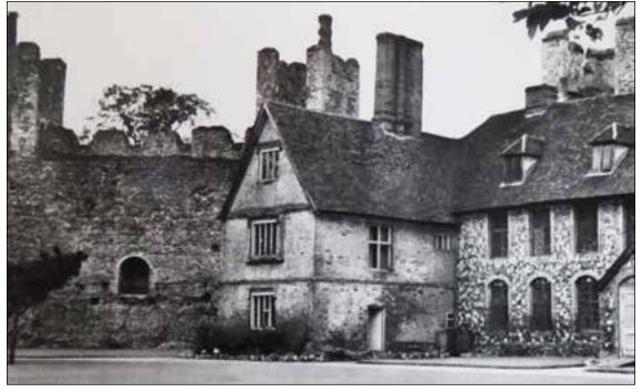
Fig. 50 Detail of a  $20^{th}$ -century postcard, showing the doorway on the north side of the Tea Room. It was replaced with a window in 1955 and the lower part blocked. (Diana Howard)
