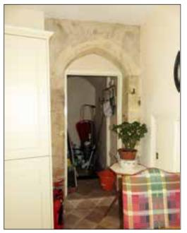
Fig. 55 (left) Doorway within the curtain wall, in the present kitchen (west room). Note the serving hatch just visible to the right (see also Fig. 23). (© Historic England, K. Morrison)
