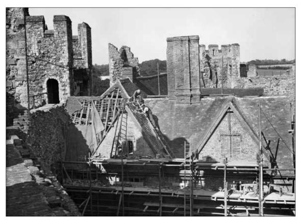
Fig. 37 Repairs to the roof of the Red House, 12 September 1933. (© Historic England Archive, OWS01/02/F01172)
