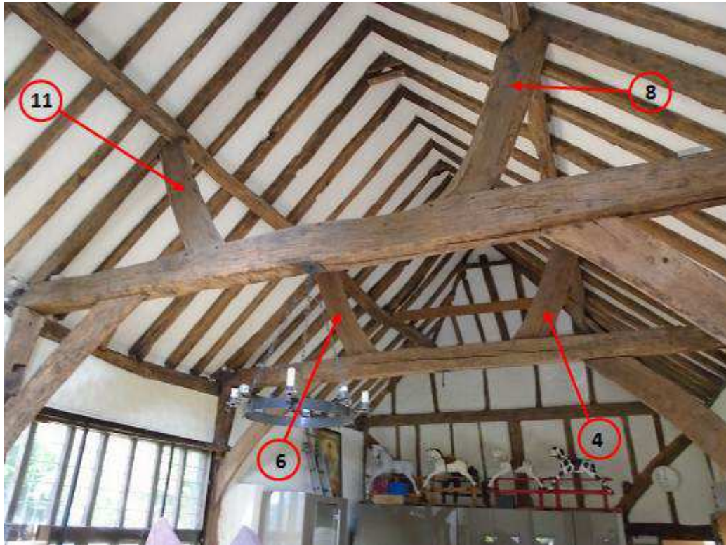
Figure 4c: Annotated photograph to help locate sampled timbers (photograph Robert Howard)
