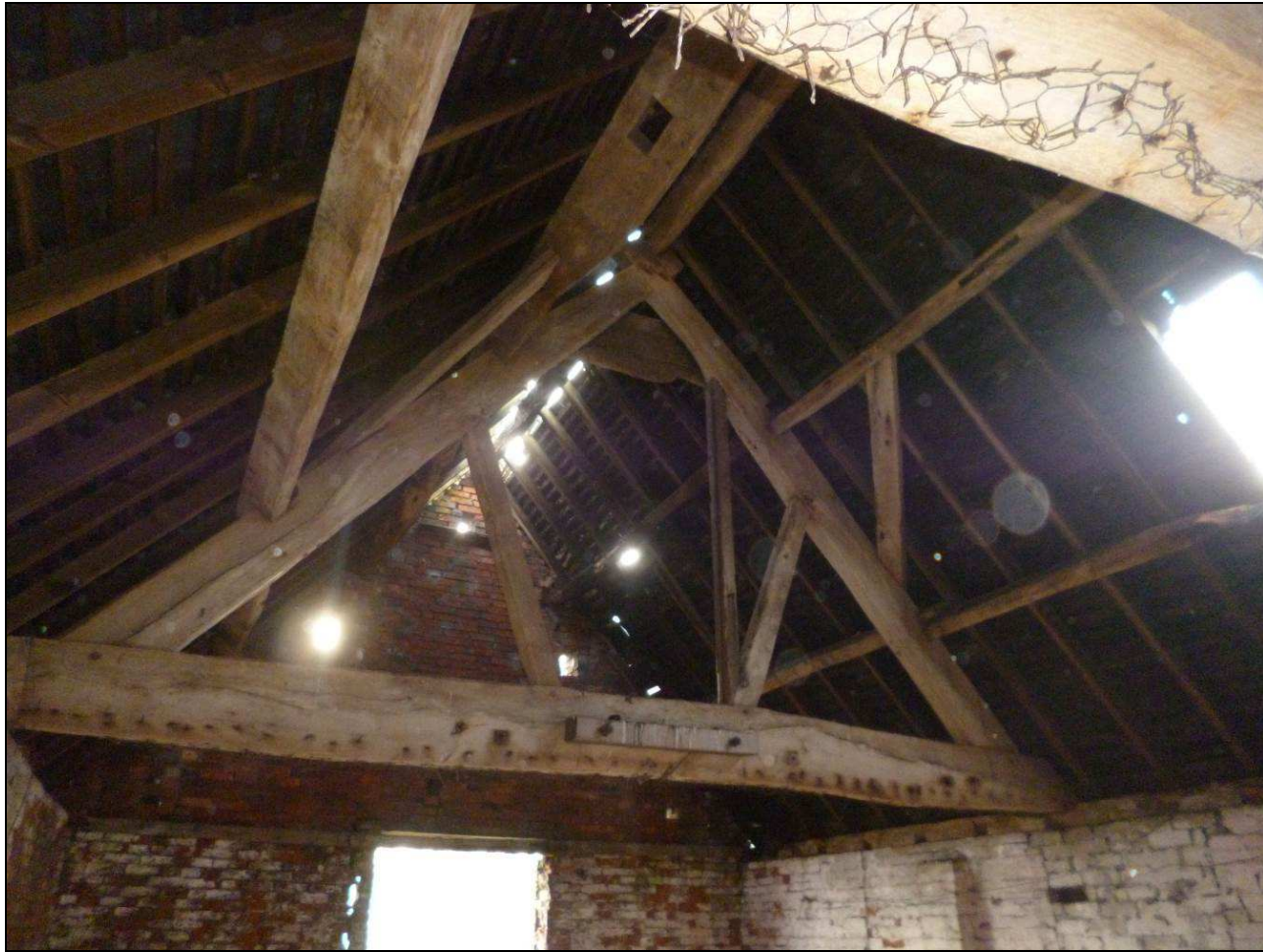
Figure 9: Barn, truss 2, photograph taken from the north (Robert Howard)
