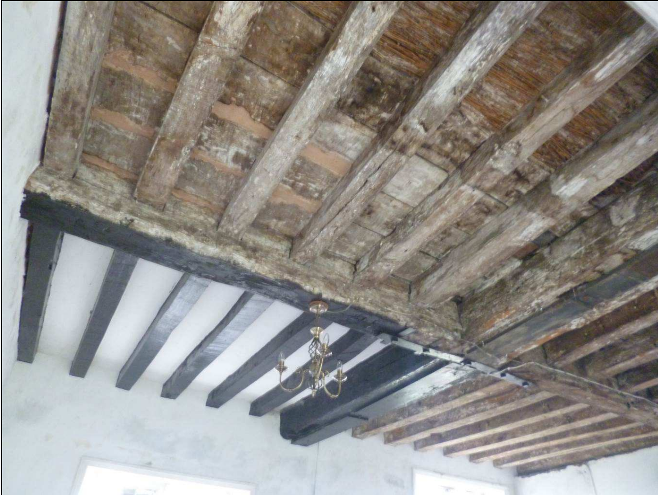
Figure 8: Farmhouse, southern extension floor frame (left of photograph), photograph taken from the south-east (Robert Howard)
