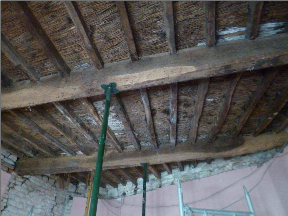
Figure 8: South-east tower ceiling, photograph taken from the south (Alison Arnold)
