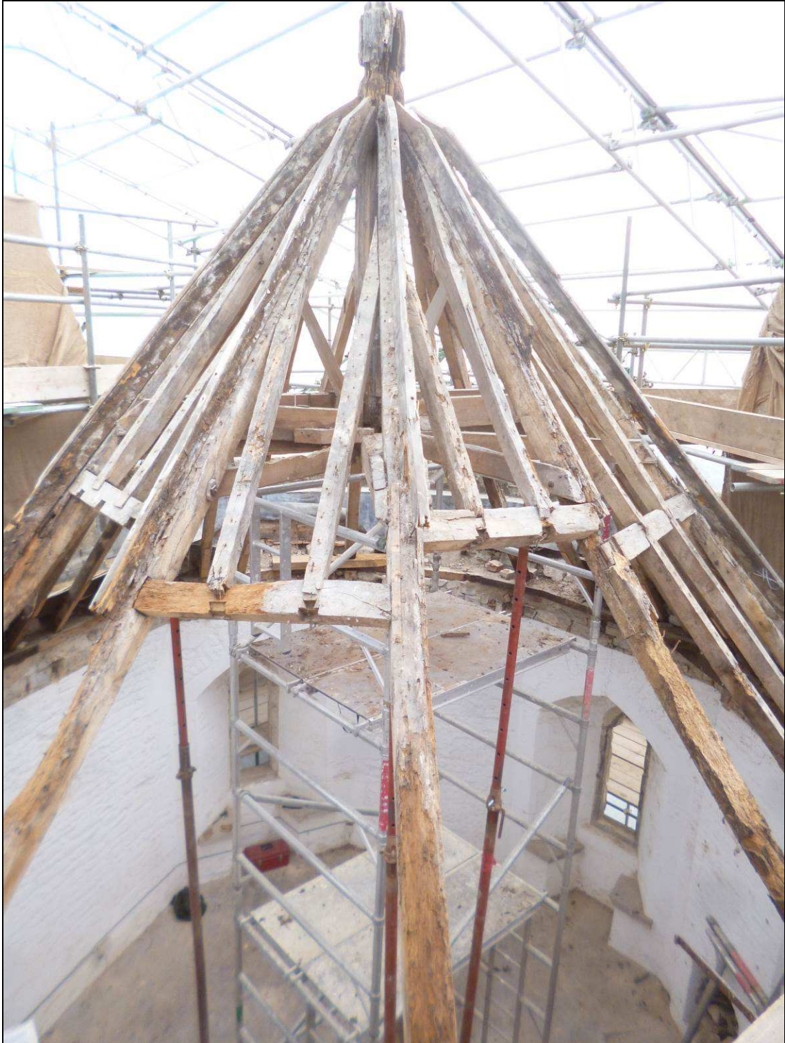
Figure 7: South-east tower roof, photograph taken from the north-west (Alison Arnold)
