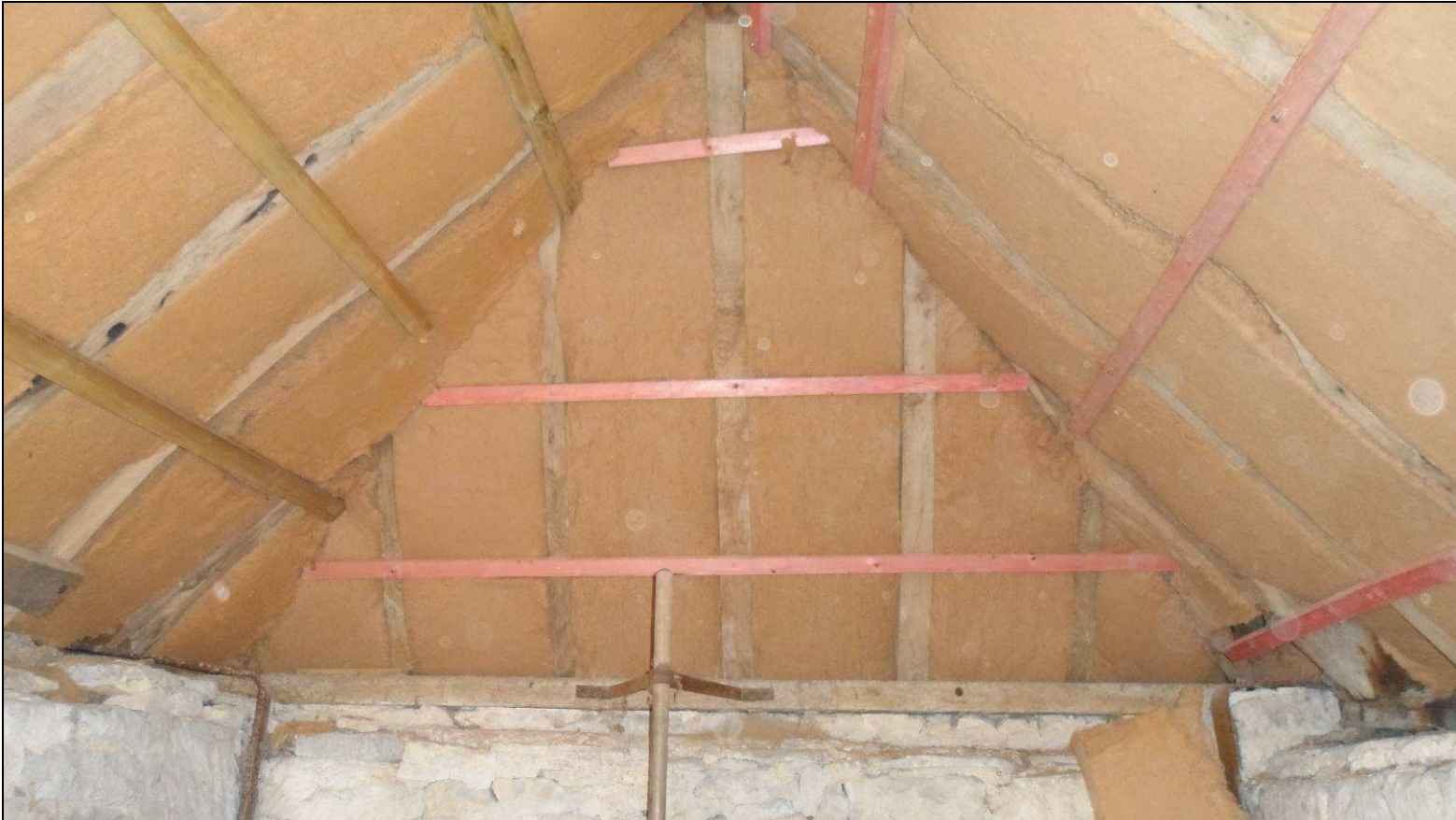
Figure 9: Garderobe roof, photograph taken from the north (Alison Arnold)
