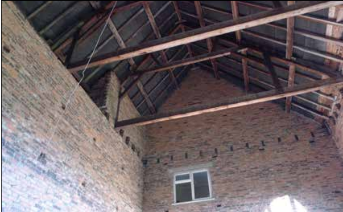
Figure 26: Roof trusses and evidence of possible loft (© Historic England, photograph taken by Lucy Jessop)
