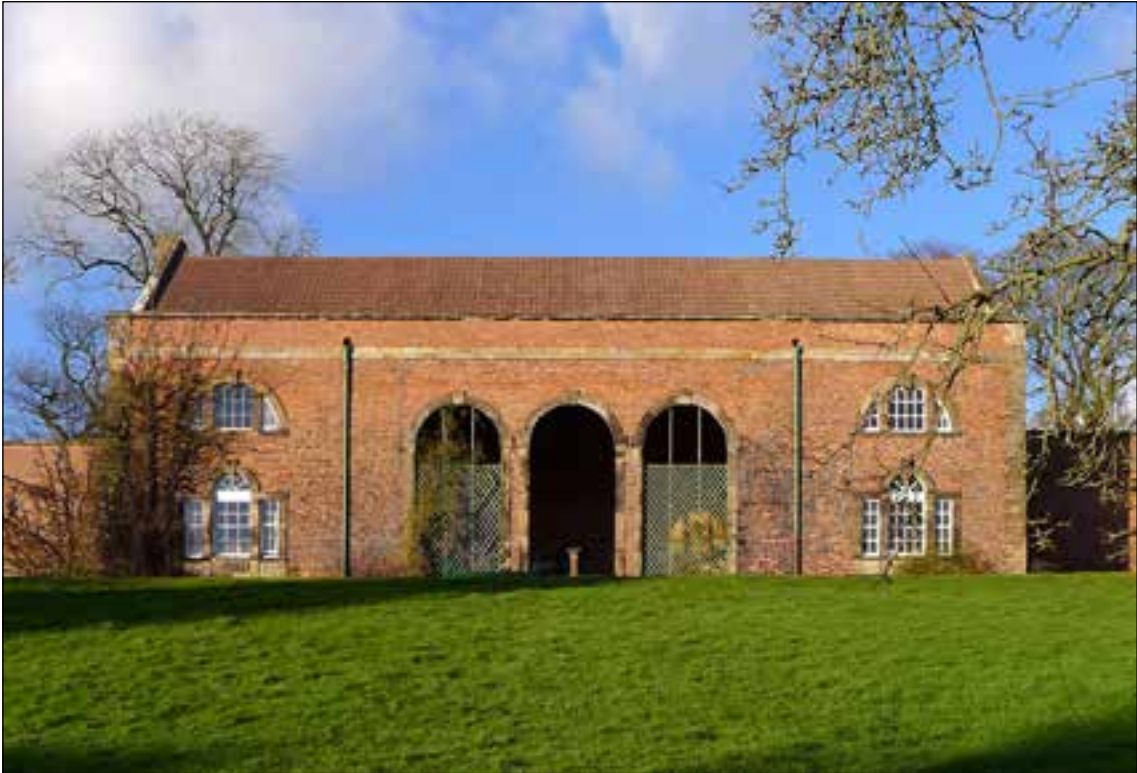
Figure 24: The pavilion from the south (© Historic England, photograph taken by Lucy Jessop)
