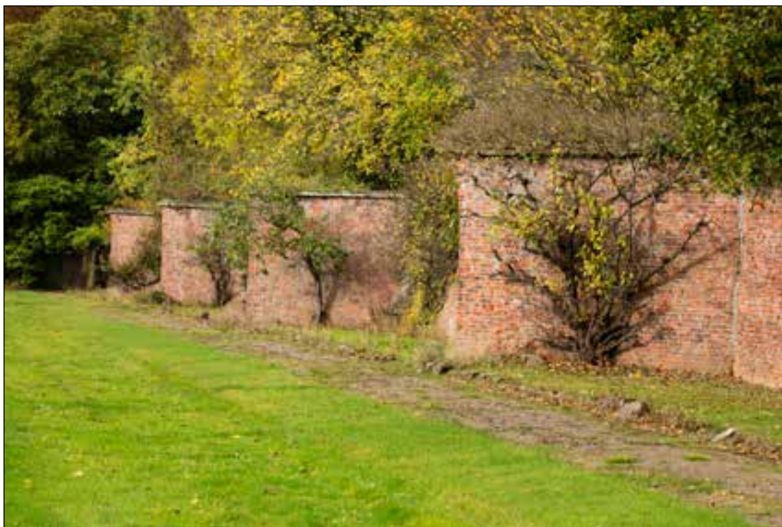
Figure 18: Triangular projections along western part of wall (DPI174229 © Historic England, photograph taken by Alun Bull)
