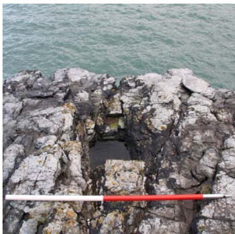
Figs 20 and 21: rock-cut holes for timbers at the outer corners of the Iron Gate quay
