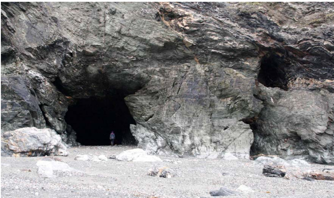
Fig 27: the mine adit to the right with the scar of the walkway passing across the top of Merlin's Cave to the left
