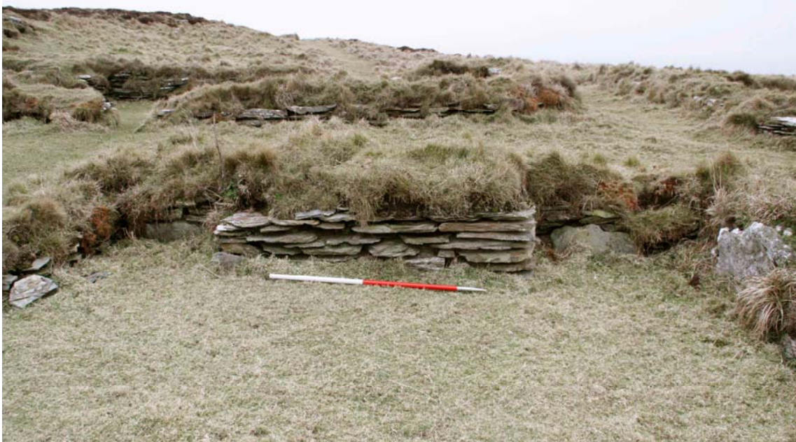
Fig 10: interior of building 032 showing the unexplained 're-constructed' structure against the west wall; buildings 029 and 030 lie beyond
