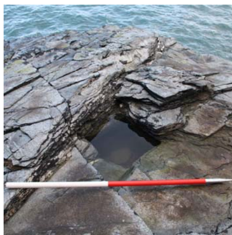
Figs 20 and 21: rock-cut holes for timbers at the outer corners of the Iron Gate quay
