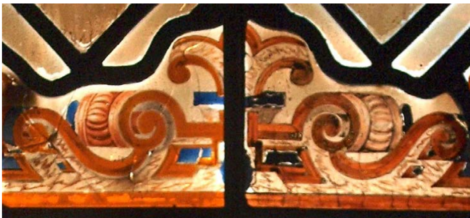
Figure 19. Window F8L1, panes P5 (right) and P8 (left) showing the later repair on the right executed using black rather than blue enamel
