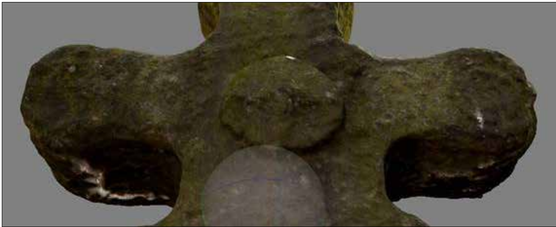
Figure 13: SFM model of the market cross. Note the uneven texture of the undersides of the cross arms, and also a rather pixelated area on the right cross arm, from a lack of photos and high resolution imagery.
