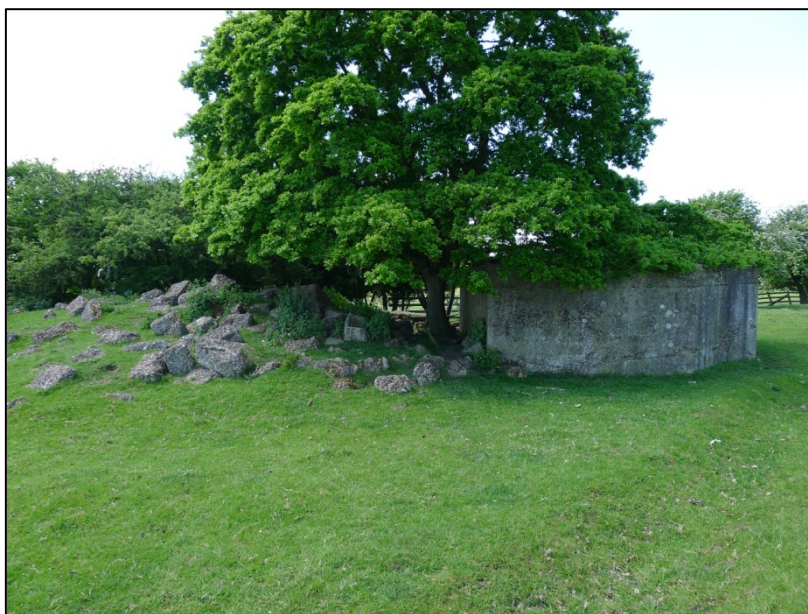
Figure 25 NRHE 1426123 Type 24 pillbox (No. 6 in Fig 22 and the table below) with adjacent rubble, possibly from a demolished pillbox. Photographed in May 2015.
