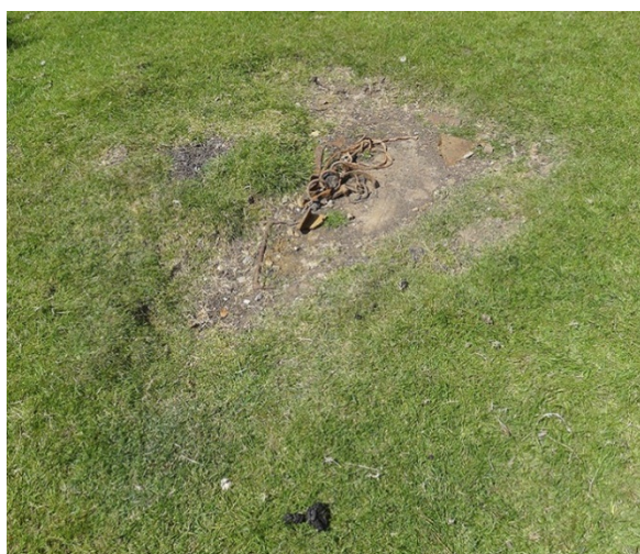
Figure 32 NRHE 1549853 Buried hatch seen on a field visit in May 2015. It is probably associated with military earthworks on the north edge of Deangate Ridge (No. 2A in table above).
