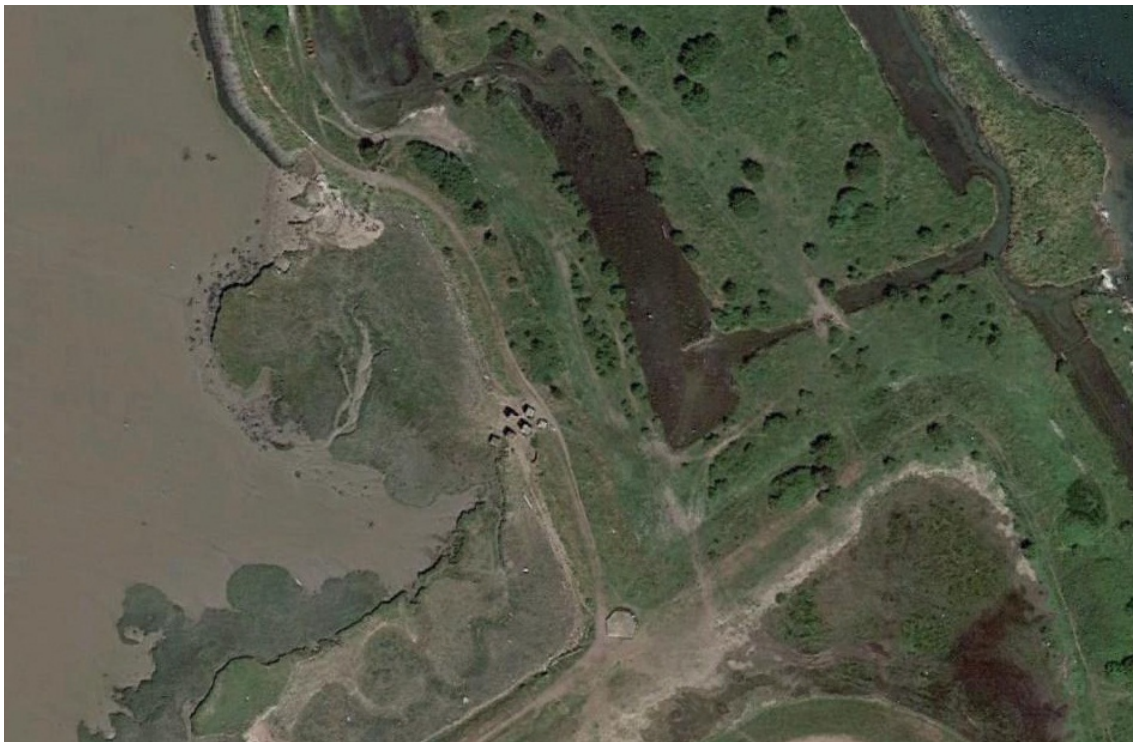
Figure 46 The remains of the anti-tank ditch, concrete pillars and pillbox on the bank of the River Thames © Google Earth 07-SEP-2013
