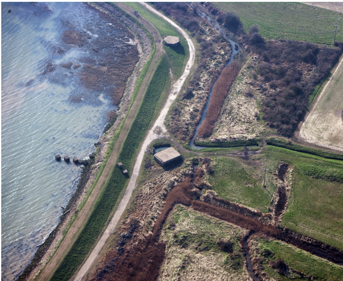
Figure 7 Anti-tank cubes and pillboxes at the southern end of the stop line on the river Medway to the south east of Hoo St Werburgh. NMR 26887_047 08-MAR-2011
