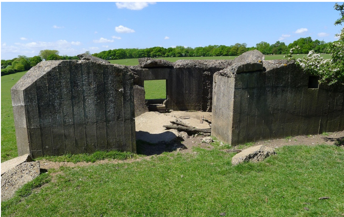
Figure 31 NHE I426099 Type 28 pillbox (No. 5 in the table above) surviving as a roofless structure photographed in May 2015. A gun emplacement is located within the embrasure in the centre of the photograph.
