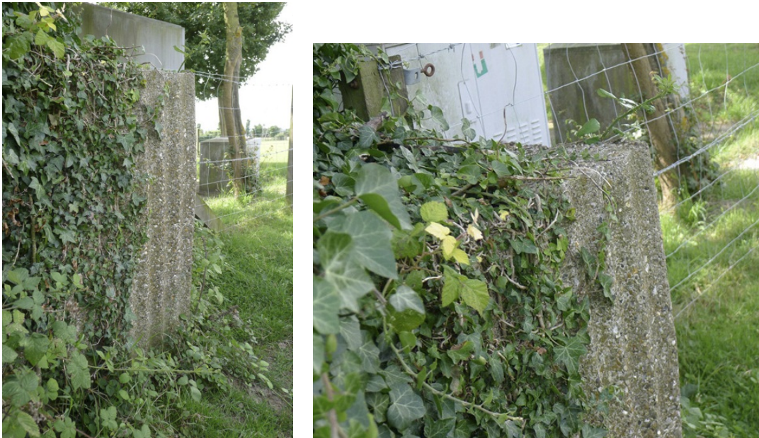
Figure 5 Concrete blocks which were part of a roadblock on a track leading north from Stoke Road, Hoo St Werburgh (NRHE 1418717)
