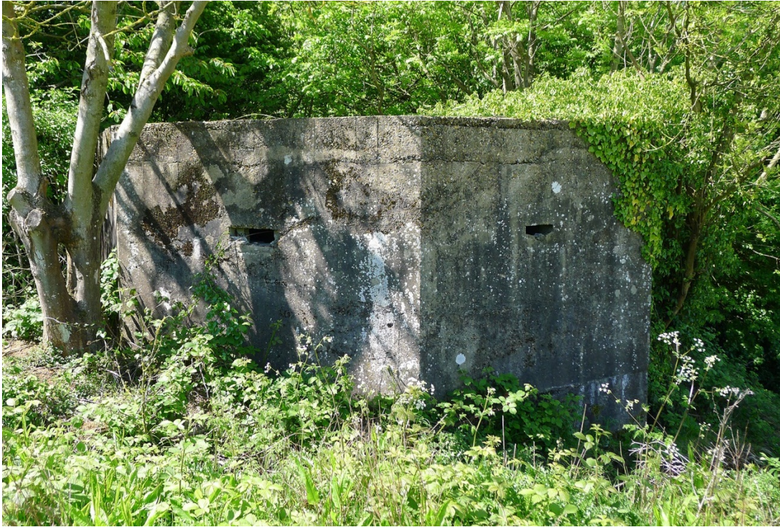
Figure 30 NRHE I426724 Type 24 pillbox (No. 2 in the table above) with blocked embrasures, photographed in May 2015.
