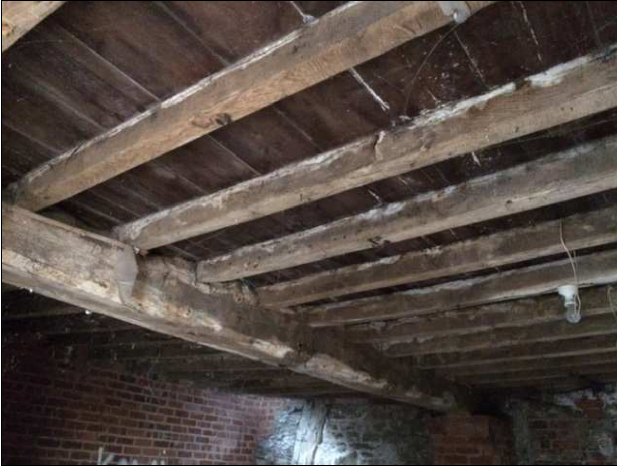
Figure 7: Floor frame in bay 1, photograph taken from the south-east (Alison Arnold):
