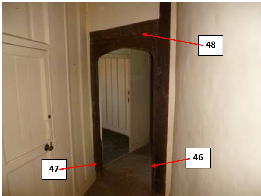
Figure 4h-i: Photographs to help locate sampled timbers of the first-floor doorway 1 (top) and 2 (bottom) (photographs Robert Howard)
