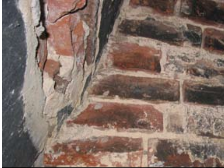
Figure 17.1 Looking up - the brick built flue.
