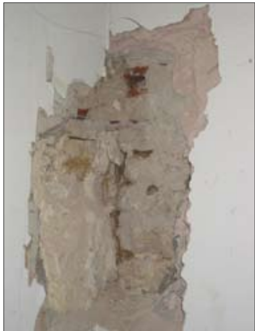
Figure 14.2 Slate damp-course. Taken from the north east.
