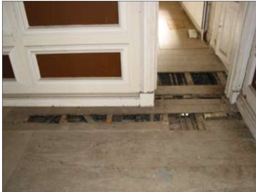
Figure 31.1 Floor structure leading from H2.12 to H2.10 Taken from the south.
