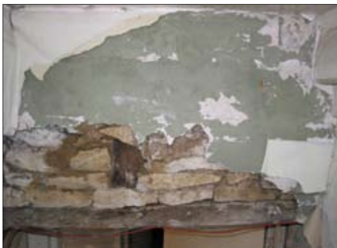
Figure 41.2 Coursed rubble walling above doorway to Cock Loft stairway, showing the incorporation of floor joists from the room above.
