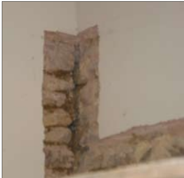
Figure 9.1 Straight joint between two walls. Taken from the south.
