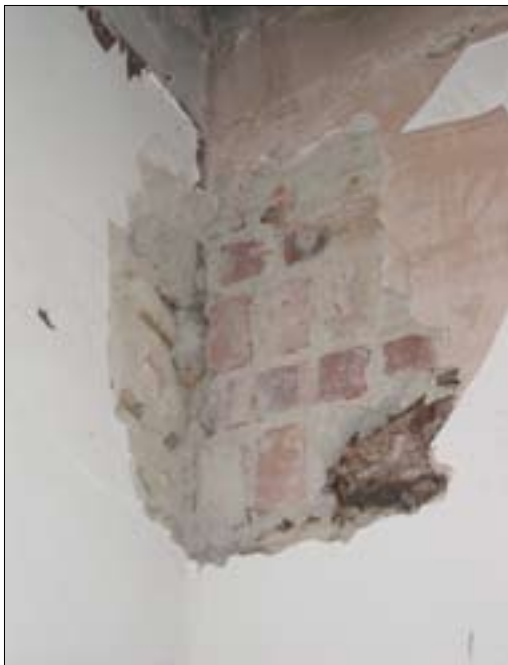
Figure 14.1 Straight join between stone and brick wall. Taken from the north east.
