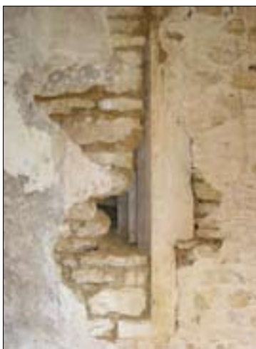
Figure 33.1 Blocked window. Taken from the north.
