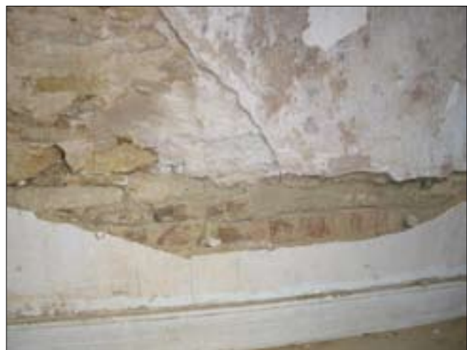
Figure 33.2 Brick underpinning. Taken from the north.
