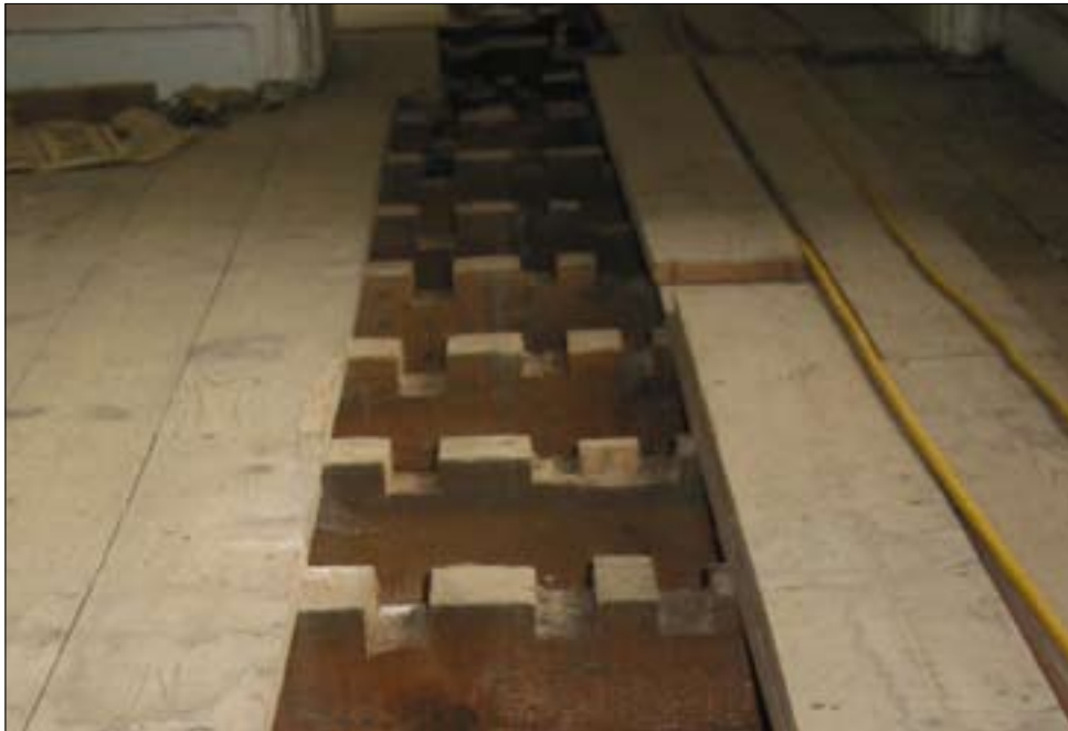
Figure 21.1 Floor structure. Taken from the west.
