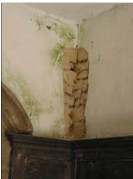
Figure 6.1 North-west corner of east porch.
