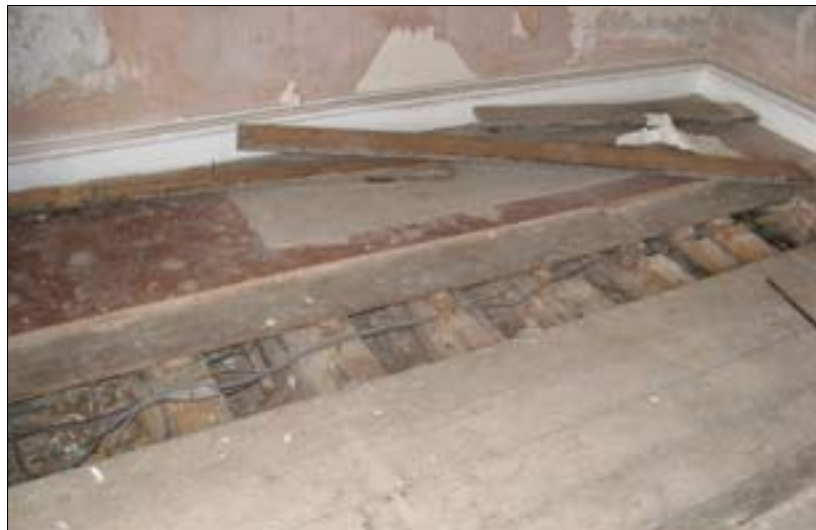
Figure 35.1 Floor structure. Taken from the east.
