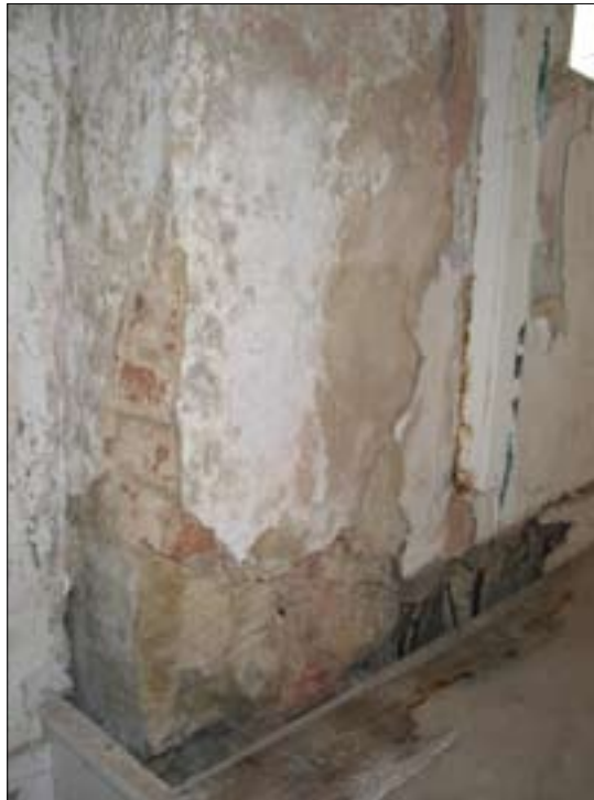
Figure 30.1 Ashlar quoin with red brick modifications. Taken from the south-east.
