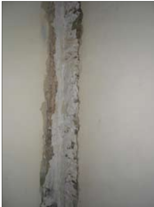
Figure 11.1 Join of two walls. Taken from the south east.
