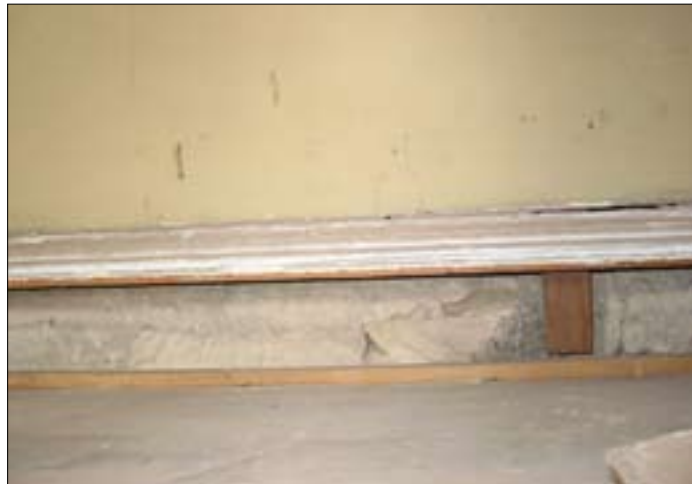
Figure 36.1 Wall surface. Taken from the east.
