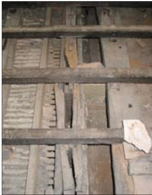
Figure 22.3 Timber partition wall slot. Taken from the east.
