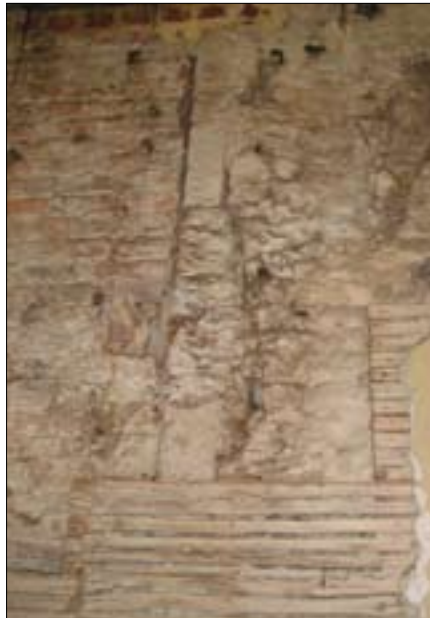
Figure 37.1 Window jamb. Taken from the north.
