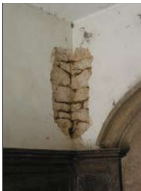
Figure 6.2 South-west corner of east porch.
