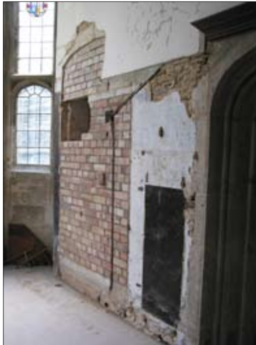
Figure 8.1 Blocked doorway and panelling effect. Taken from the north-west.
