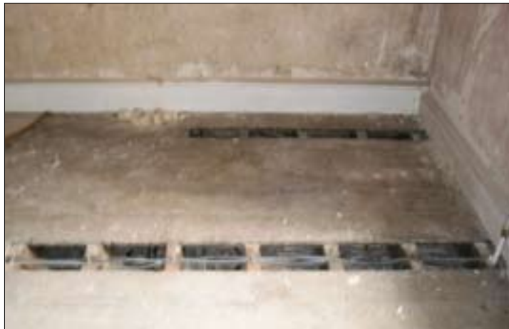
Figure 28.1 Floor structure. Taken from the south.
