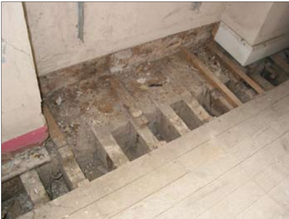
Figure 20.1 Floor structure. Taken from the south.
