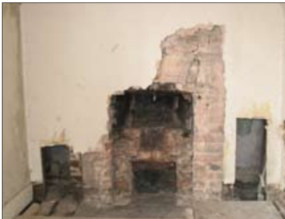
Figure 40.1 Fireplace. Taken from the east.
