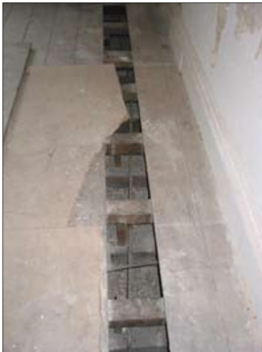
Figure 31.2 Showing levels of floor structure. Taken from the west.
