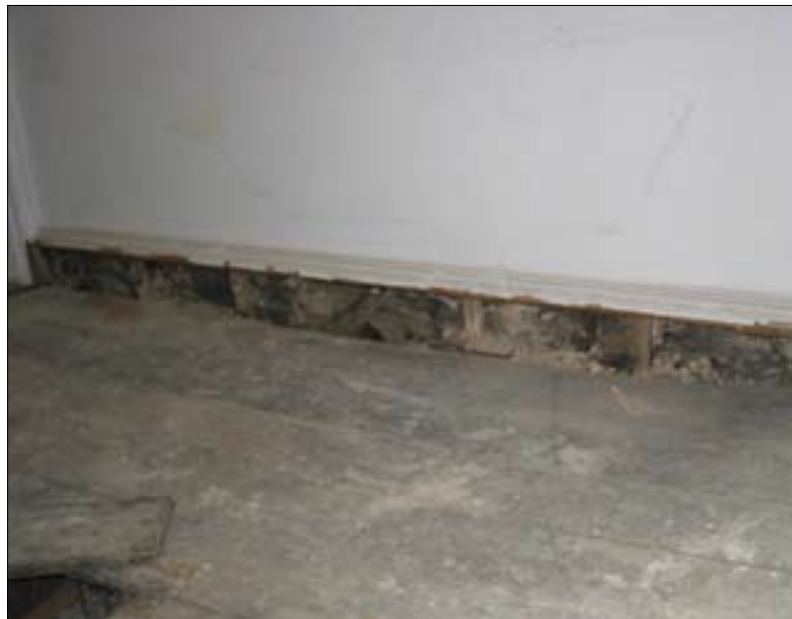
Figure 27.1 Coursed rubble walling. Taken from the east.
