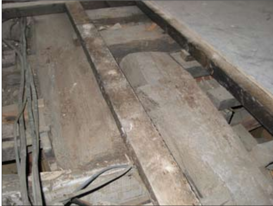
Figure 22.2 Overlapping main beams. Taken from the north.
