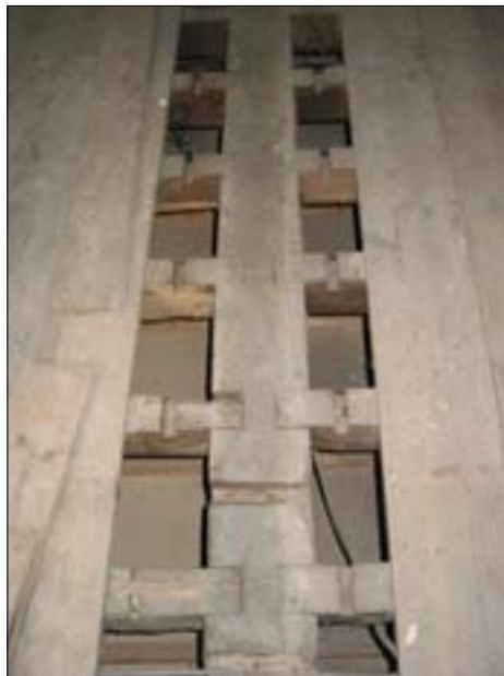
Figure 34.1 Floor structure in H2.11. Taken from south.
