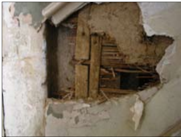
Figure 24.1 Stone door jamb behind lathe, reed and plaster wall.
