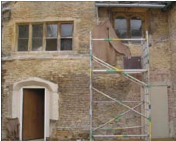
Figure 3.1 External wall from the west.
