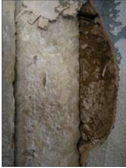
Figure 24.2 Detail taken from the west.
