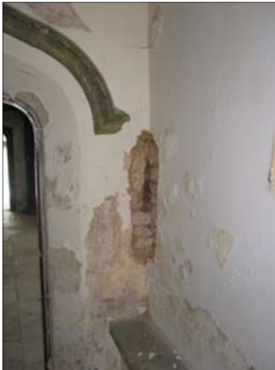
Figure 5.1 South-east corner of west porch.
