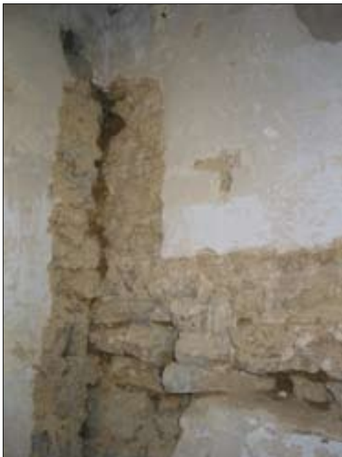
Figure 12.1 Join of two walls. Taken from the south west.
