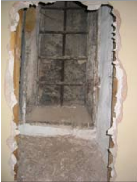
Figure 10.1 Blocked two-light stone mullion window. Taken from the north.
