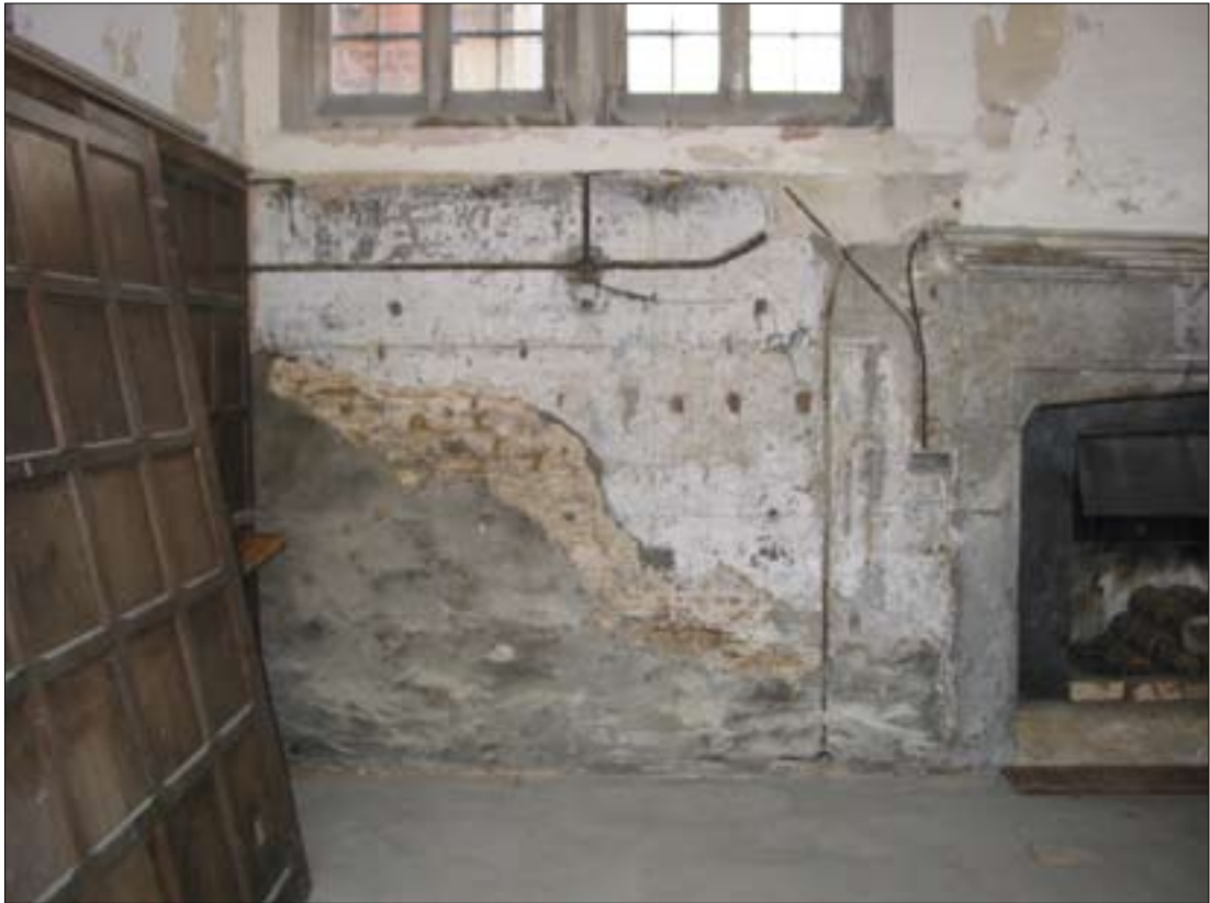
Figure 7.1 Wall and fixings. Taken from the east.
