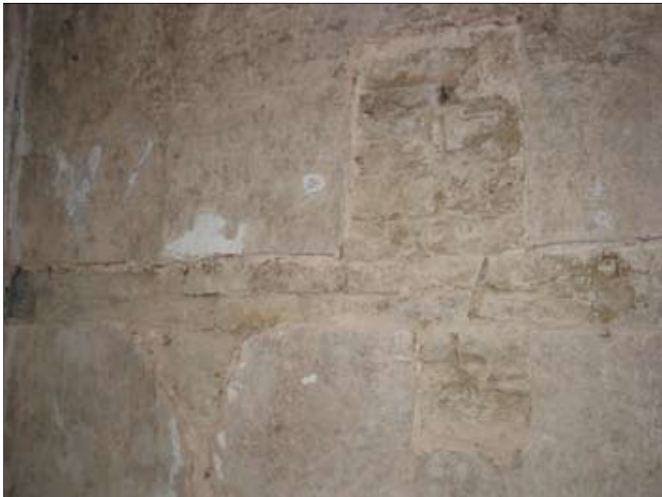
Figure 29.1 Coursed rubble walling. Taken from the south-west.
