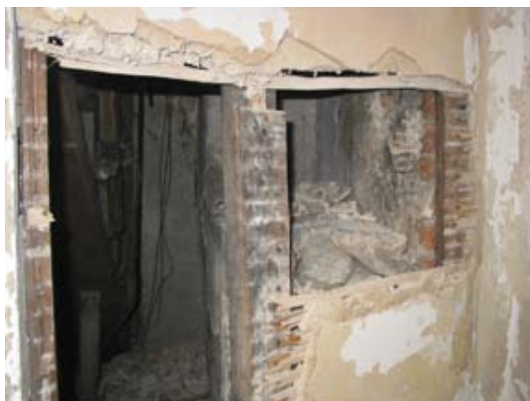
Figure 25.1 Wall with former cupboard behind. Taken from the south.
