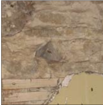
Figure 37.2 Void for wall fixing. Taken from the north.
