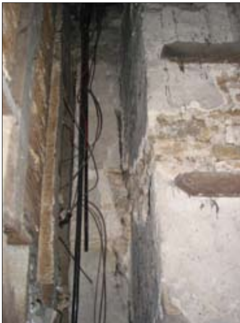
Figure 25.2 Showing the ashlar door jamb, the rubble constructed wall and wooden shelf brackets.
