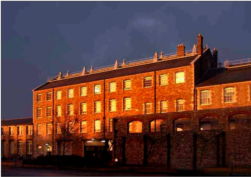
Figure 1: West elevation of the Engine House, Swindon.
