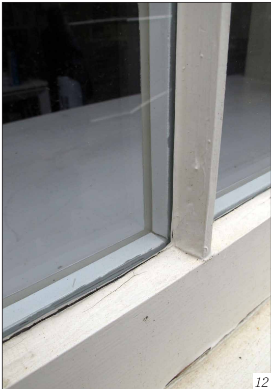
Figure 9: Reception Area windows after installation of double glazing system. Figure 10: Typical window pane before installation (interior view). Figure 11: Typical window pane after installation (interior view). Figure 12: Interior of the Reception Area window after installation.
