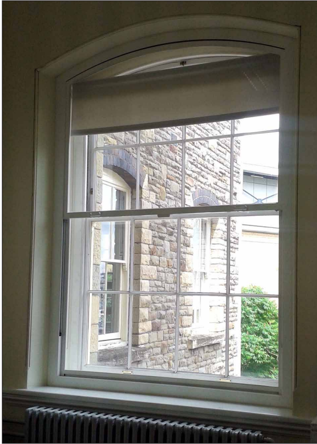
Figure 3: Typical secondary glazing installation in The Engine House.
