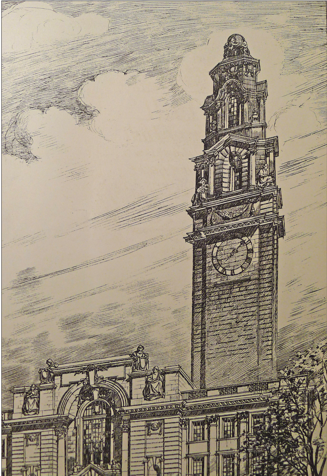
Fig. 14: Detail of the clock tower from the perspectival view of Cooper's competition-winning design, published in The Builder, 11 July 1903
