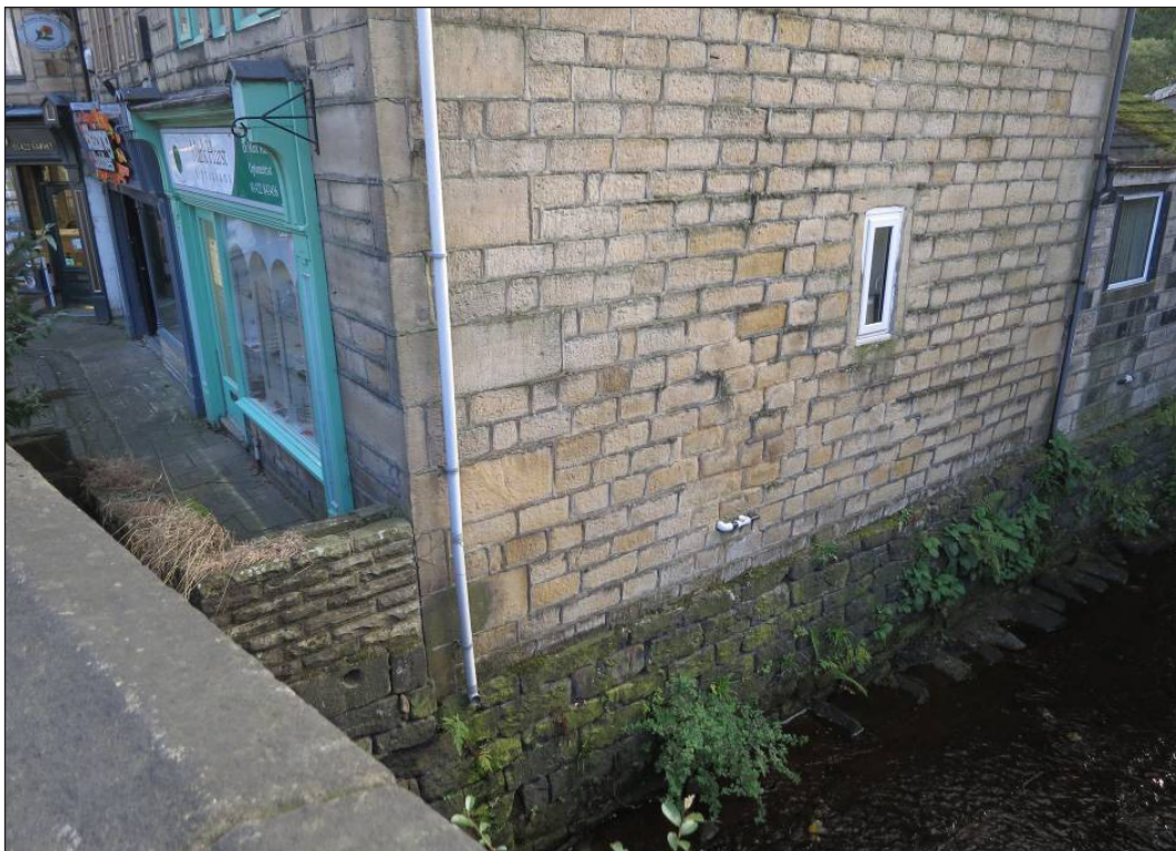
Figure 8: The shop is located on the banks of the river.
