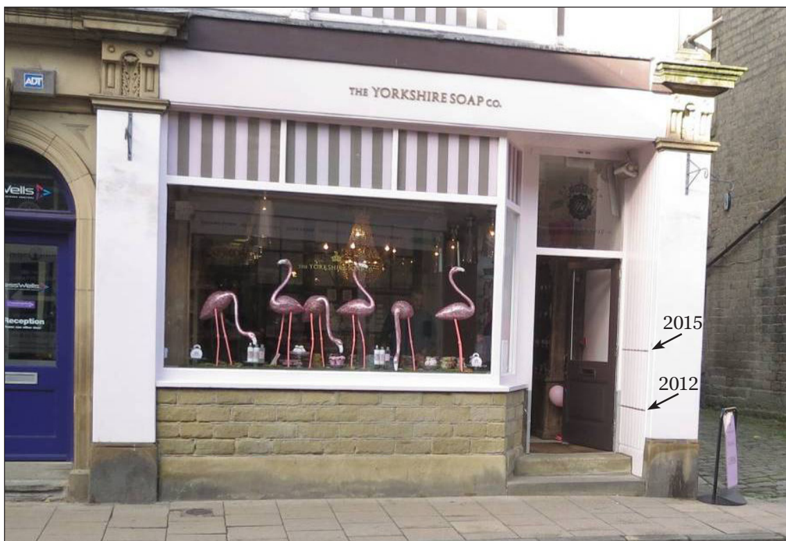
Figure 1: Shop front in Hebden Bridge showing levels reached by flood water in 2012 and 2015.
