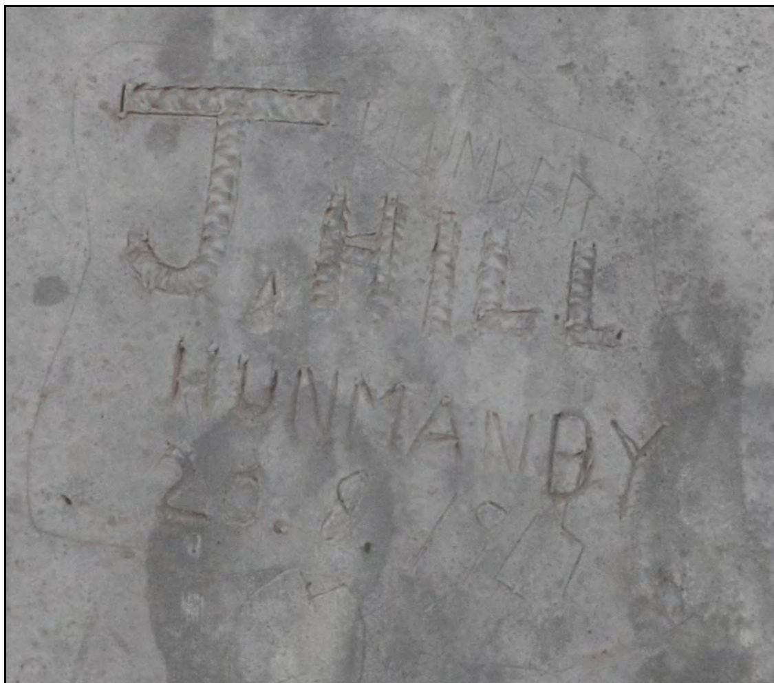
Figure 6. Panel W13 with J Hill, Plumber, Hunmanby 20.8.1947
