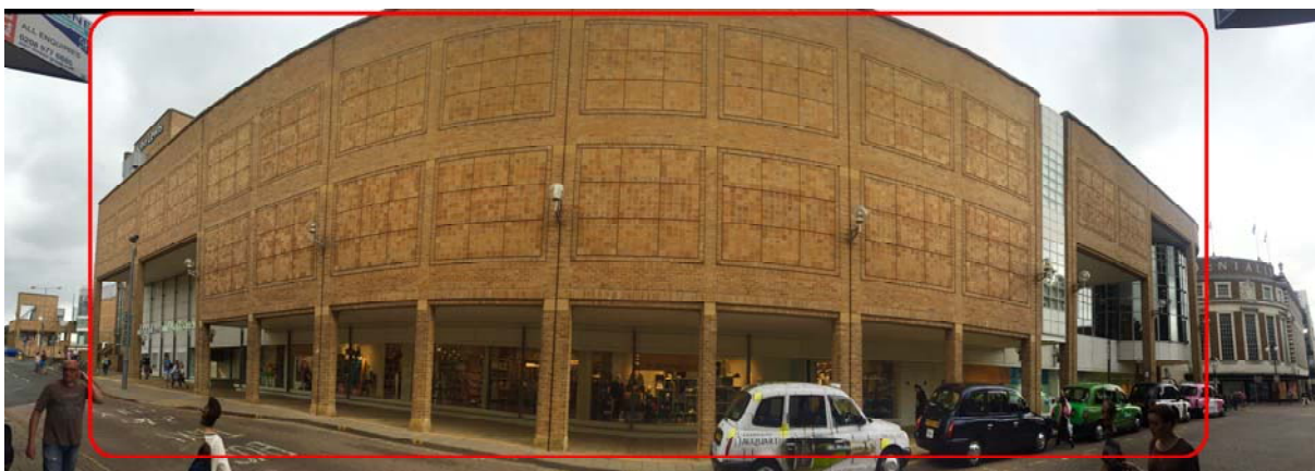
John Lewis: a significant building by Ahrends, Burton and Koralek (phases 1979-90); architecturally impressive and useful connection of Clarence Street over Horse Fair to the Thames
