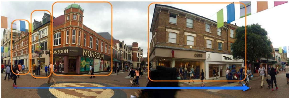
Nos 37-57: Materials and massing are largely consistent but the use of different brick across schemes creates a pleasing visual variety
