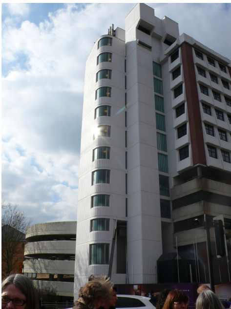
Fig.10 Combined House (Premier Inn and car park), Wheatfield Way (Owen Luder, 1975) © Historic England
