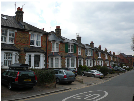
Fig. 17 Staggered semi-detached houses in The Bittoms
