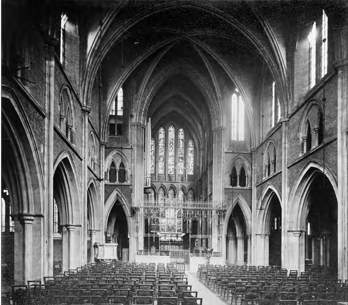
Figure 39: Interior of St John the Evangelist, Red Lion Square, London (3004_020 © Historic England Archive)
