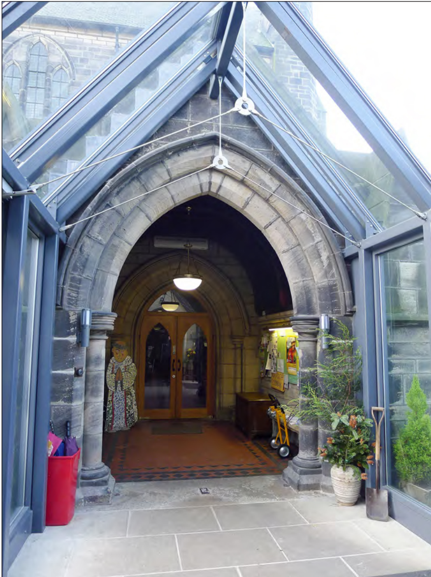
Figure 40: Glazed corridor linking church porch with the later parish centre at the Church of St Margaret, Horsforth (© Historic England, photograph: Clare Howard)
