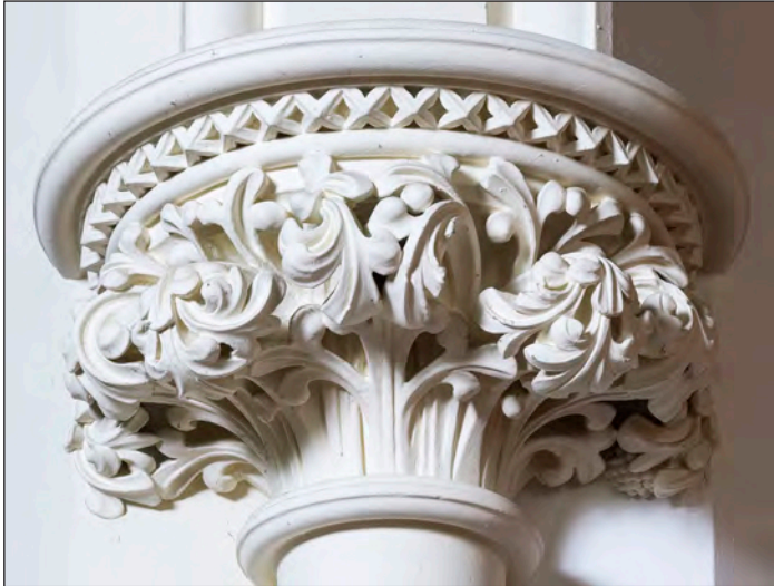
Figure 11: One of the foliate corbels carrying the chancel arch at the Church of St John and St Petroc, Devoran, Cornwall (DP172563 © Historic England, photograph: James O Davies)
