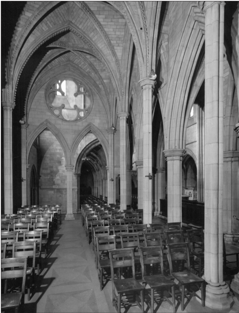
Figure 114: The south chapel of the Catholic Apostolic Church, Maida Avenue, taken from the south-east in 1967 (67/00907 © Historic England Archives)
