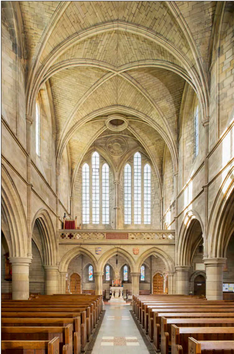
Figure 100: The nave, showing baptistery underneath gallery, at the Church of St George in Cullercoats, (DP168585 © Historic England, photograph: Alun Bull)
