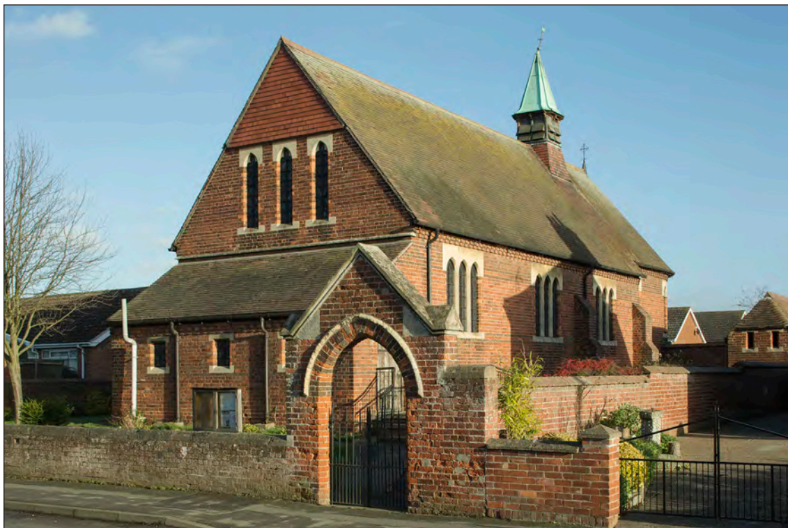
Figure 79: The Church of St Hugh, Sturton by Stow, taken from the south-west (D172344 © Historic England, photograph: Pat Payne)
