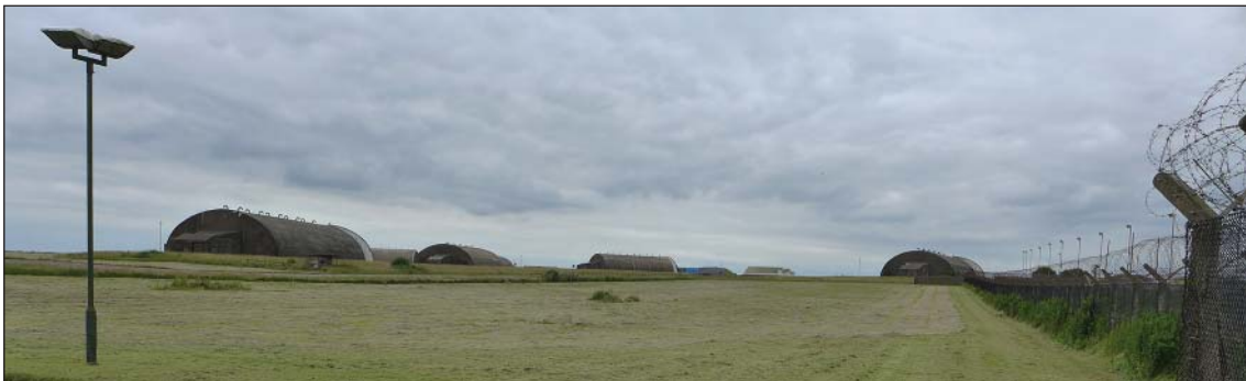
Figure 14: RAF Upper Heyford, the airfield landscape with Hardened Aircraft Shelters. (c) W D Cocroft
