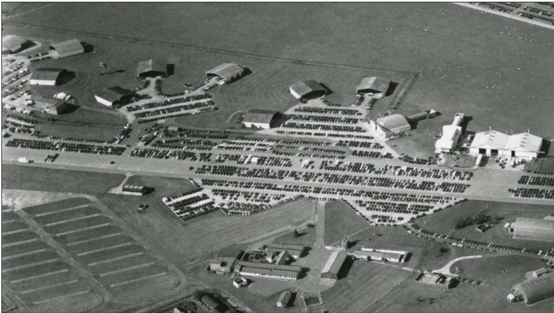
Figure 13: RAF Upper Heyford, early 1970s weather shelters to the right is a Hush House and engine test cell, to the bottom is the 79th squadron headquarters complex (c) Historic England 18537/13
