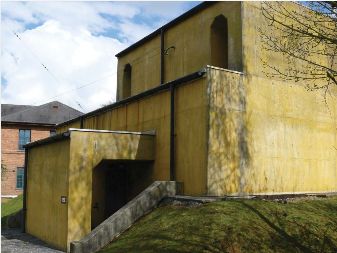
Figure 20: RAF Upper Heyford, 129 Telephone Exchange. (c) W D Cocroft
