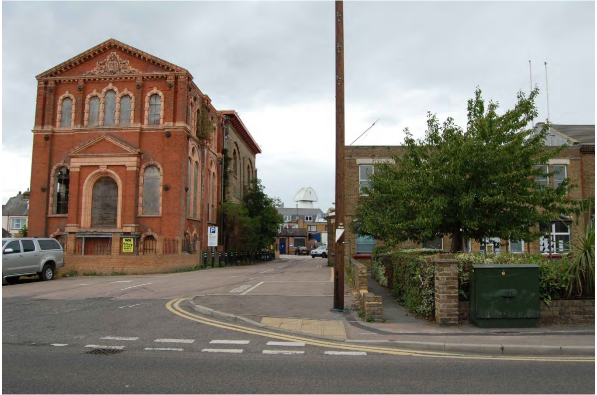
Photograph 35: HCA11 – unlisted pumping station and adjacent offices, fronting Trinity Road
