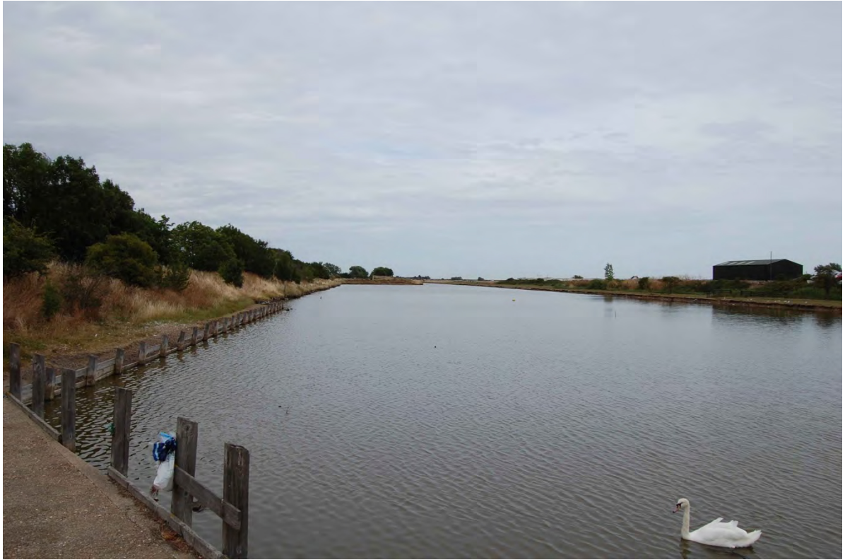
Photograph 12: HCA04 – wet section of Queenborough Lines, east of Halfway Road
