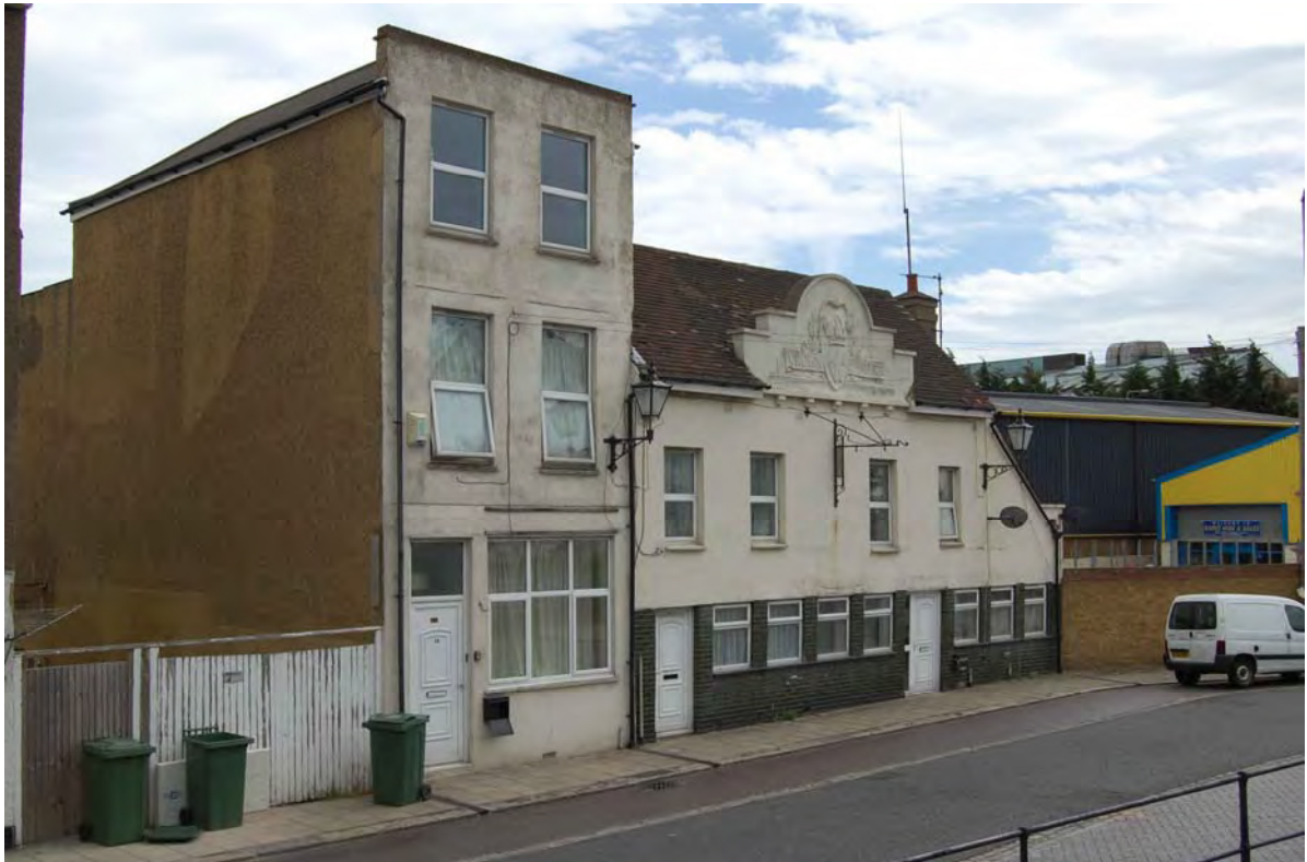
Photograph 23: HCA07 – the former Crown and Anchor on West Street, Blue Town
