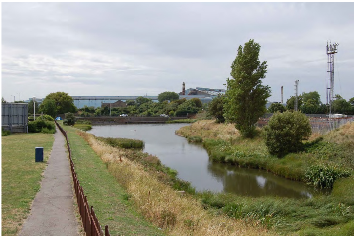
Photograph 8: HCA03 – northern section of Sheerness lines showing Bridge Road and supporting sub-structure
