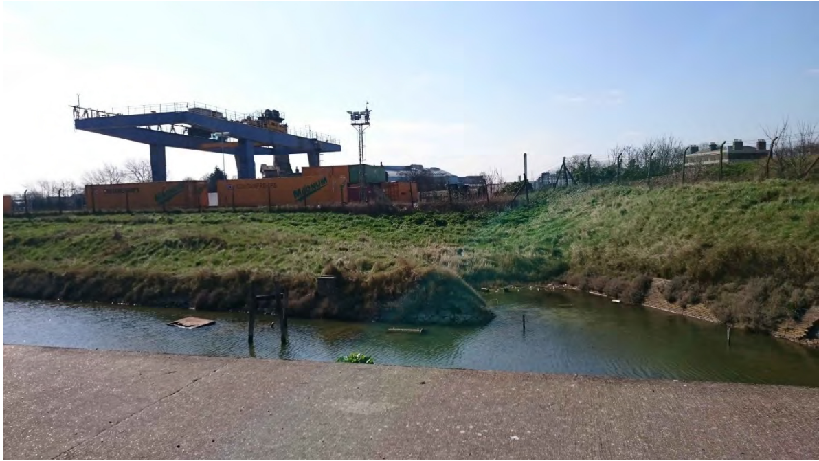
Photograph 1: HCA01 – junction of Indented Lines and Linking Trace
