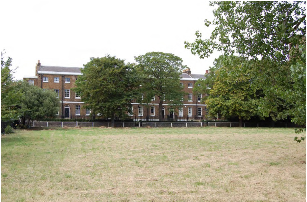
Photograph 6: HCA01 – Dockyard Terrace
