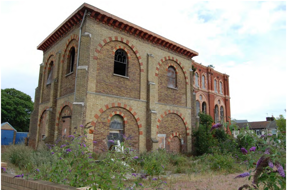
Photograph 36: HCA11 – rear of unlisted pumping station
