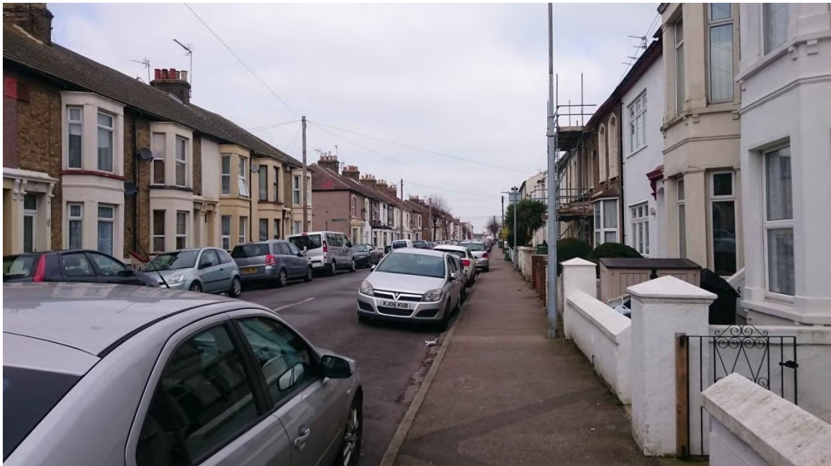
Photograph 43: HCA 14 – terraced housing along Invicta Road from the junction with Winstanley Road
