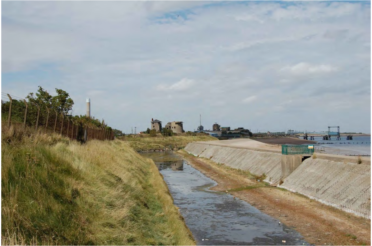
Photograph 3: HCA01 - Centre Bastion emplacements, Garrison Point Fort and defensive line at the northern port boundary
