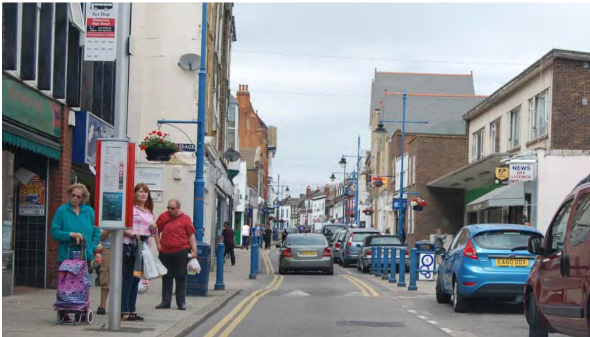
Photograph 34: HCA11 – south end of High Street, Mile Town, showing 1960s infill and historic street frontage
