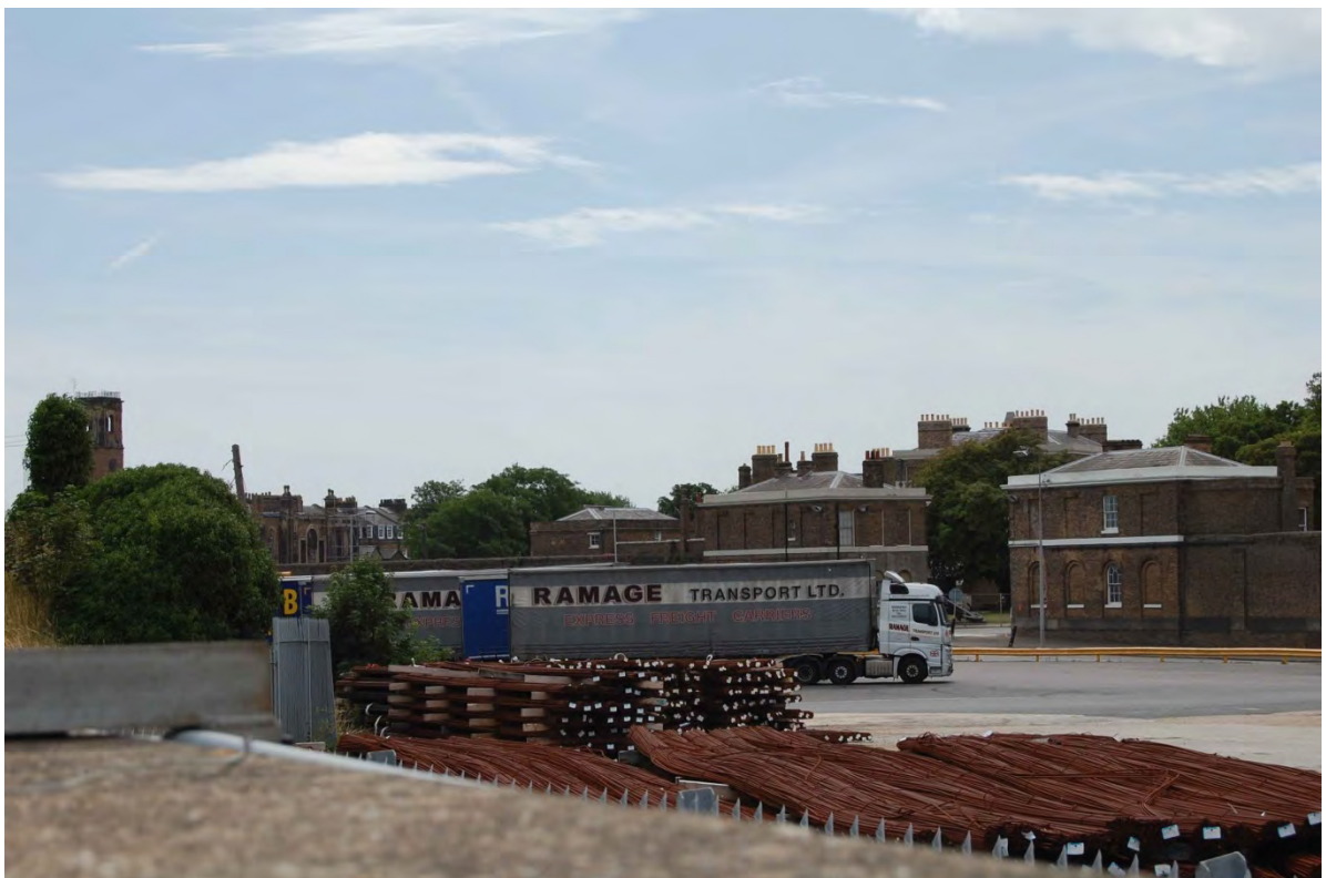
Photograph 4: HCA01 – port interior showing listed structures: (L-R) Dockyard Church, Dockyard Wall, North Gate House and South Gate House
