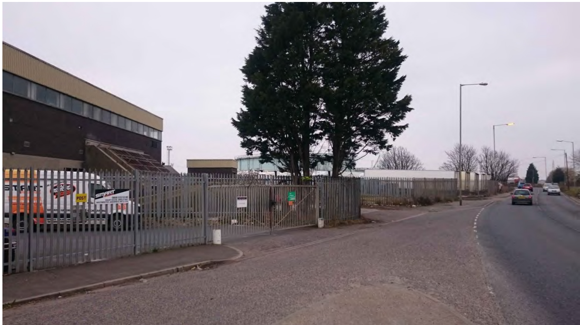
Photograph 49: HCA22 – pumping station and gas holders adjacent to Brielle Way
