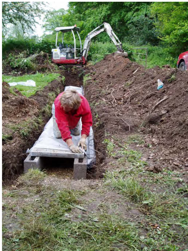
Figure 16: TAD installation working shot, Christ Church, Hatherden, Winchester diocese
