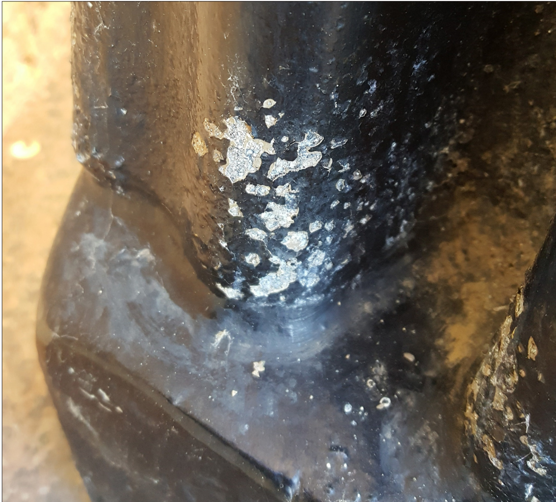
Fig 1: Osborne House statue (Urania) showing areas where the bronze-effect coating has deteriorated, exposing the underlying zinc metal.
